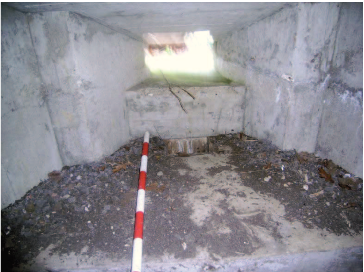
Plate 22: Internal view. NW facing loop in NW room
