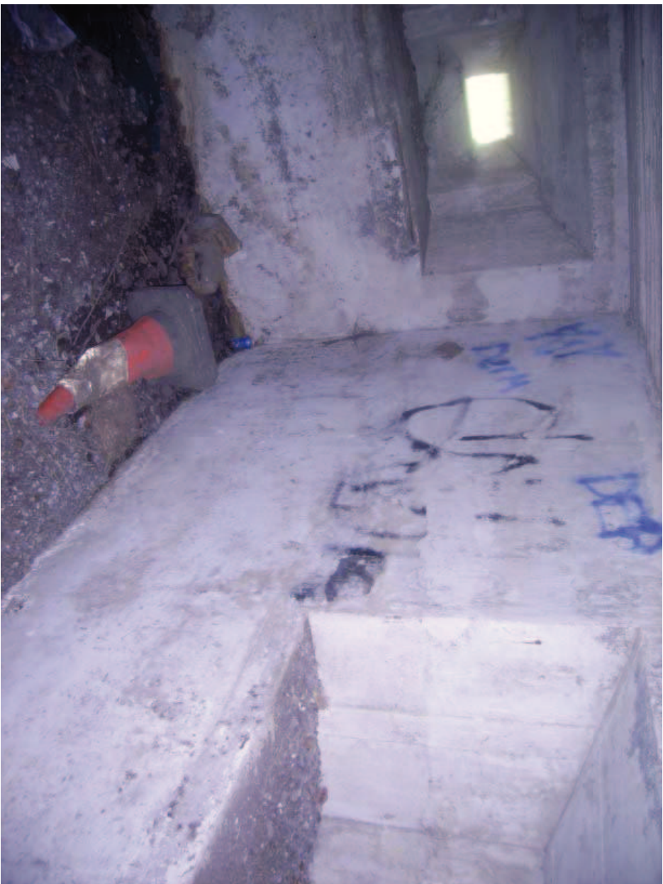
Plate 24: NW room looking west
