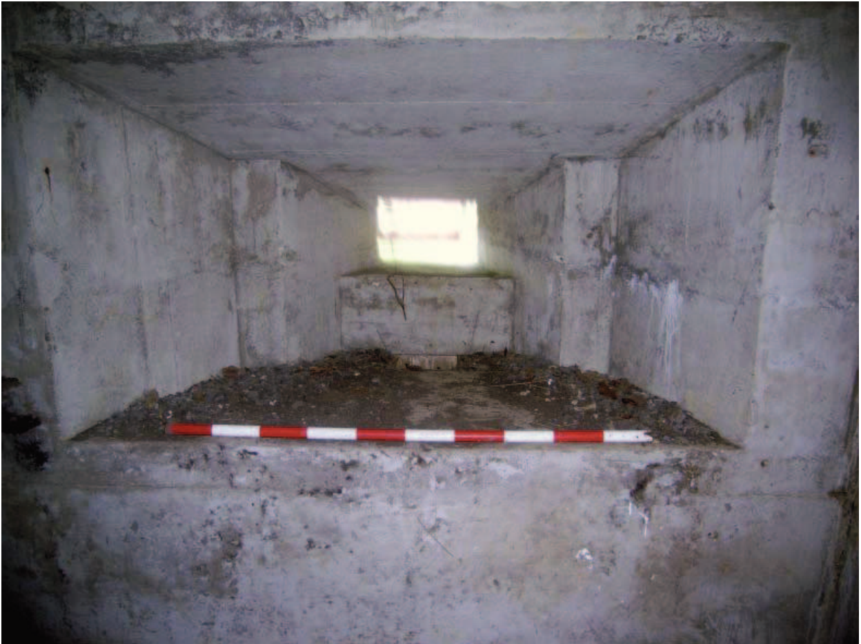
Plate 21: Internal view. NW facing loop in NW room
