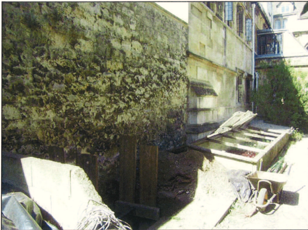
Plate 4: ATP3 General View
