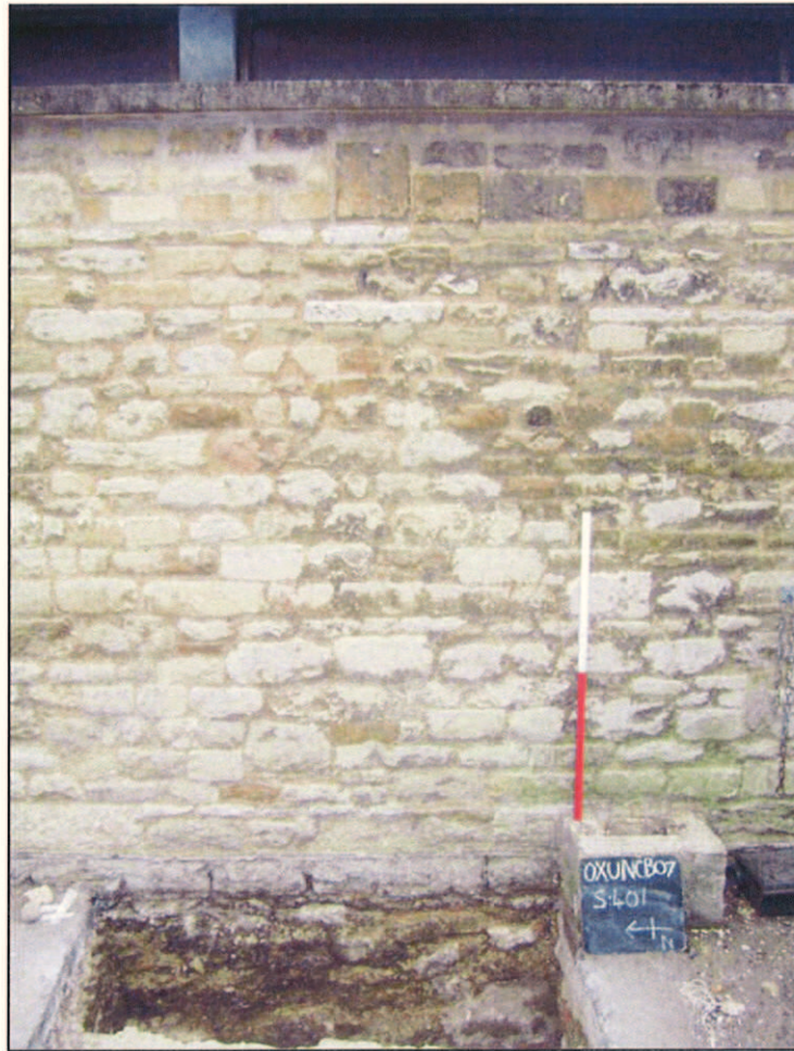
Plate 3: ATP4 - as excavated looking east
