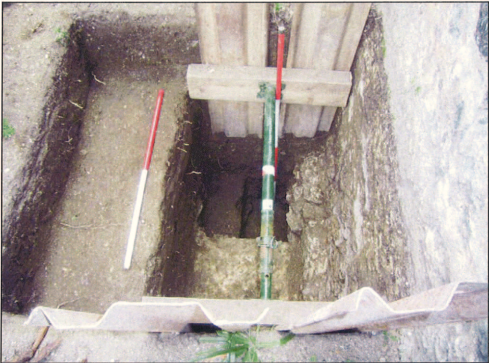
Plate 2: ATP3 - as excavated looking south
