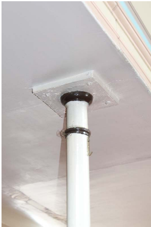
Plates 25 and 26: The capital of a cast iron column supporting the gallery above. The right hand image shows the ramped pews along the eastern gallery looking north
