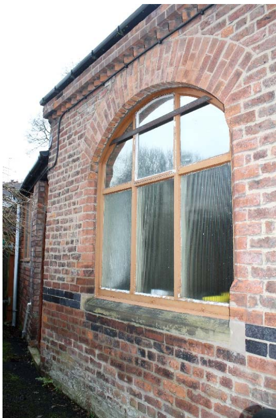
Plate 34: The southern window on the eastern elevation of school room, facing south-west. Note the dog tooth cornice and decorative use of engineering brick at sill height
