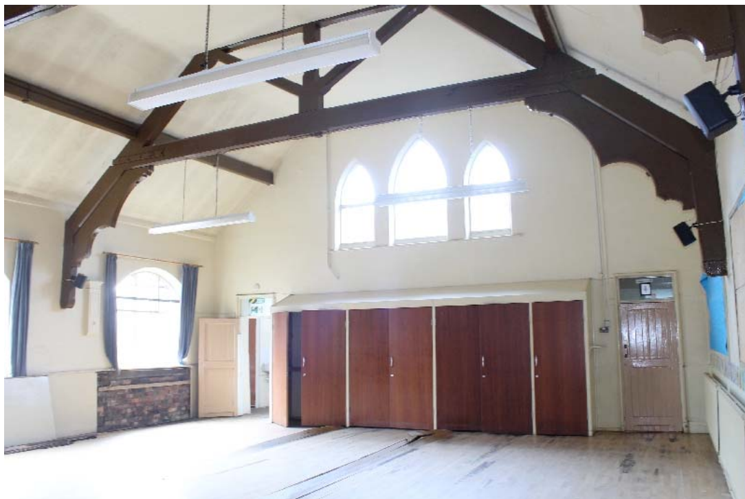
Plate 36: The interior of the school room, facing south; note the poor condition of the floor. The doorways at either end of the wall lead into the ancillary building
