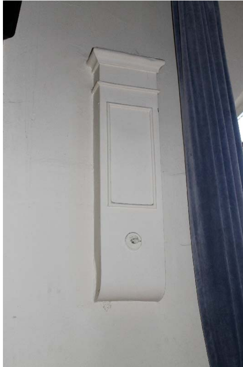
Plate 38: A vent on the eastern wall of the school room
