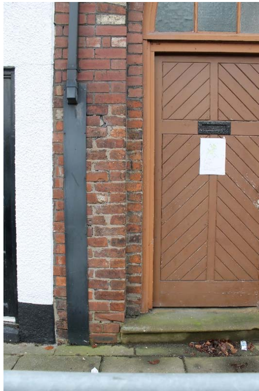
Plate 41: The variable character of brick work on the eastern jamb of the doorway on the northern elevation
