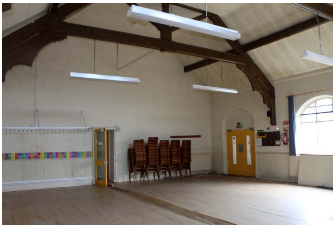
Plate 37: The interior of school room, facing north-east. The timber boarding of the northern wall can just be seen to the left of the doorway and behind the chairs
