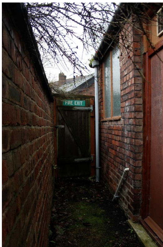
Plate 50: The eastern elevation of the ancillary building, facing south along a narrow yard
