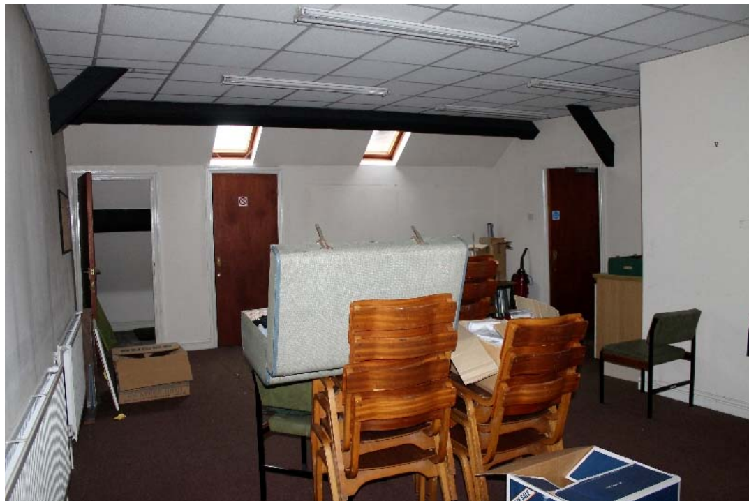
Plate 48: The first-floor of the Sunday school, facing south. Note the feet of the earlier 'A' frame truss just visible beneath the artificial ceiling
