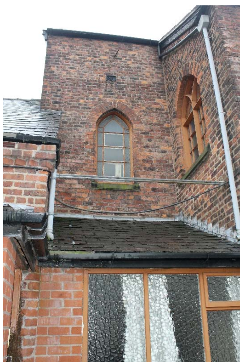
Plates 17 and 18: The first floor window on the eastern elevation of the square cell at the southern end of the chapel. The window to the right lights the gallery of the chapel. The photograph to the right shows the modern vestry extension
