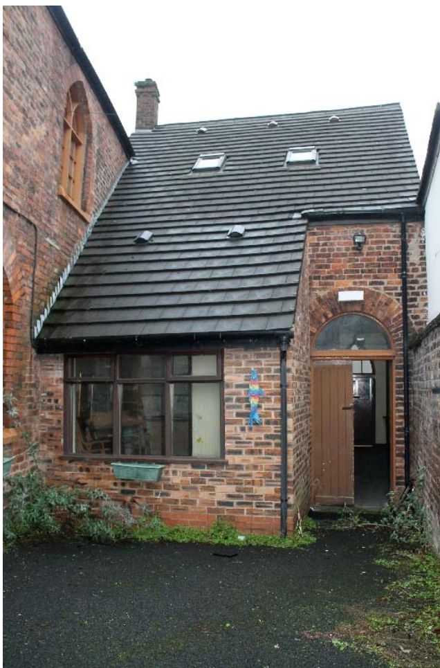
Plate 43: The southern elevation of the Sunday school with a modern extension lying beneath the cat slide roof. The original doorway with semicircular headed arch lies to the right of frame
