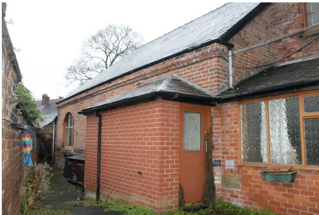
Plate 35: The modern porch extension with school room behind, facing south-west
