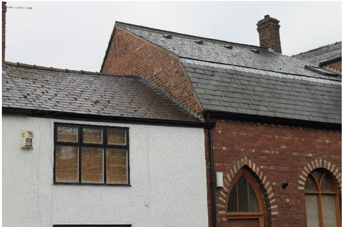
Plate 42: The eastern gable of the Sunday school visible above the roof of the attached cottage. A change in the character of the brickwork demonstrates that alterations have been carried out. Note the chimney stack on the opposing gable end
