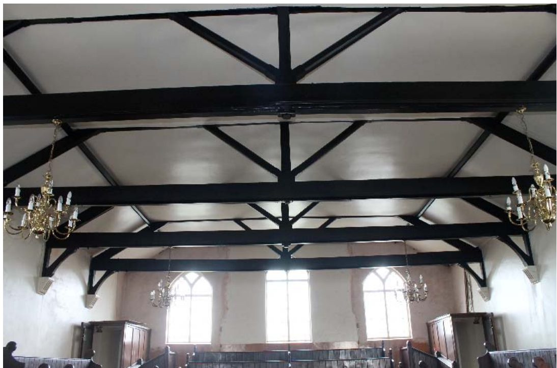
Plate 29: The king-post roof in the chapel, facing north
