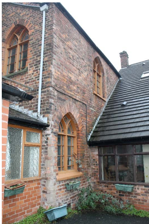
Plates 15 and 16: Eastern elevation of chapel, with Sunday school to the right of frame. The probable construction joint to the right of the window is visible in the photo to right; the joint coincides with a slight change in the character of the brickwork
