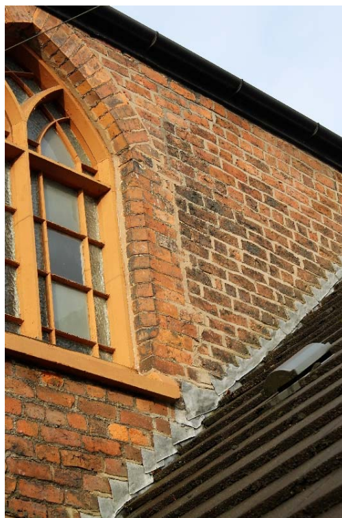
Plates 15 and 16: Eastern elevation of chapel, with Sunday school to the right of frame. The probable construction joint to the right of the window is visible in the photo to right; the joint coincides with a slight change in the character of the brickwork
