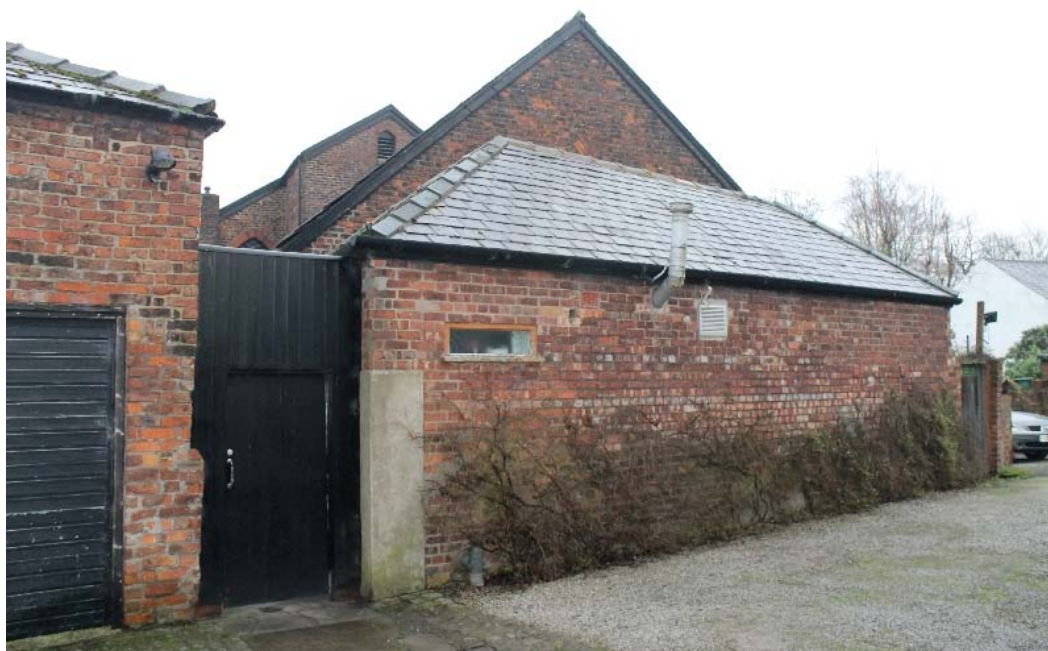
Plate 49: The southern elevation of the ancillary building, facing north-east
