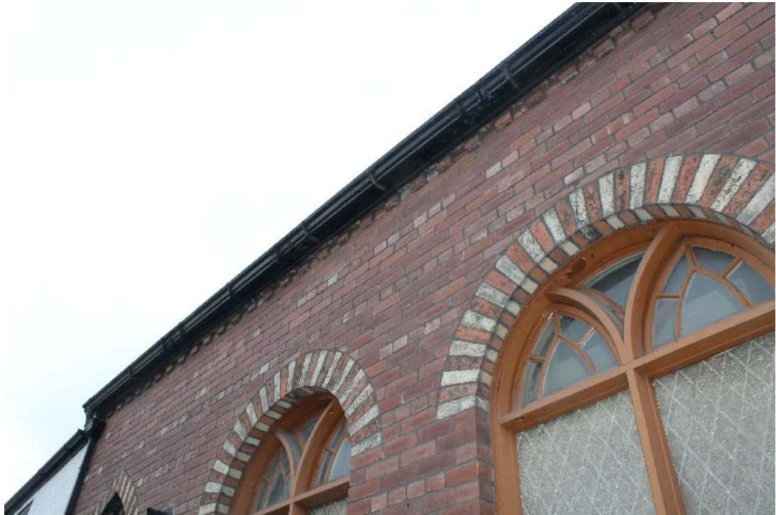
Plate 40: Polychrome window arches on the northern elevation, with dentil cornice visible at the head of the wall
