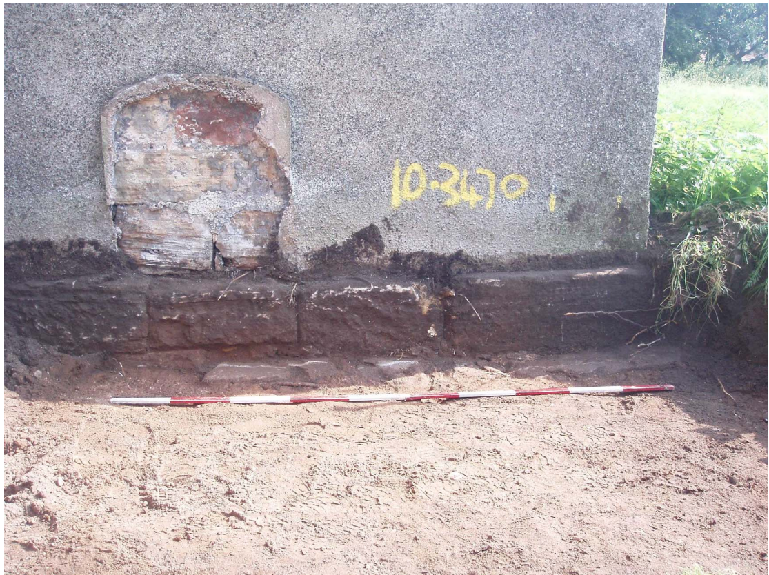
Plate 8: Trench 2, wall foundations, 105 , of St Mary's church, looking east
