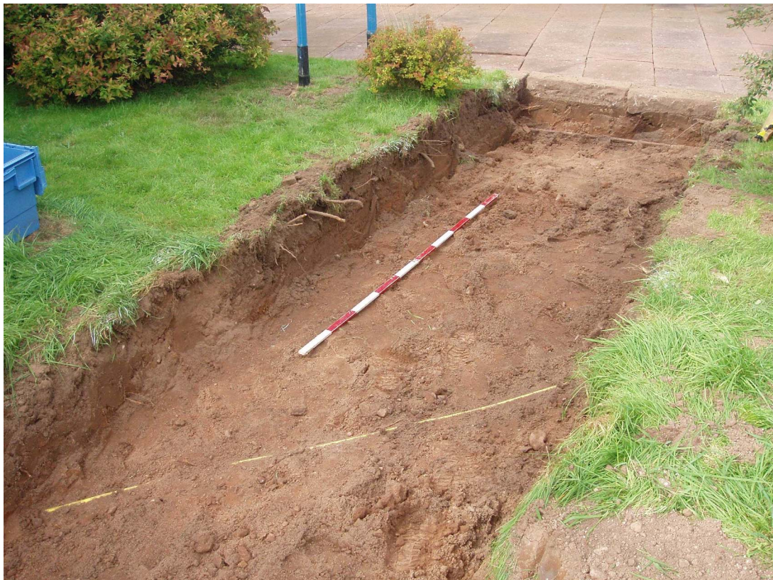
Plate 4: Trench 1, north end, showing two modern services and subsoil 101 , looking north
