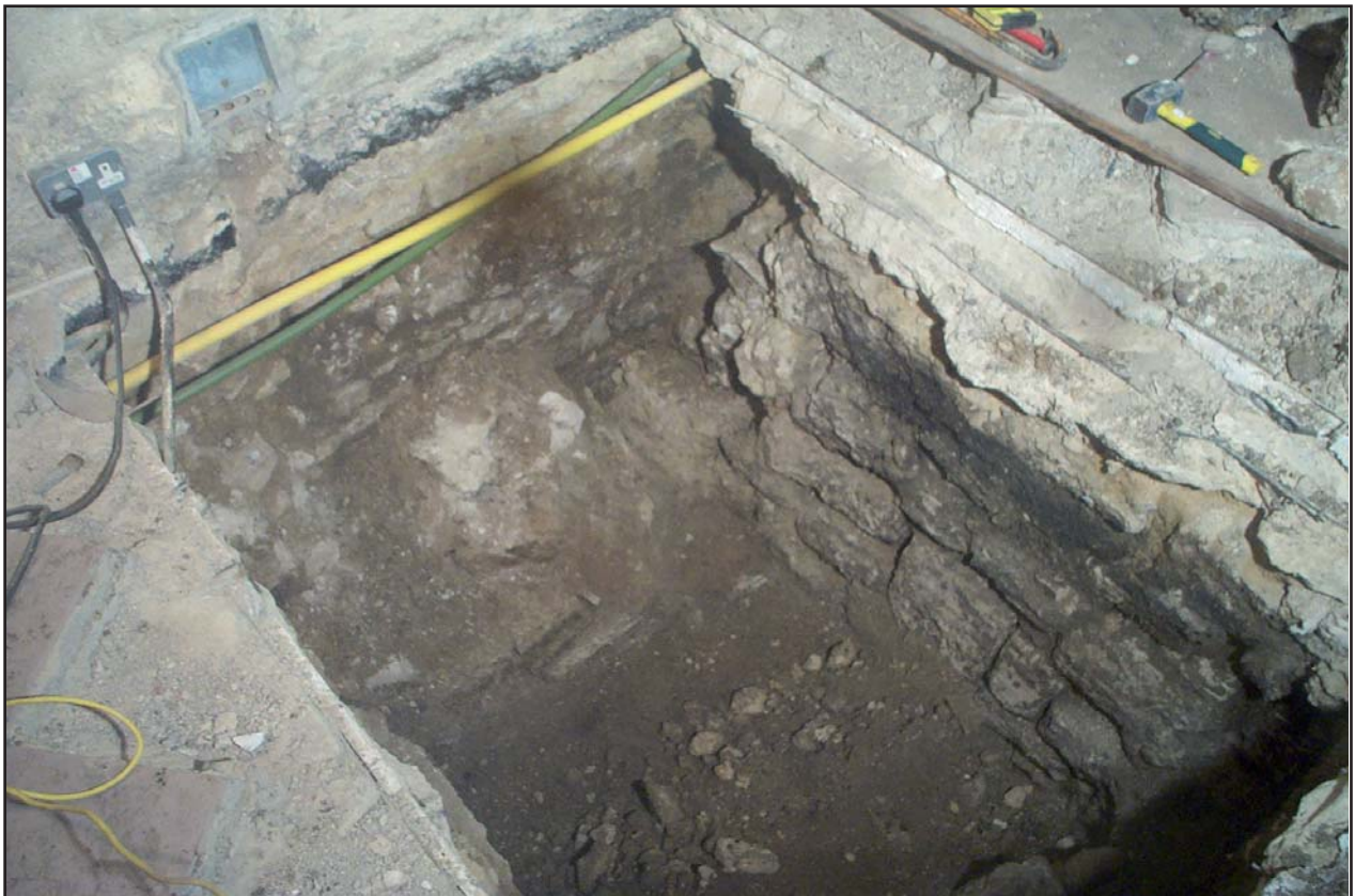
Plate 6: Trench 3 Footing 313 following partial dismantling of wall 305
