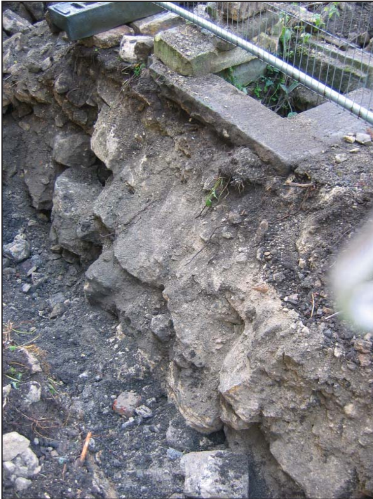
Plate 10: The west side of Trench 1b, showing the water tank's robbed (?) east side and the pennant framed manhole, 133
