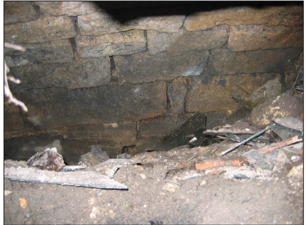
Plate 11: Interior of the water tank next to Trench 1b seen through a void in the side wall, showing it almost full of rubble and rubbish
