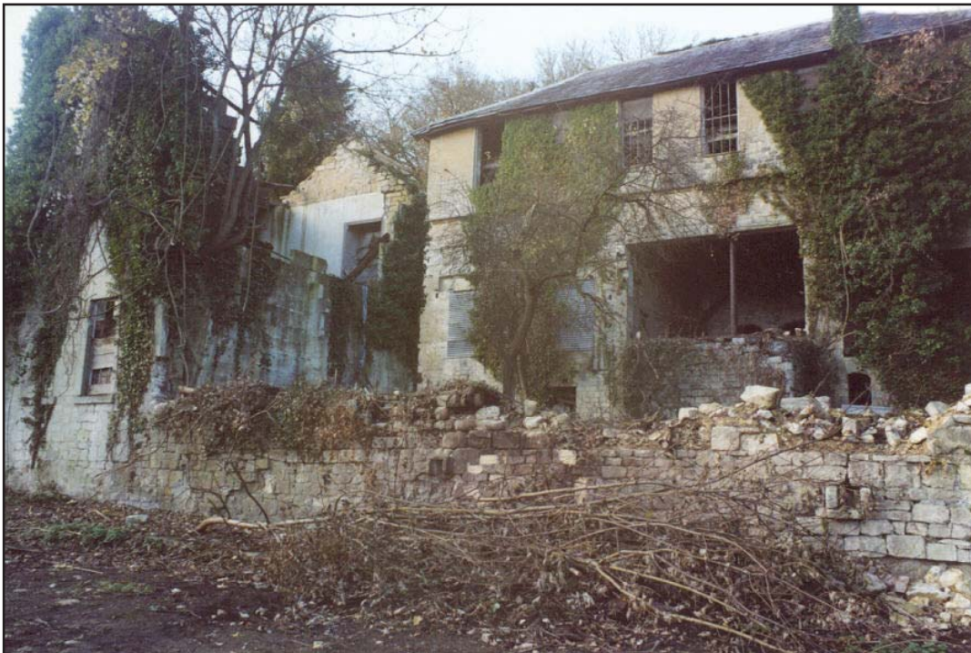
Plate 2: View from south with the platform of Building 3 in foreground (Building 4 to left) and Building 2 in the background
