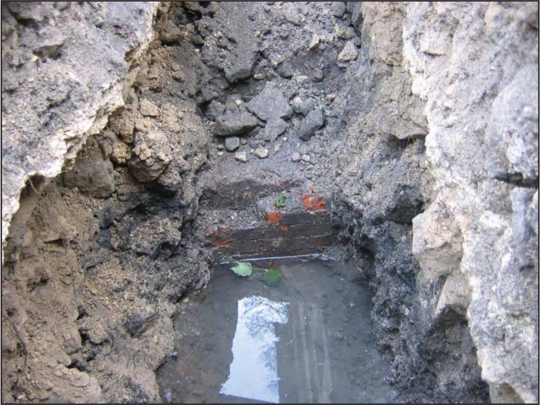
Plate 8: The brick culvert in Trench 1a seen from the south, just after discovery. Note the strong ledge formed by layer 129, the mortar layer between rubble fills 127 and 128
