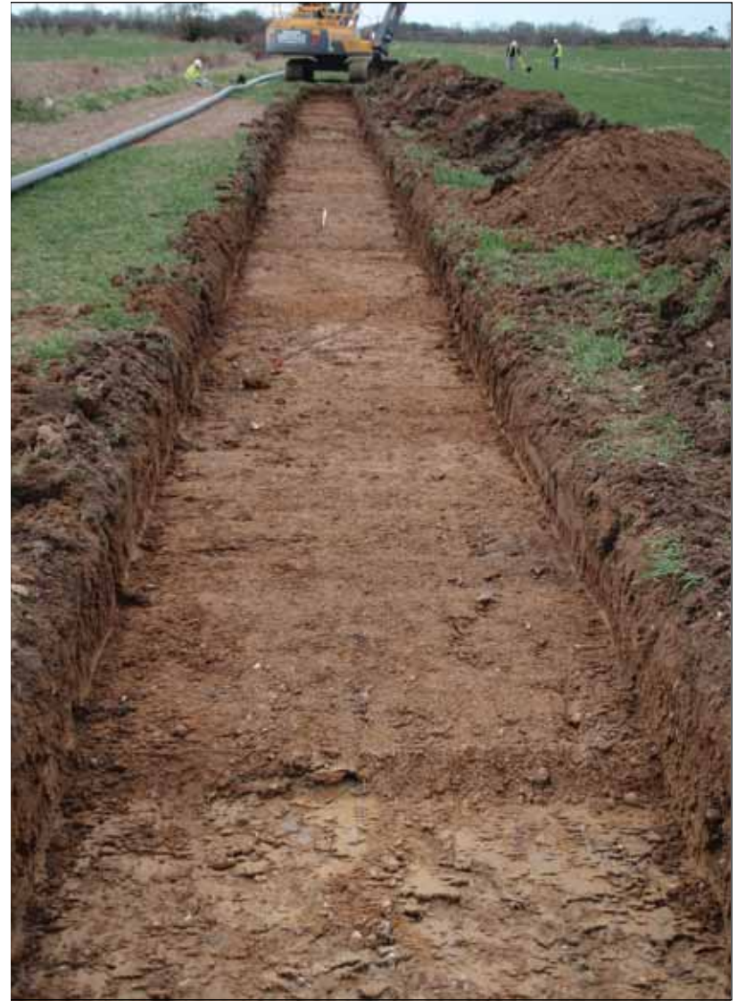
Plate 2 General view of trench looking south-west
