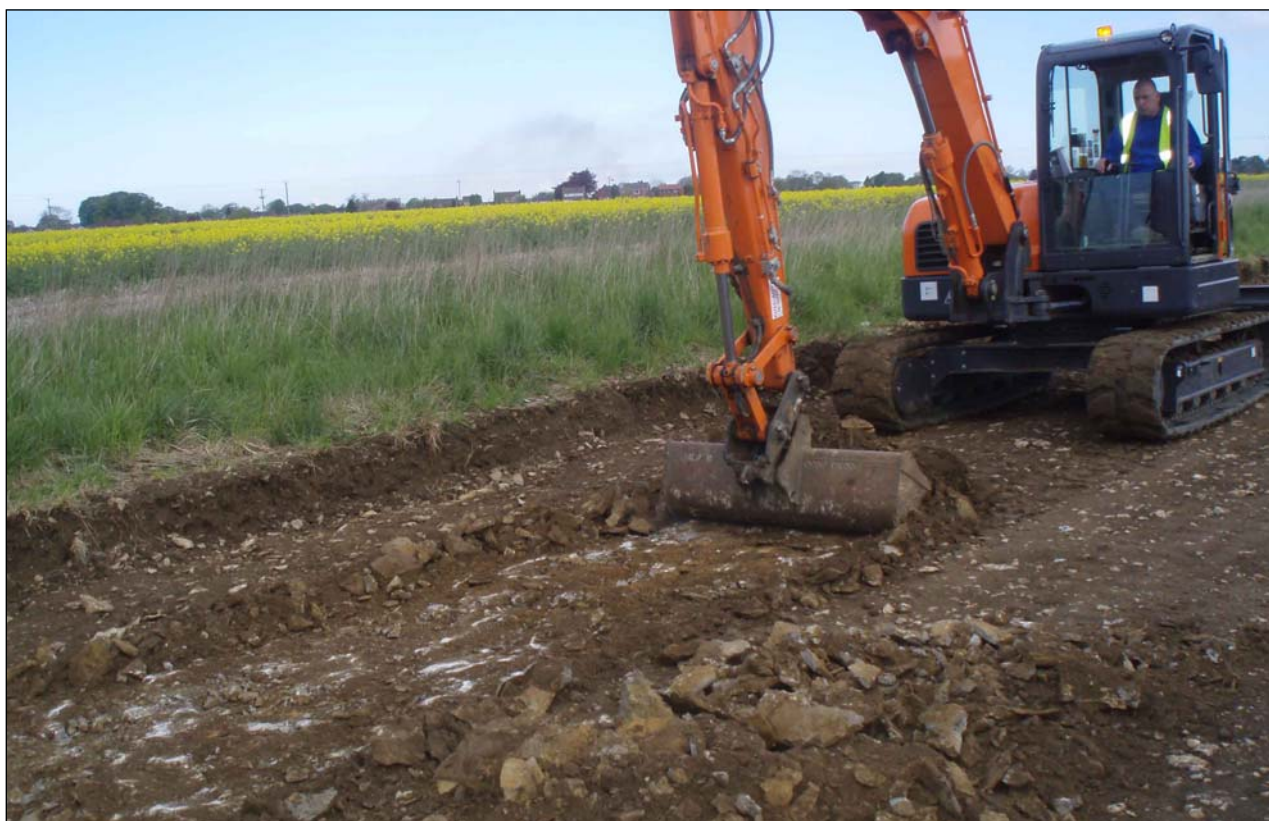
Plate 1: Excavation of pipe trench in field 1.
