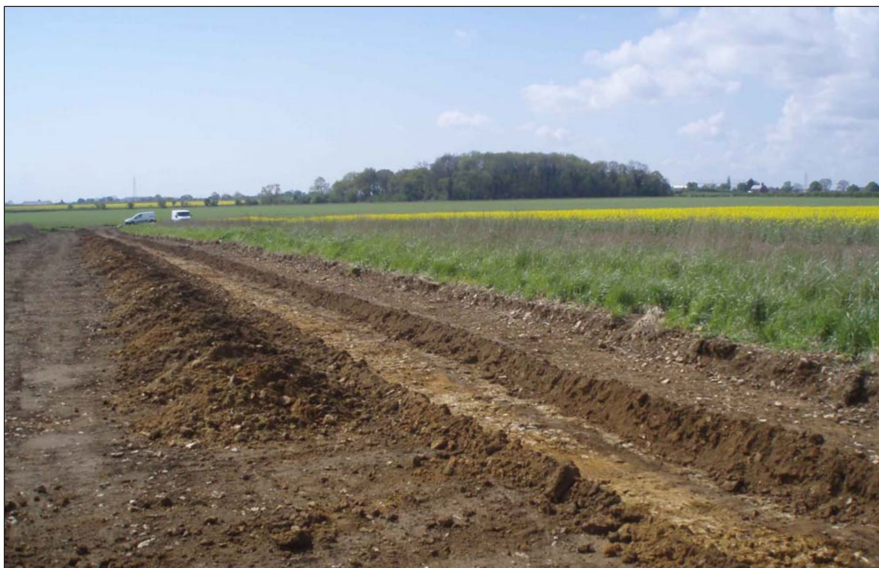
Plate 2: View of field 1 pipe trench from the north-east, showing modern boundary ditch in plan.
