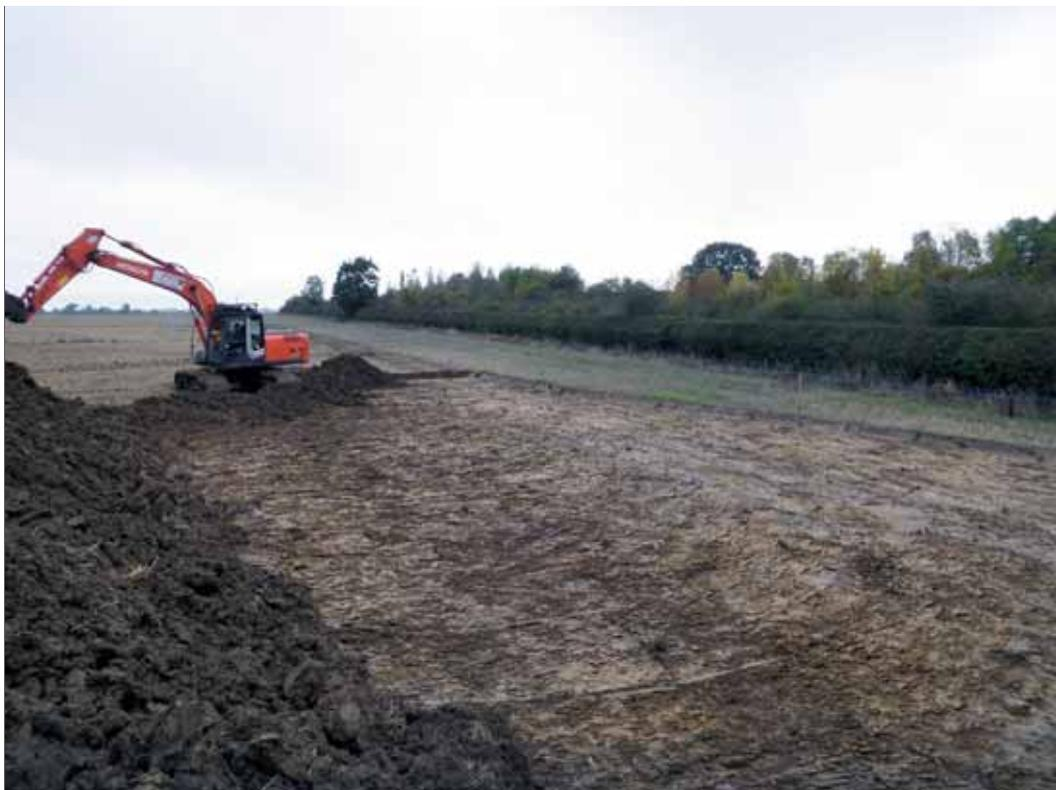
Plate 6: Topsoil stripping in watching brief area.
