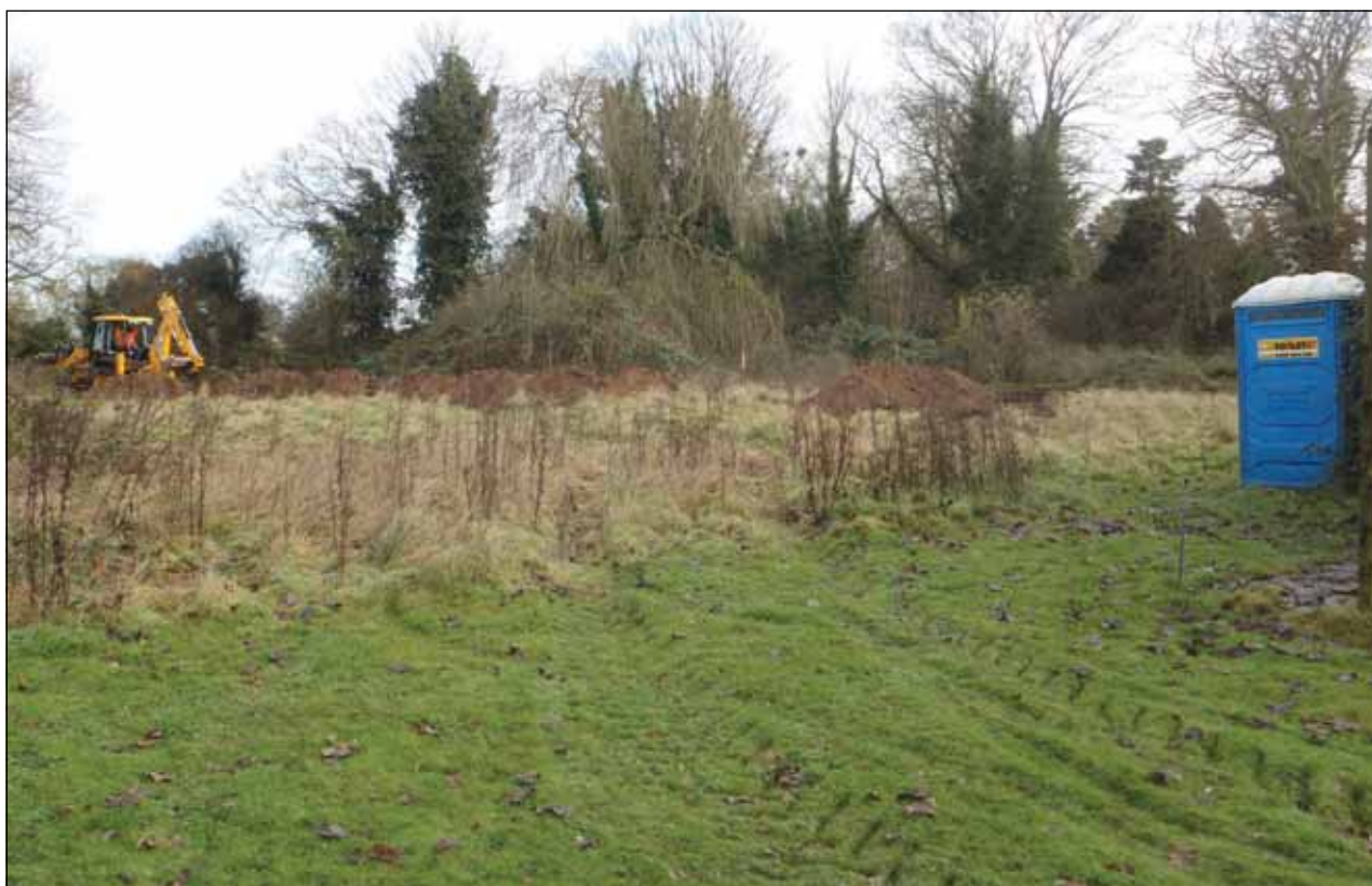
Plate 1: Working shot of site looking south east to trenches 1 and 2
