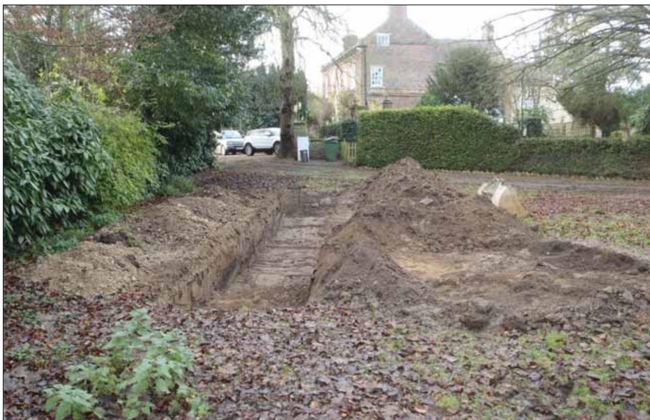
Plate 2: Working shot of site looking west to trench 4 and Lancewood house
