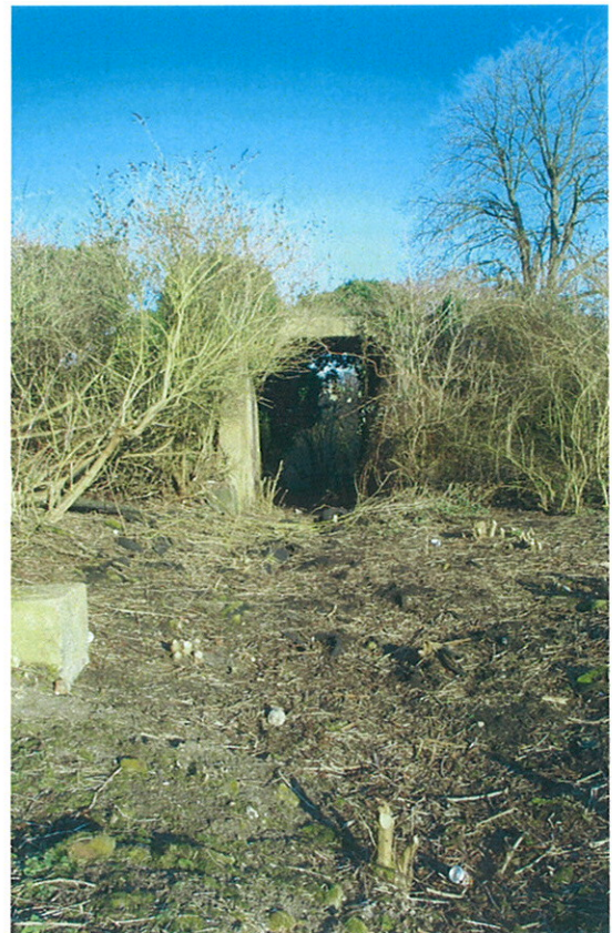
Plate 19: East view showing earthworks of internal rail track
