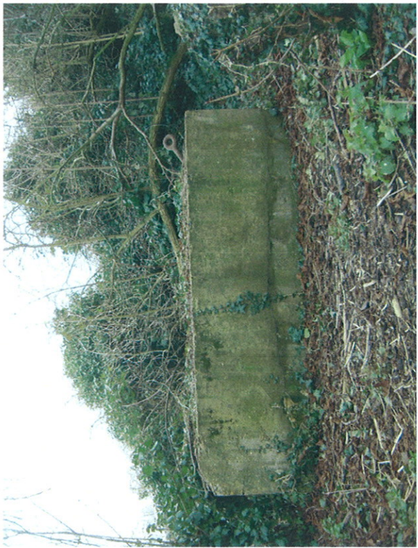
Plate 11: East view detailing iron hook extending from type 2 block, west embankment
