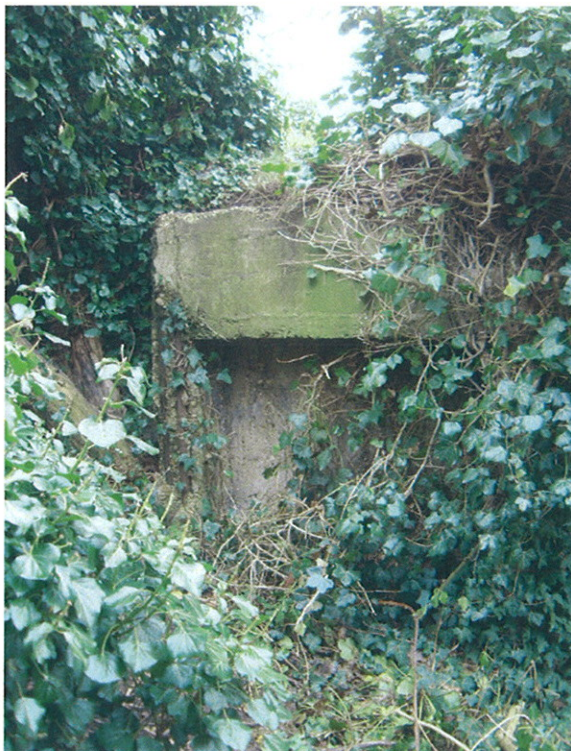
Plate 18: South view of tunnel 2 showing reinforced concrete side supports
