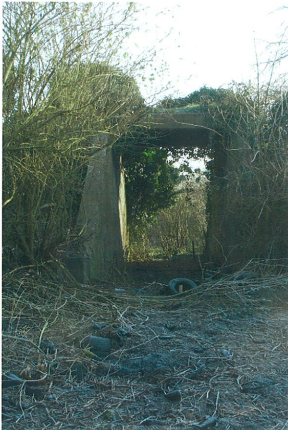
Plate 17: East view of tunnel 2
