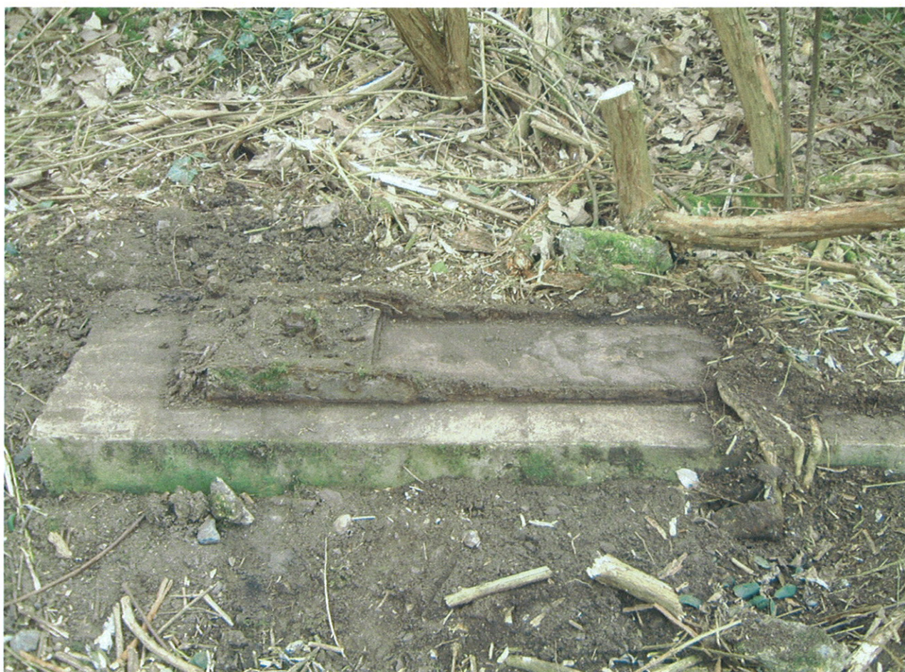
Plate 23: West view of internal concrete and iron platform
