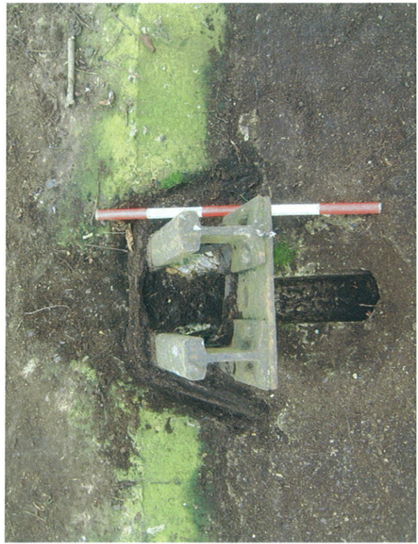
Plate 7: North view detailing iron bar extending from type 1 block, south embankment
