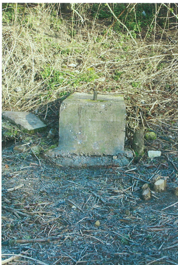
Plate 21: North view of internal concrete block
