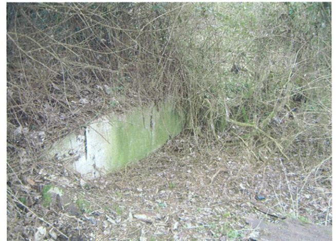
Plate 20: North west view showing internal railway buffer
