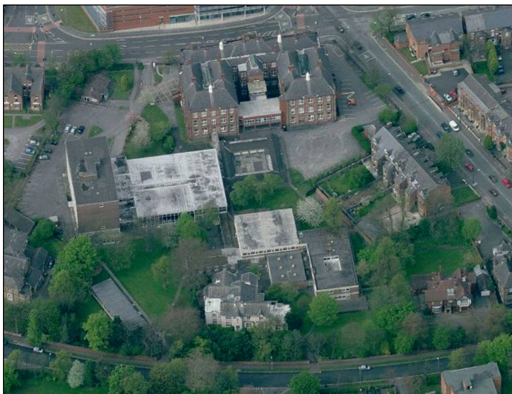
Plate 1: Ariel view across the study area, looking north. The excavation area lay to the left of the main collage building across the access road and lawn
