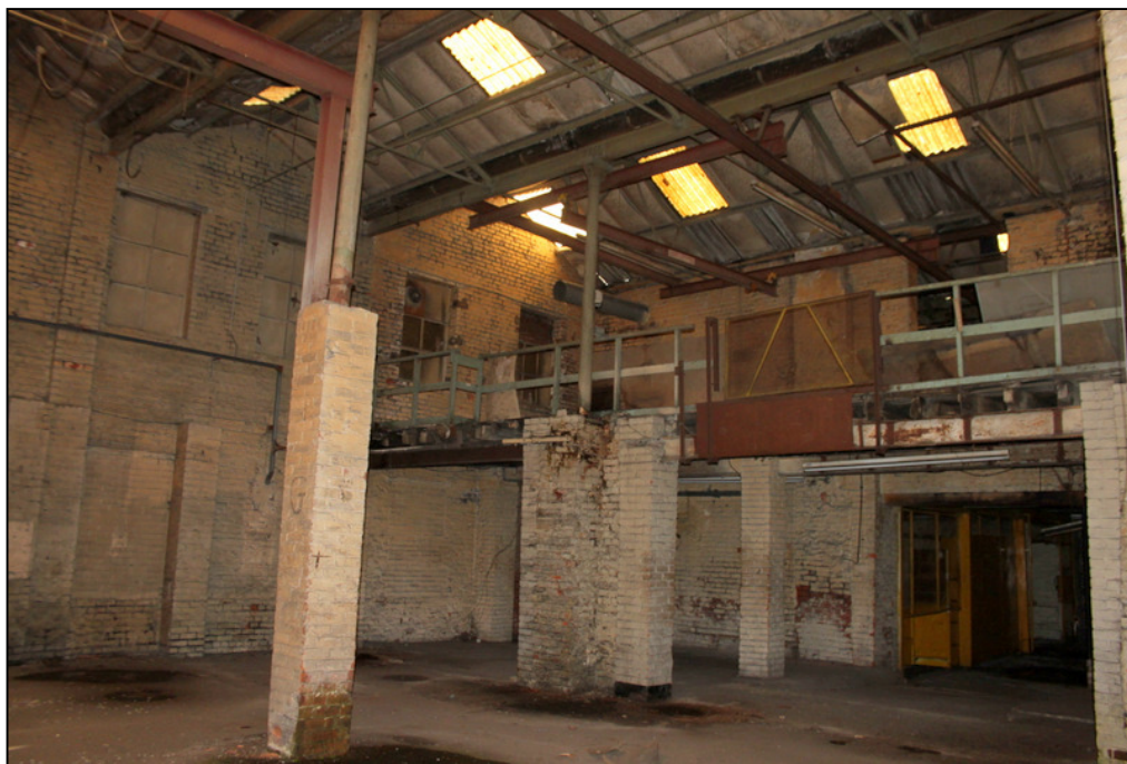
Plate 17: Internal view of Building B, from east bay, looking south-west
