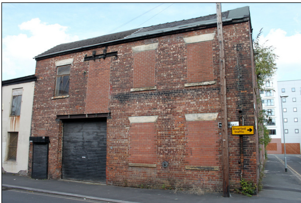
Plate 13: Western elevation of Building B, fronting Murray Street
