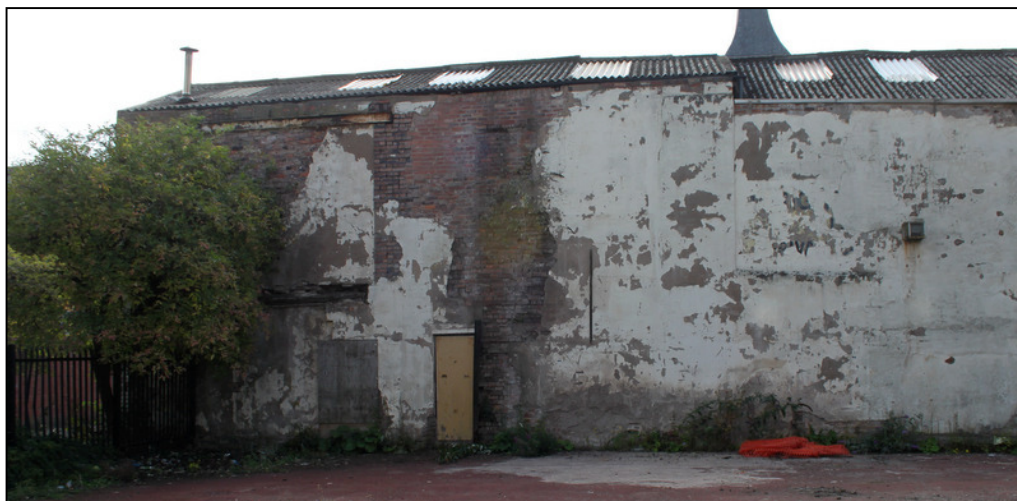
Plate 15: East elevation of Building B, with Building C on right
