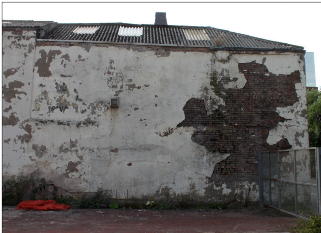
Plate 25: East external wall of Building C
