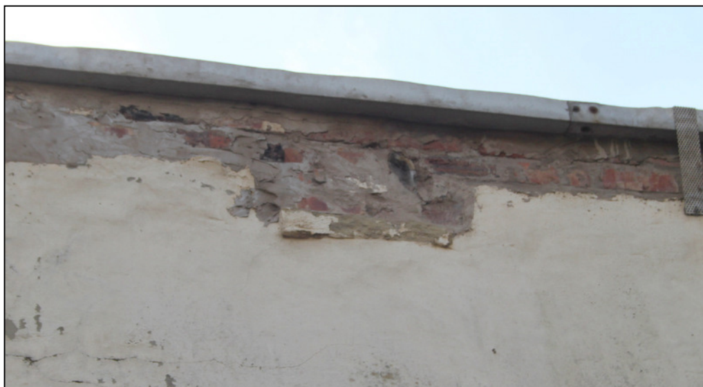
Plate 26: Sandstone pad in external east wall of Building C
