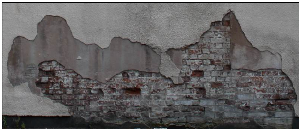
Plate 6: Flemish bond brickwork exposed beneath render in façade of Building A
