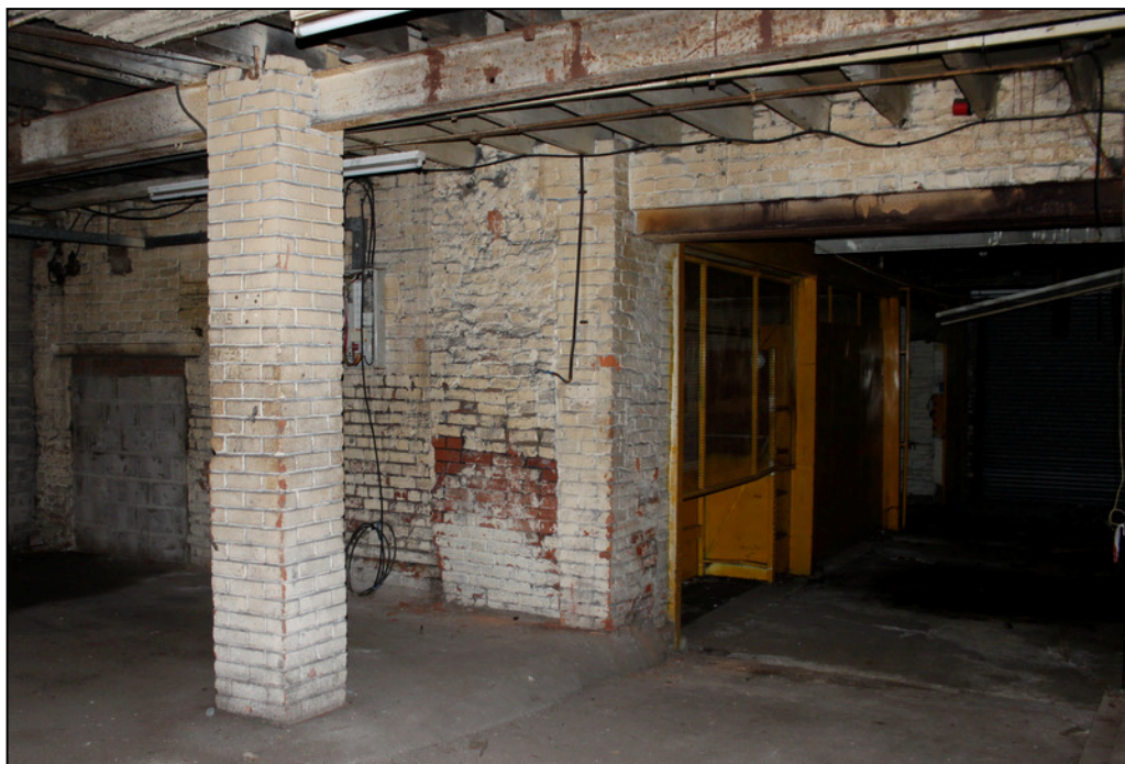
Plate 22: View across Bay 4, with steel cage across Bays 1-3 to rear
