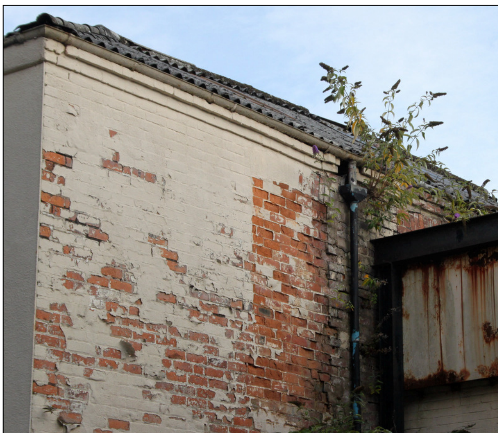
Plate 28: Blocked segmentally-arched windows in west external wall of Building C
