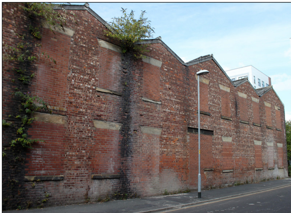
Plate 16: Detail of Hood Street elevation of Building B
