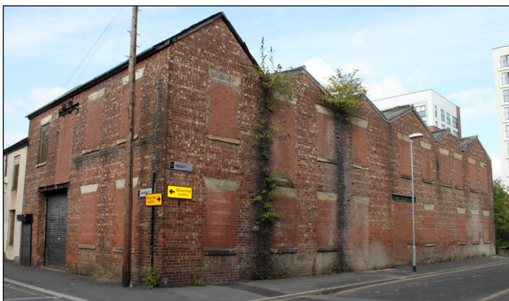
Plate 14: Hood Street Elevation of Building B
