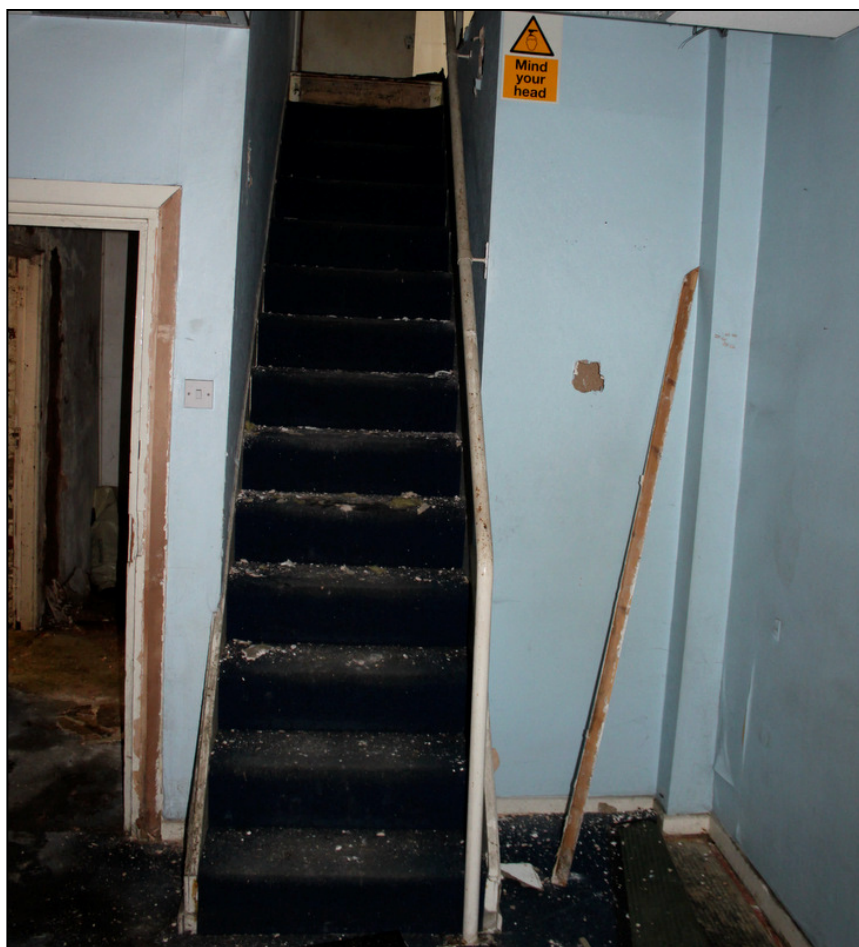
Plate 10: Inserted staircase within Building A, looking south
