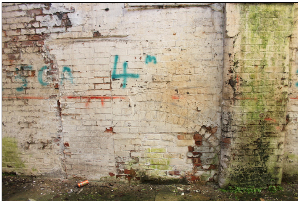
Plate 19: Segmentally-arched aperture in north wall of Building B
