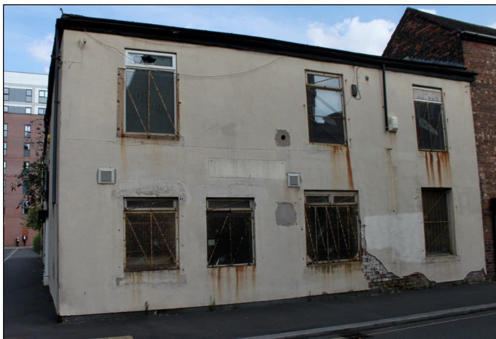
Plate 9: West elevation of Building A
