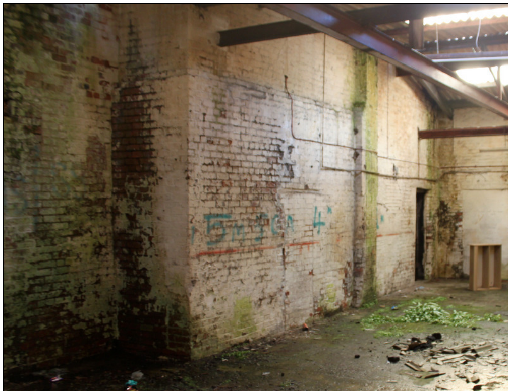
Plate 18: North external wall of Building B, looking south-west
