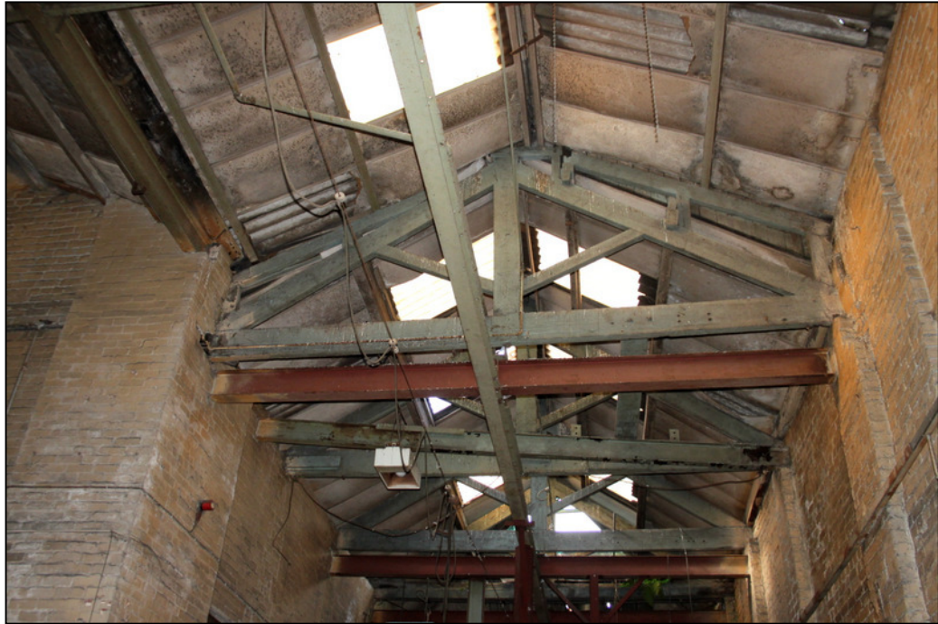
Plate 30: Internal view of Building C, with roof truss detail, looking north
