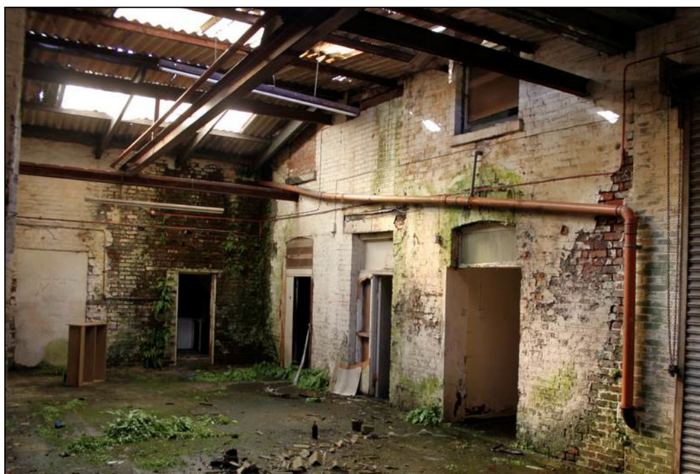
Plate 7: View of rear elevations of Building A, looking north-west
