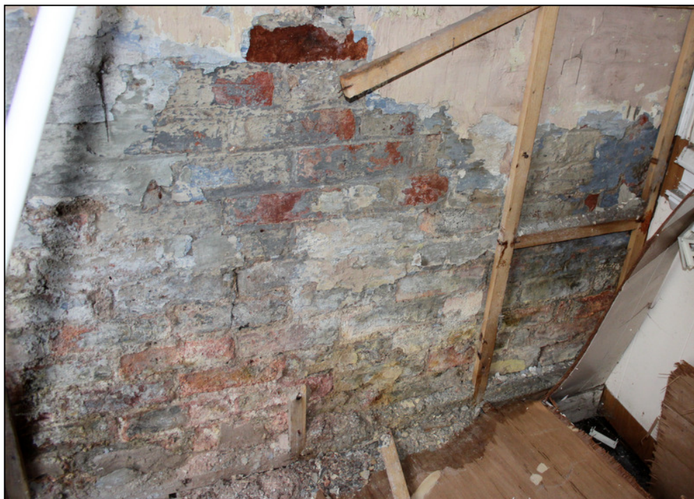
Plate 12: Chimney breast at first-floor level in west range of Building A
