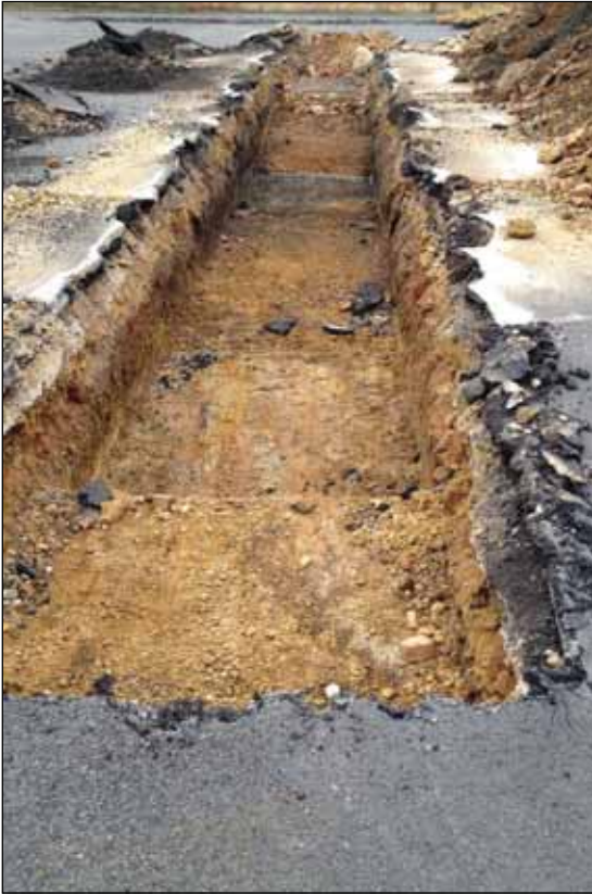
Plate 9: Trench 1, from the east
