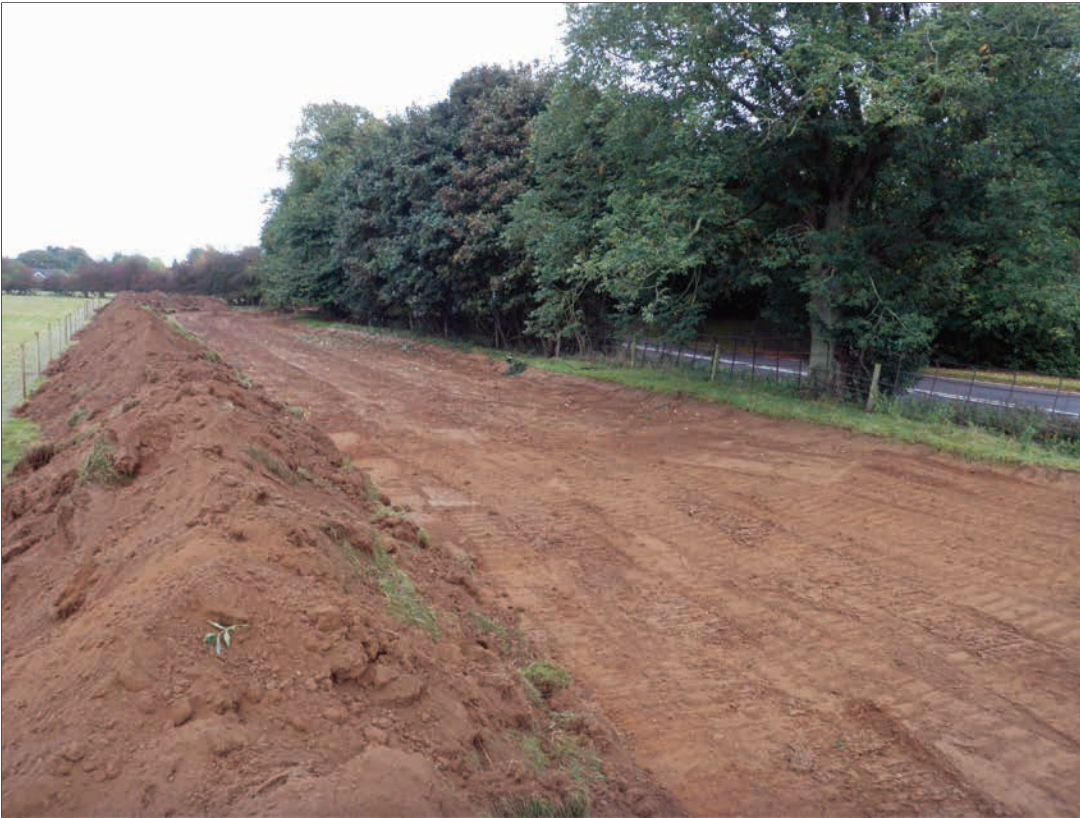
Plate 3: Stripping of Chainage 2000-2300
