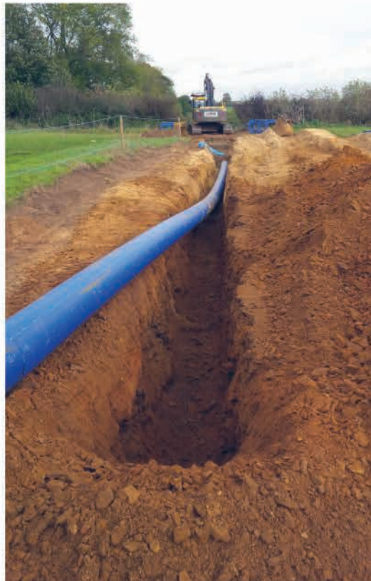
Plate 2: Trenching of pipe, Chainage 2000-2300
