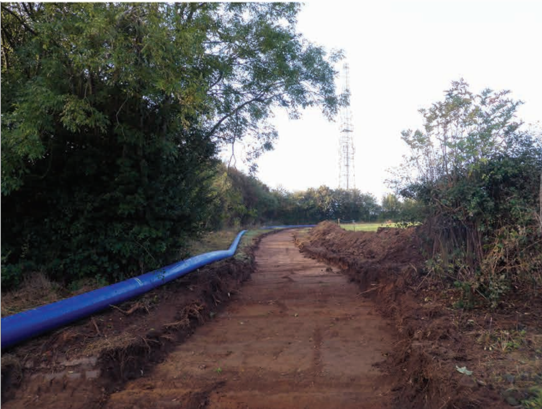
Plate 5: Chainage 2600-2900, looking north-west
