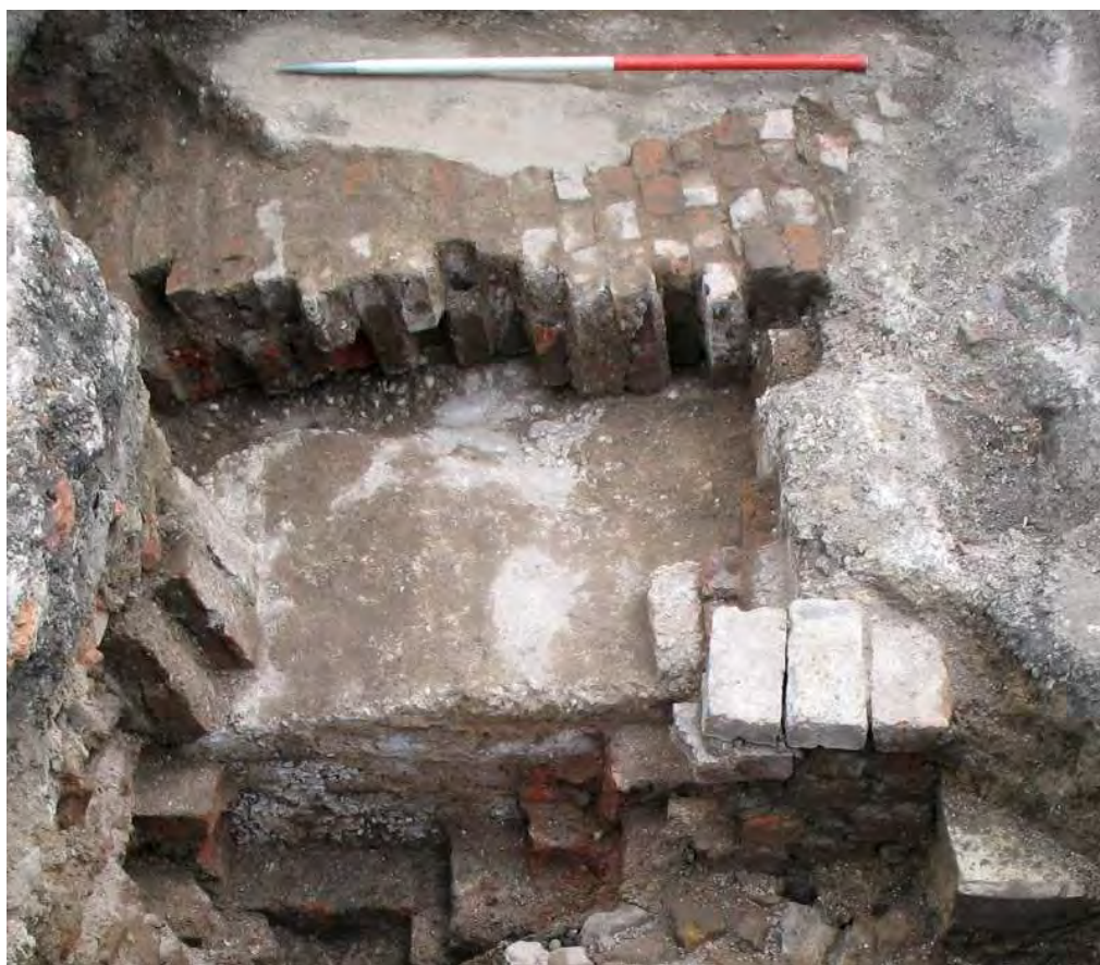
Plate 9: Vault (Room 231) with the roof and wall partially removed to reveal its concrete filling
