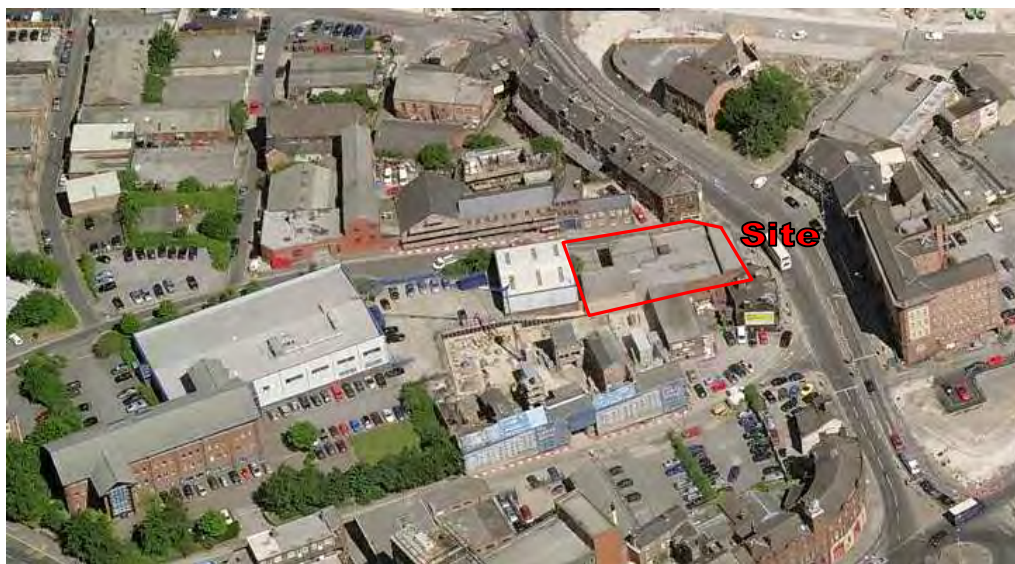
Plate 1: Aerial view of the site
