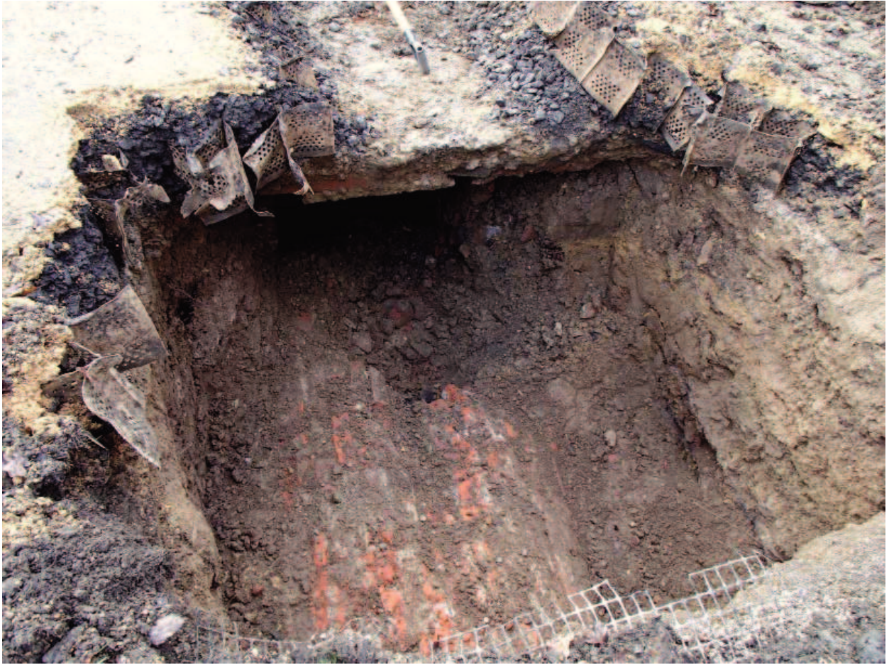
Plate 3: Showing state of condition of culvert
