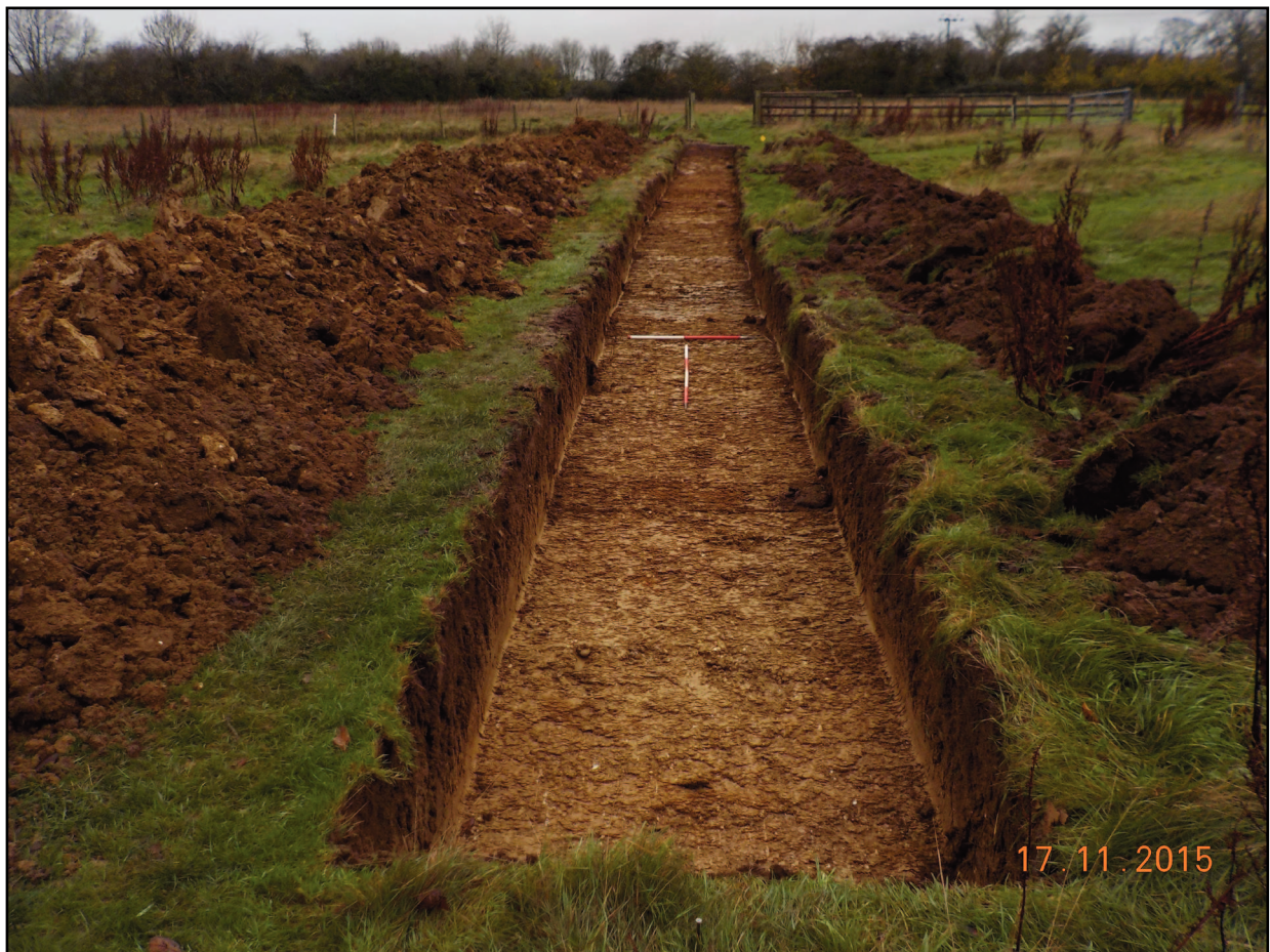
Plate 8: Trench 6 north-west facing view
