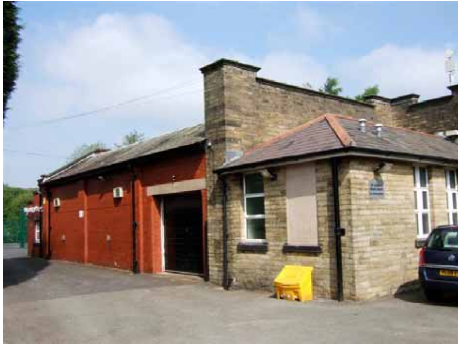
Plate 17: Rear of The Oswaldtwistle School (Site 35) showing twentieth century additions
