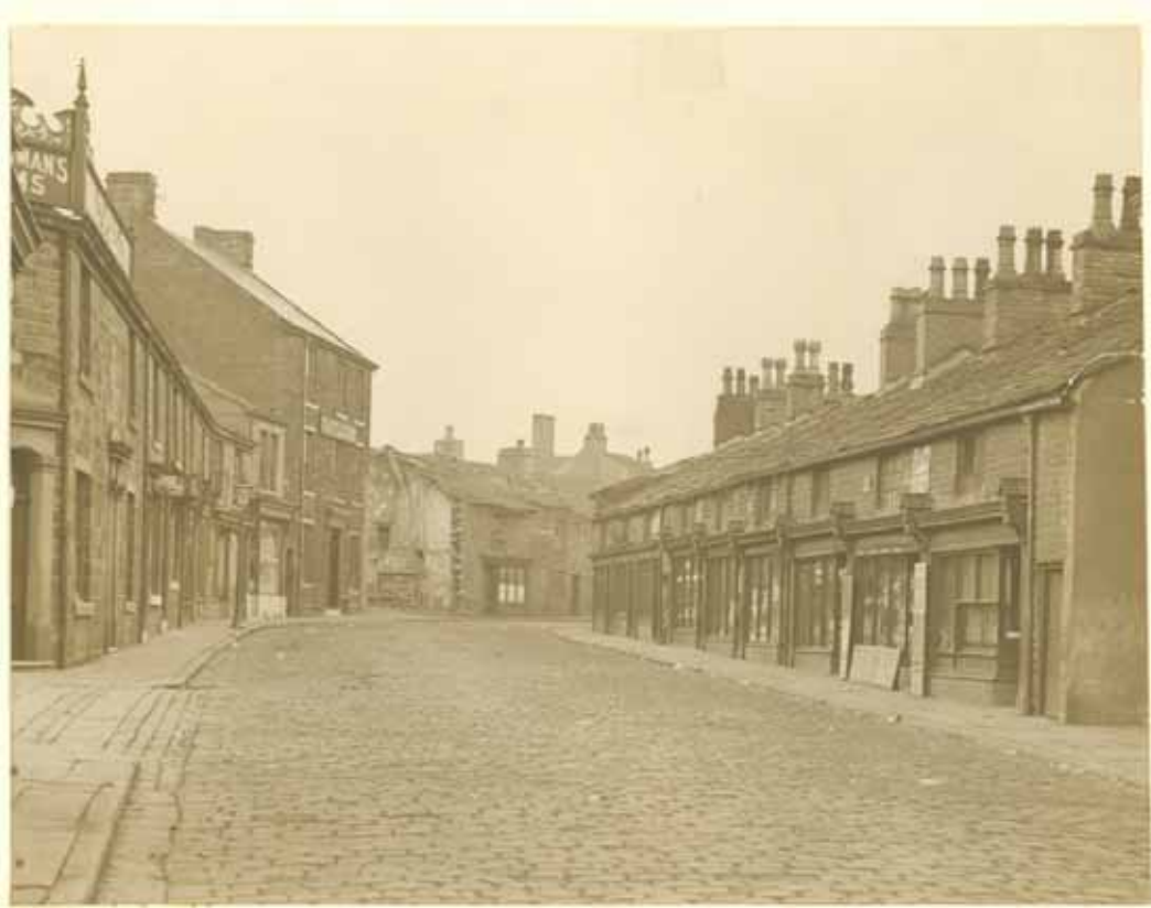
Plate 2: Treacle Row, Oswaldtwistle from Union Road. The building in the foreground of Plate 1 is visible on the left side of Union Road
