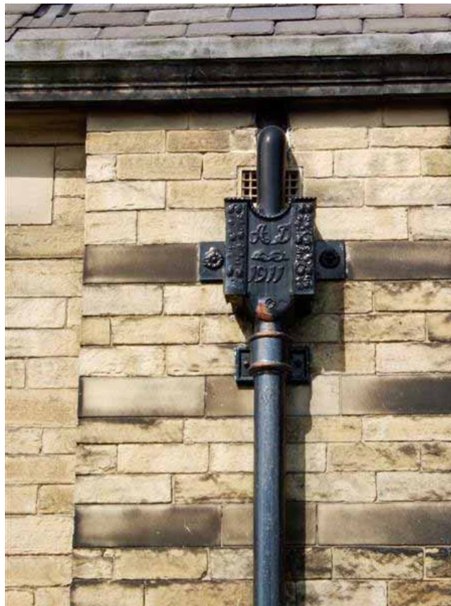
Plate16: Drainpipe on the front of Oswaldtwistle School showing construction date of 1911
