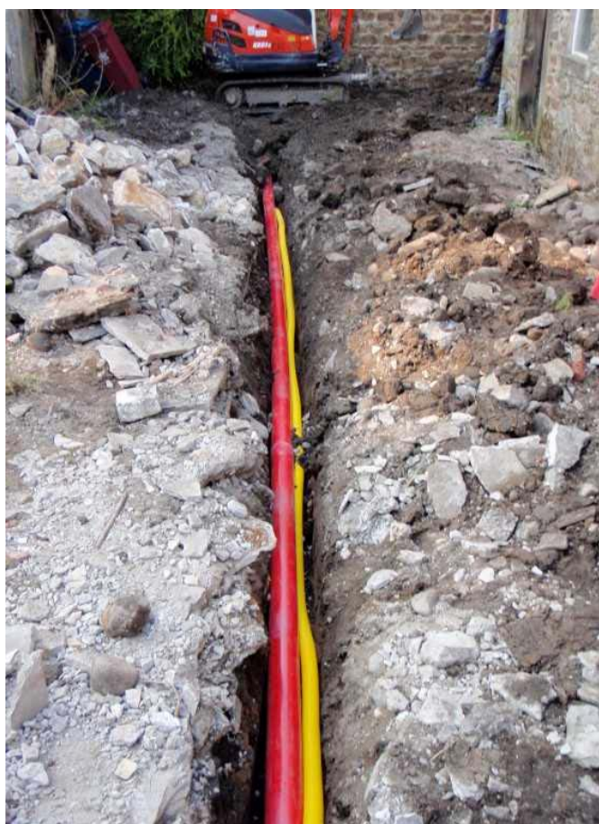
Plate 2: the rear of 29 Church Street after excavation
