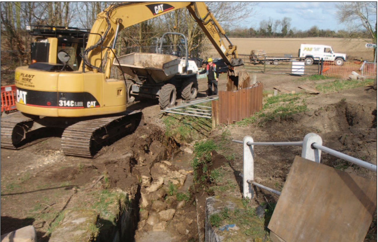
Plate 4: Digging out for new channel
