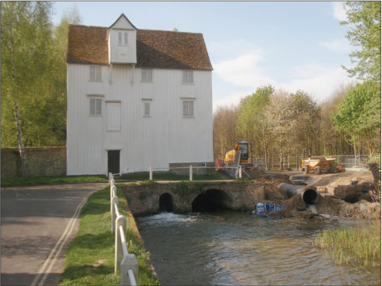
Plate 7: Mill and works, without bridge
