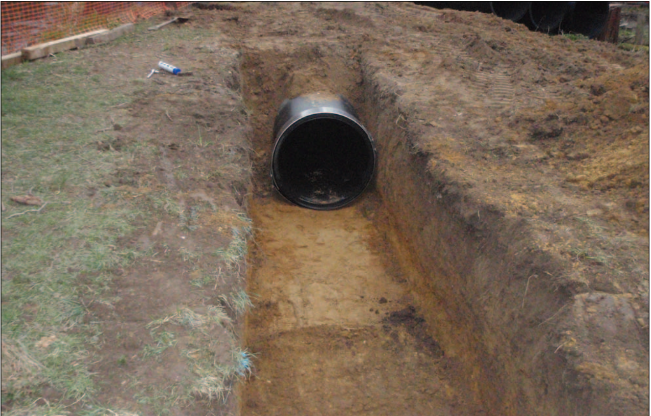
Plate 3: Pipe trench and Pipe
