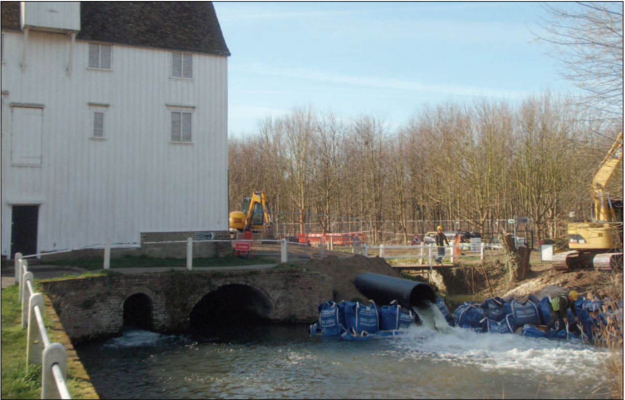
Plate 1: Temporary pipe and Mill
