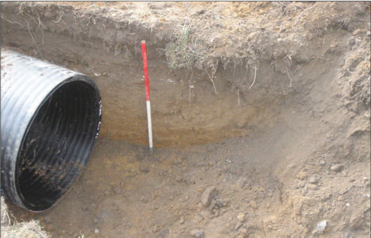
Plate 2: Section 1 of pipe trench
