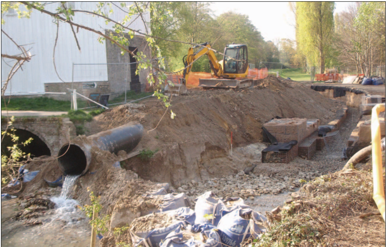
Plate 5: Stone cages for sides of new channel
