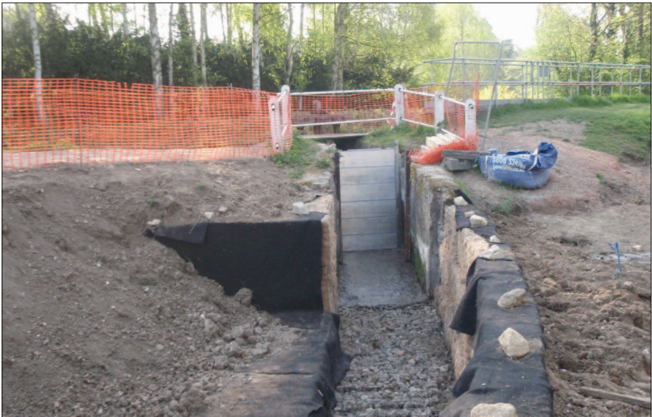
Plate 6: Sluice Gate in new channel
