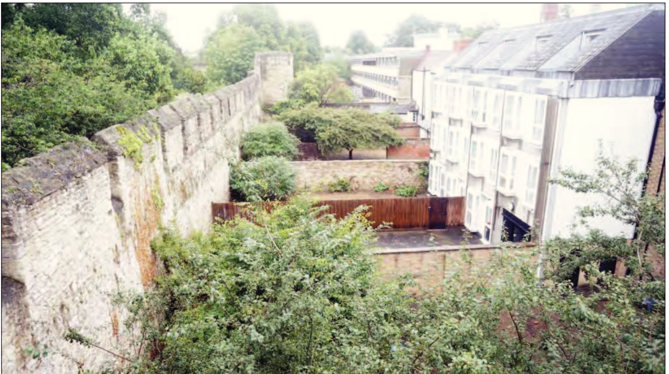
Figure 4: View of the site looking S with Bodicote House in the right foreground and the Sacher Building behind. Bastion 25 is also visible
