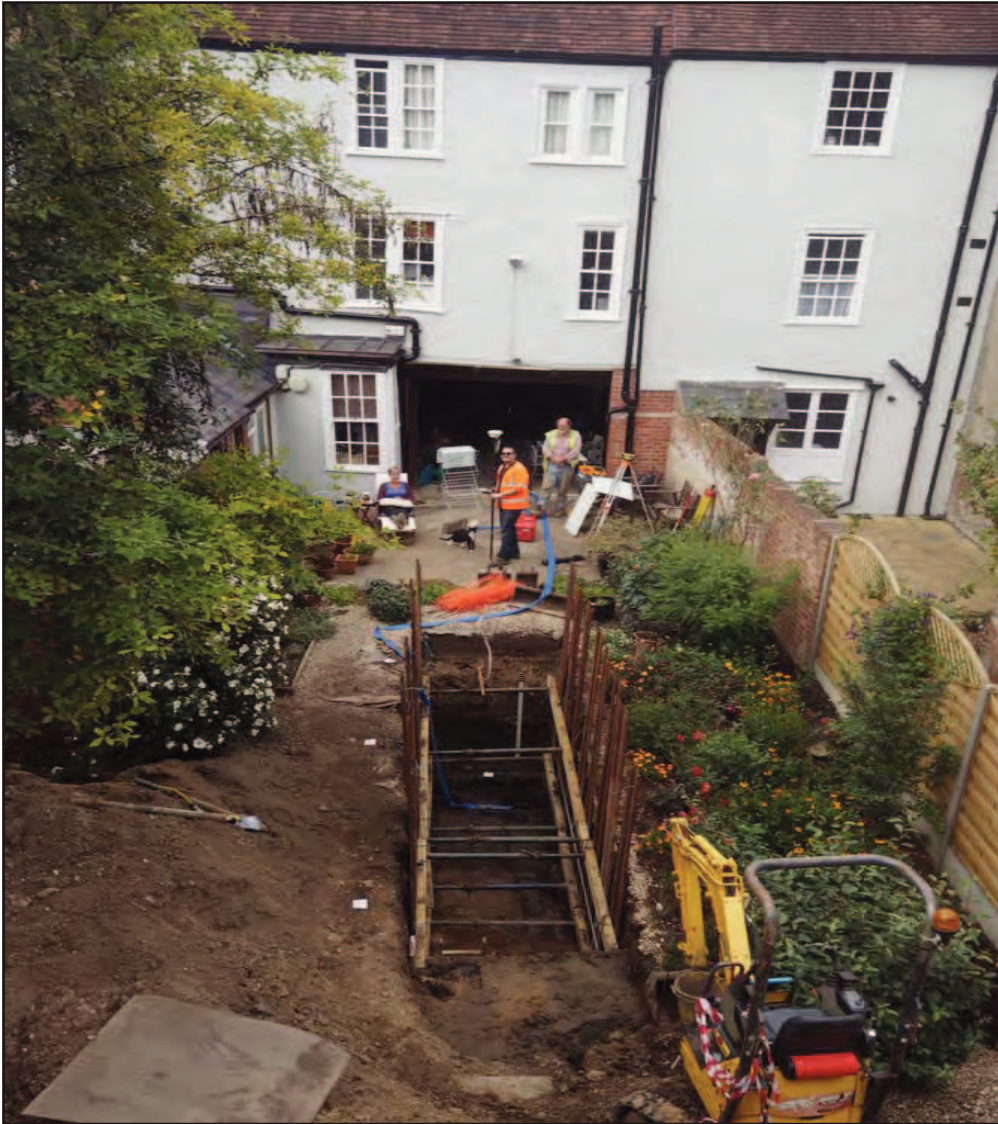
Figure 12: Trench 2 under excavation
