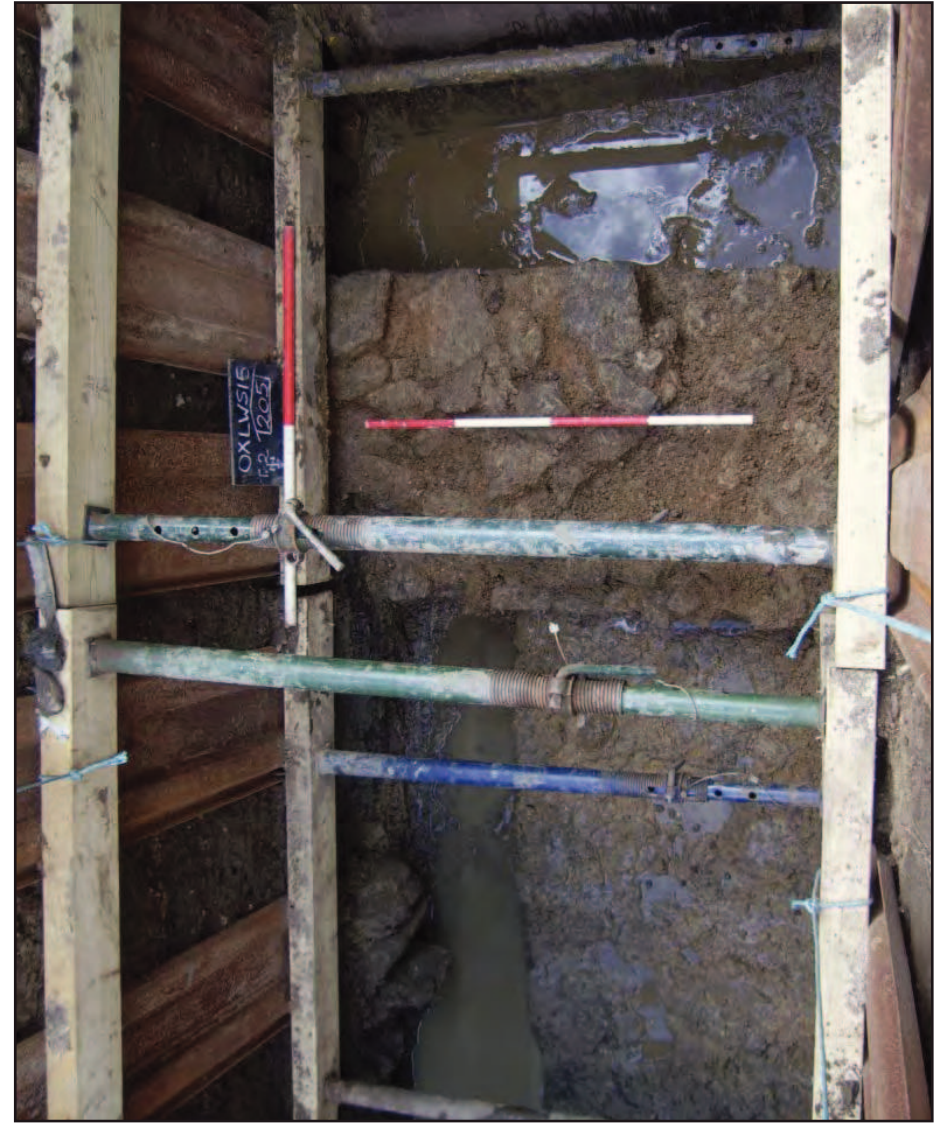
Figure 13: Trench 2 footing 205 of outer town wall
