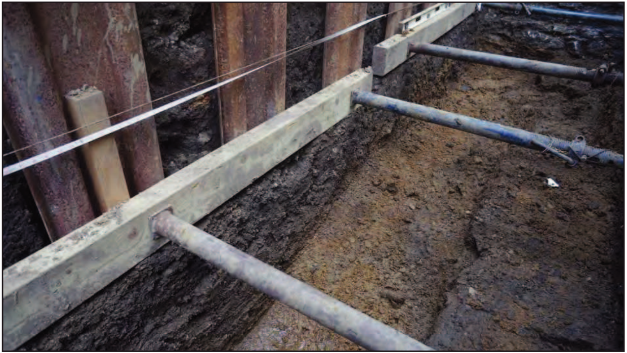
Figure 15: Trench 3 after excavation
