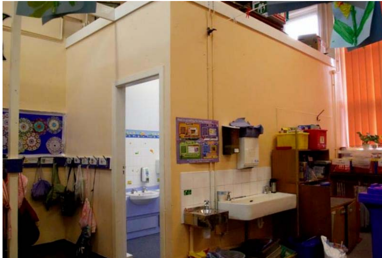
Plate 4 Example of a partition wall
