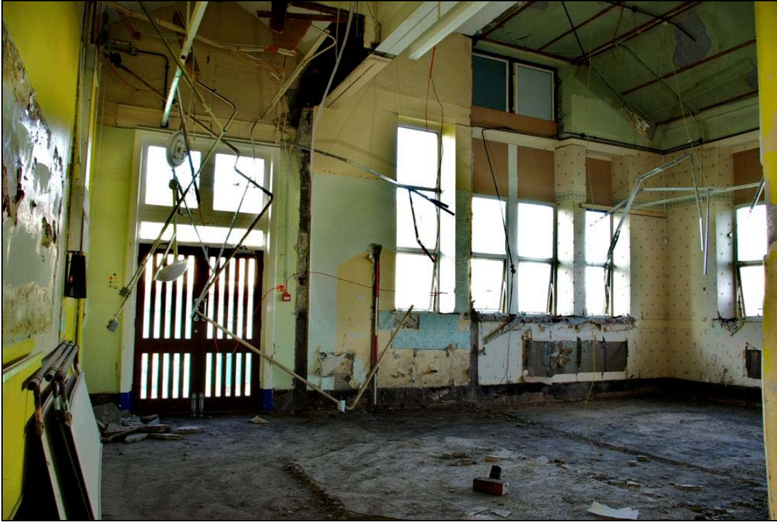
Plate 18: Rooms 46-52 following stripping
