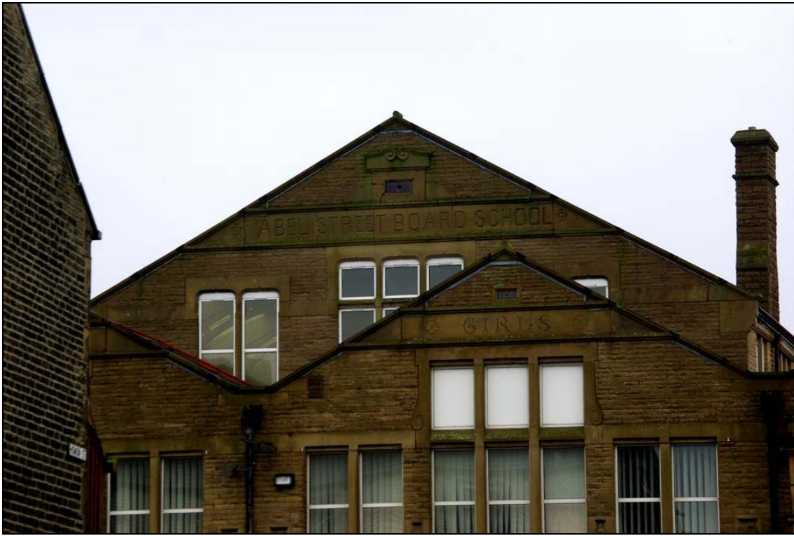
Plate 12: View of west elevation of the main hall of the Junior School
