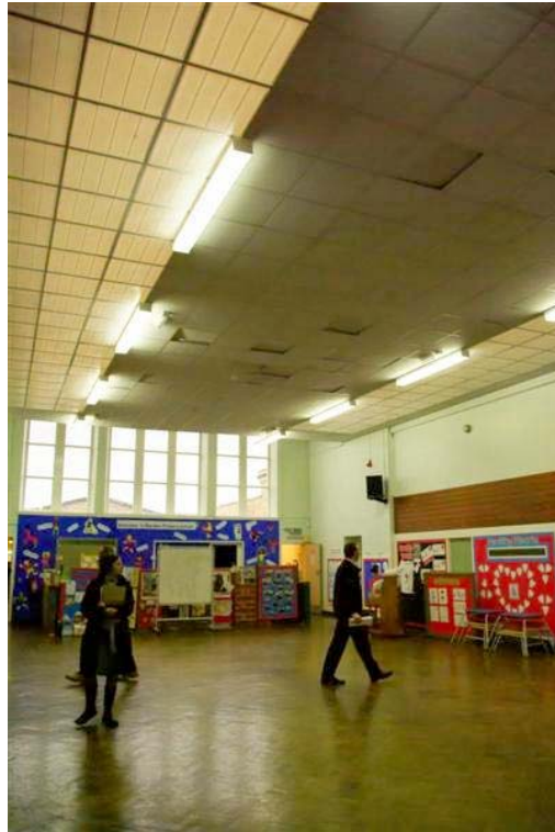
Plate 2 Ceiling to be removed in main hall of the infant block
