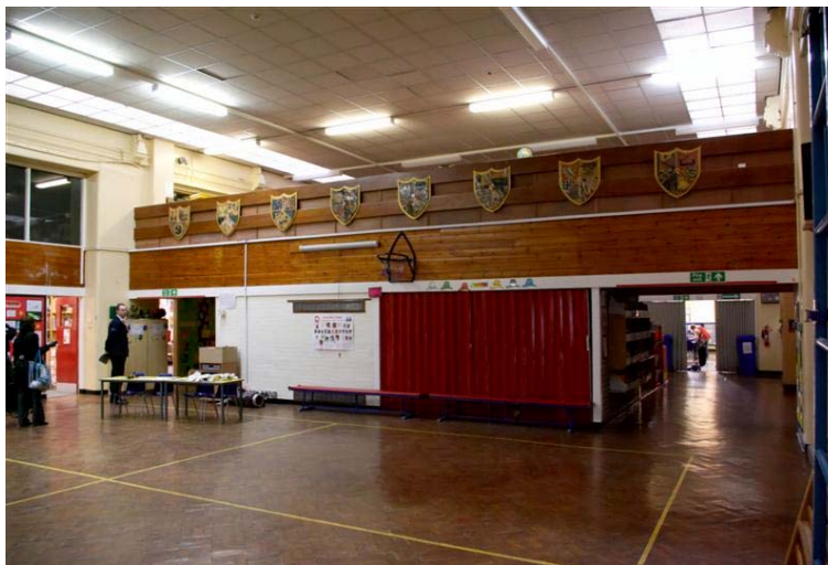
Plate 3 Mezzanine to be removed in the main hall of the senior school
