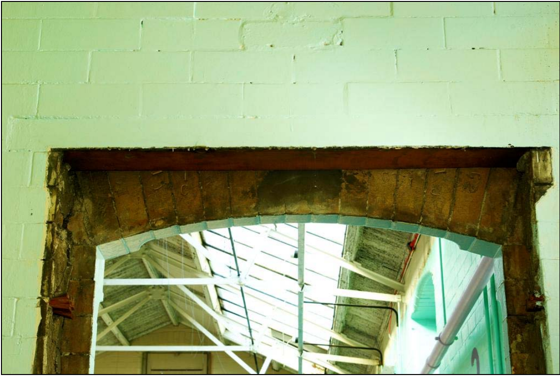
Plate 64: Segmental arch of the doorway from Room 100 to Room 60 in the Science Building
