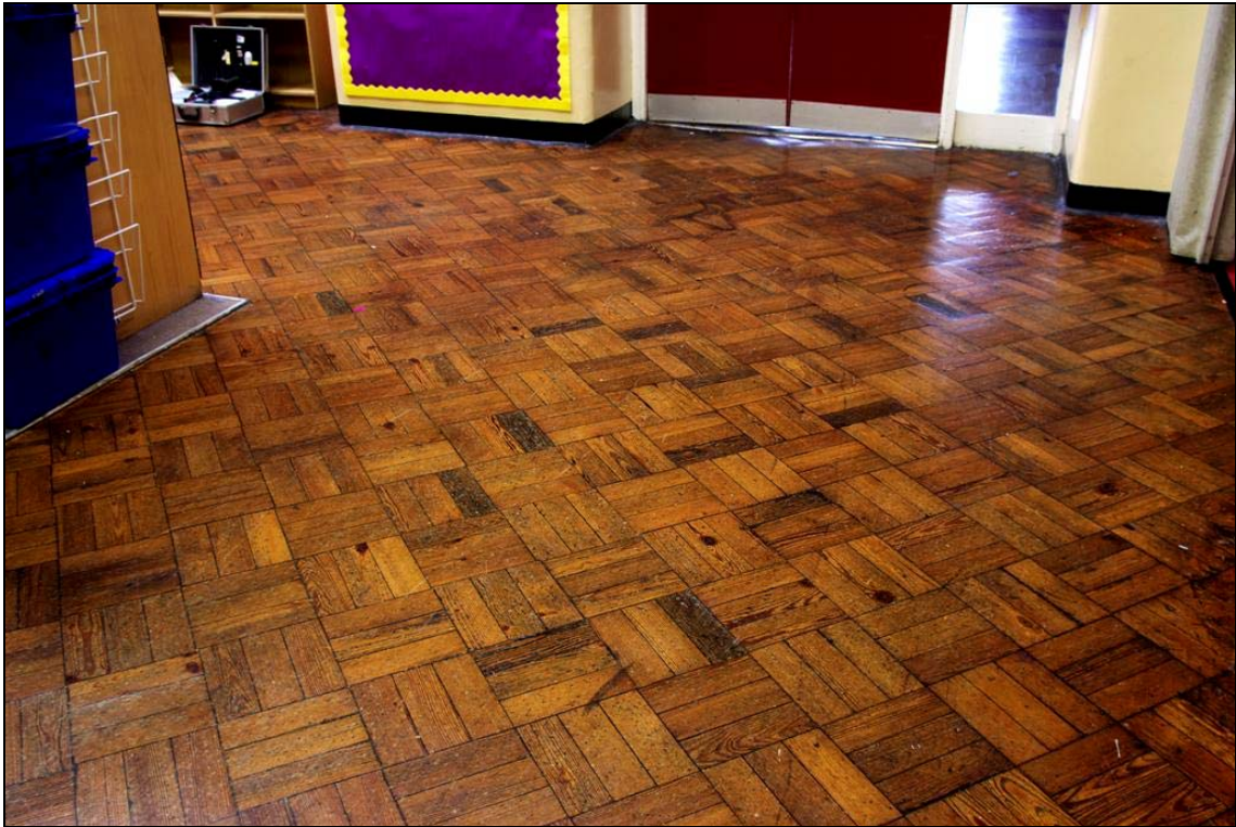
Plate 24: Square pattern block flooring
