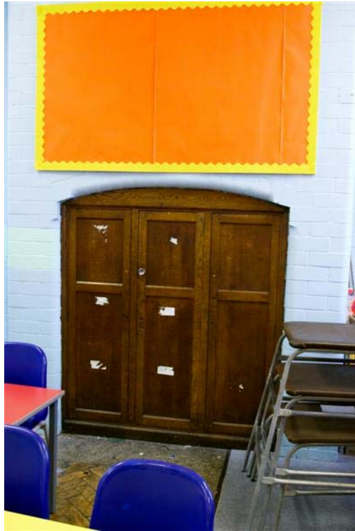
Plate 6 Example of fabric to remain in situ
