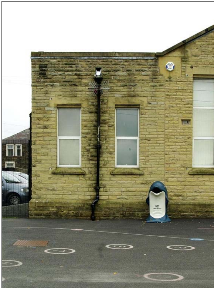
Plate 13: East side of the north elevation of the Junior School showing butt-joint
