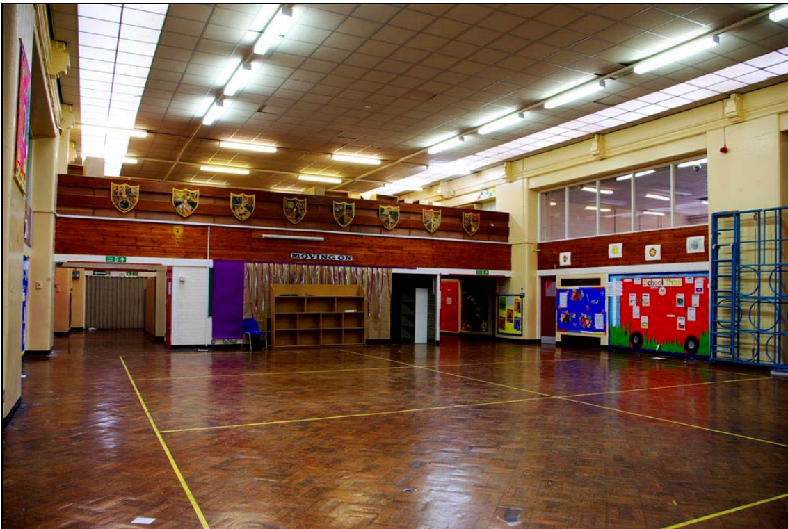
Plate 35: View of the main hall in the Junior School prior to stripping (facing north-west)
