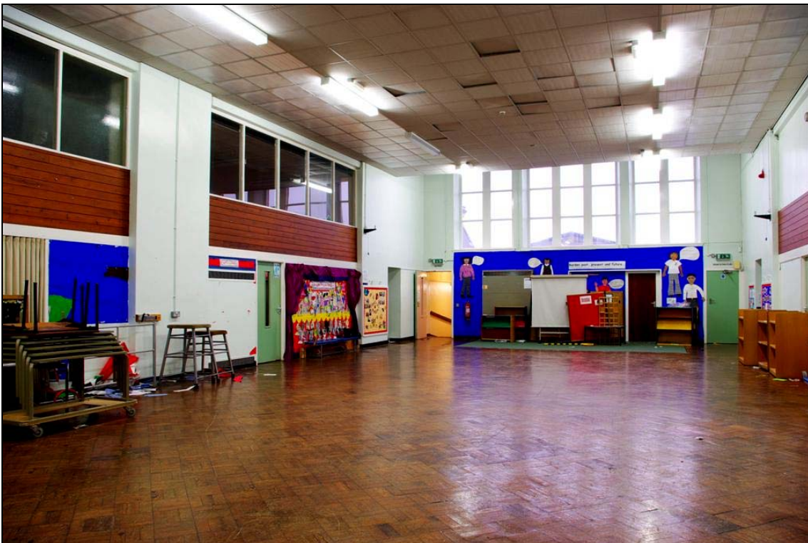
Plate 55: General view of the main hall (Room 29) in the Infants School (facing north) prior to stripping
