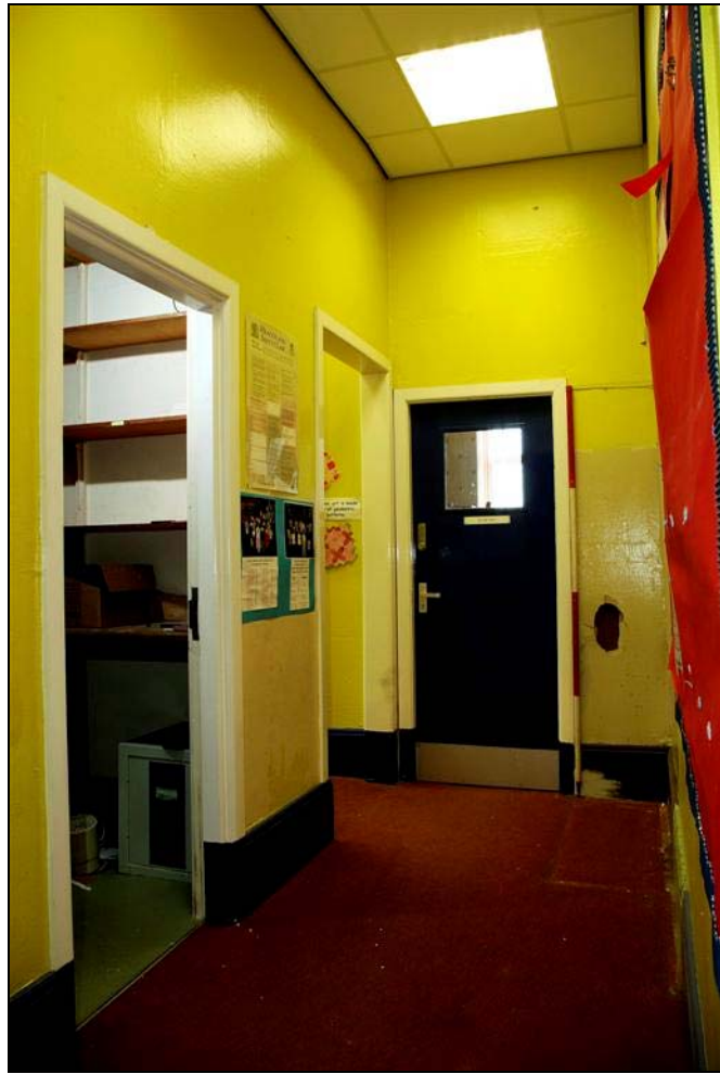
Plate 16: General Appearance of Rooms 46-52
