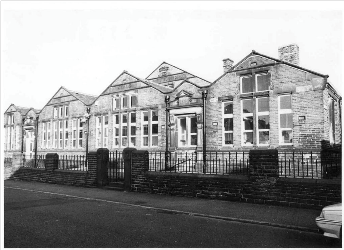
Plate 3: Main elevation of Abel Street School, 1980s
