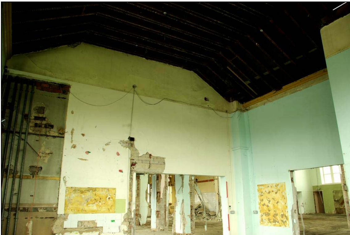
Plate 53: Example of a classroom in the Infant School following stripping
