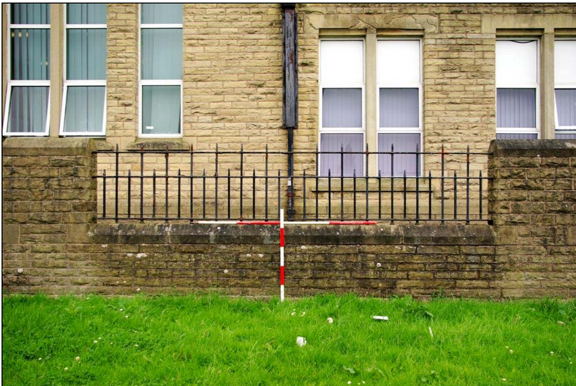
Plate 49: Example section of the original appearance of the perimeter wall
