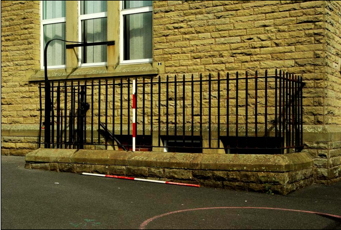
Plate 46: Steps down to basement on the principal elevation of the Infant School
