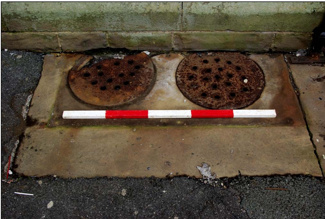
Plate 15: Coal chute on the south side of the Junior School
