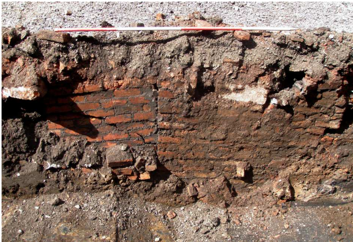
Plate 5: Walls 103 and 104 exposed in Trench 1
