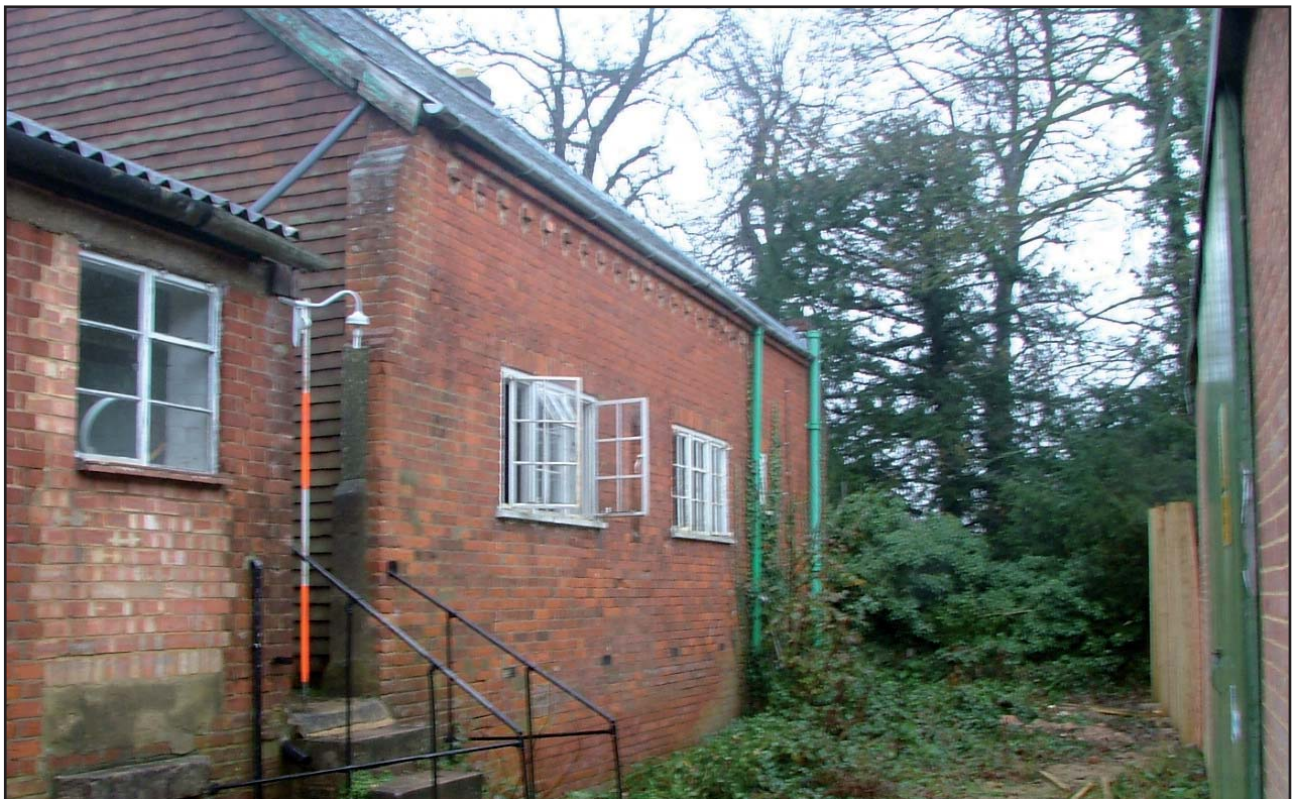
Plate 6: South and west walls of the staff cottage
