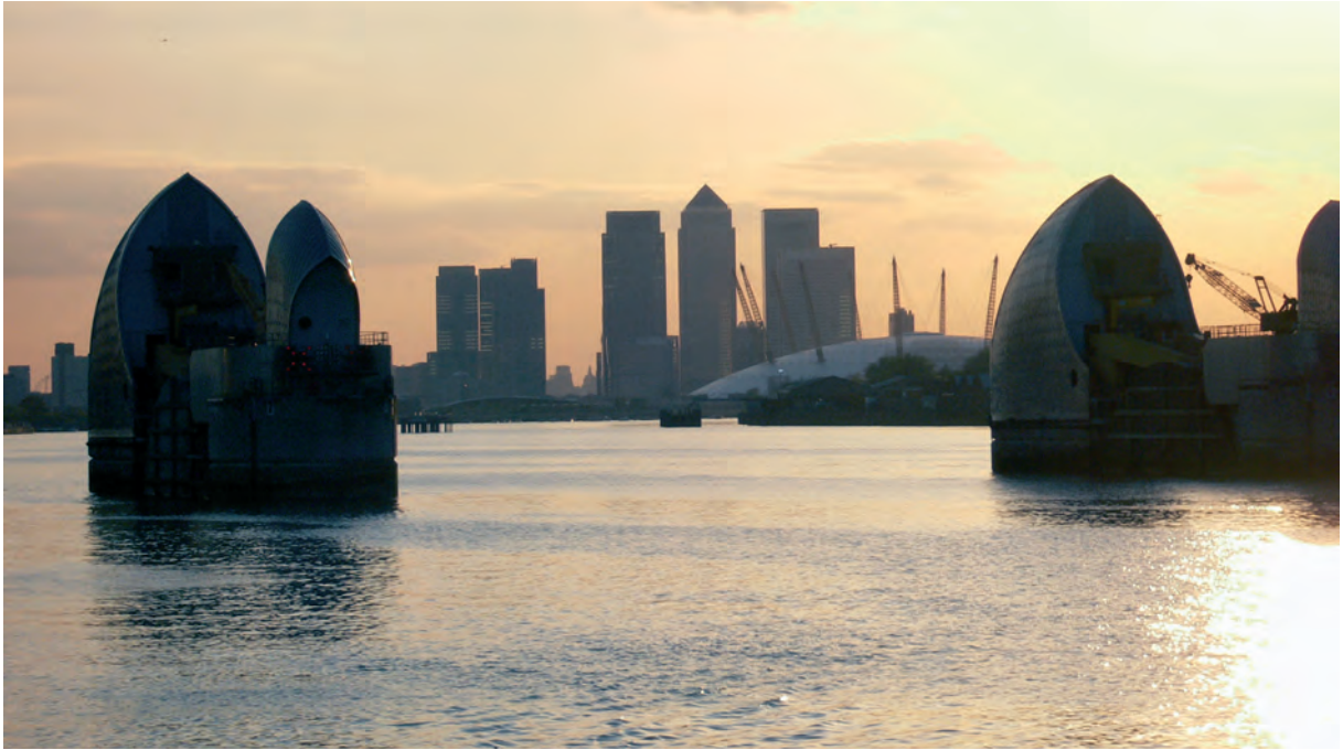
Plate 22 Thames Barrier at Woolwich (photo by Herry Lawford)
