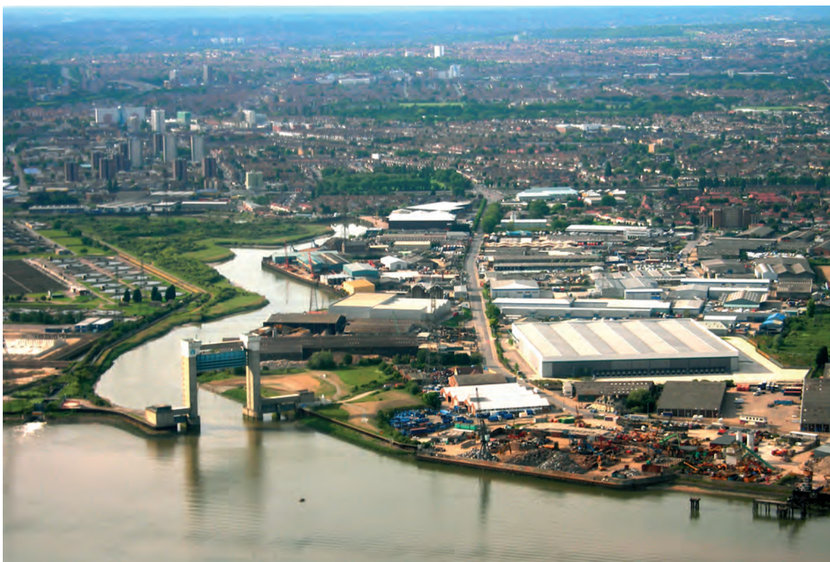
Plate 23 Flood defences at Barking Creek on the River Roding (photo by Lars Plougmann)
