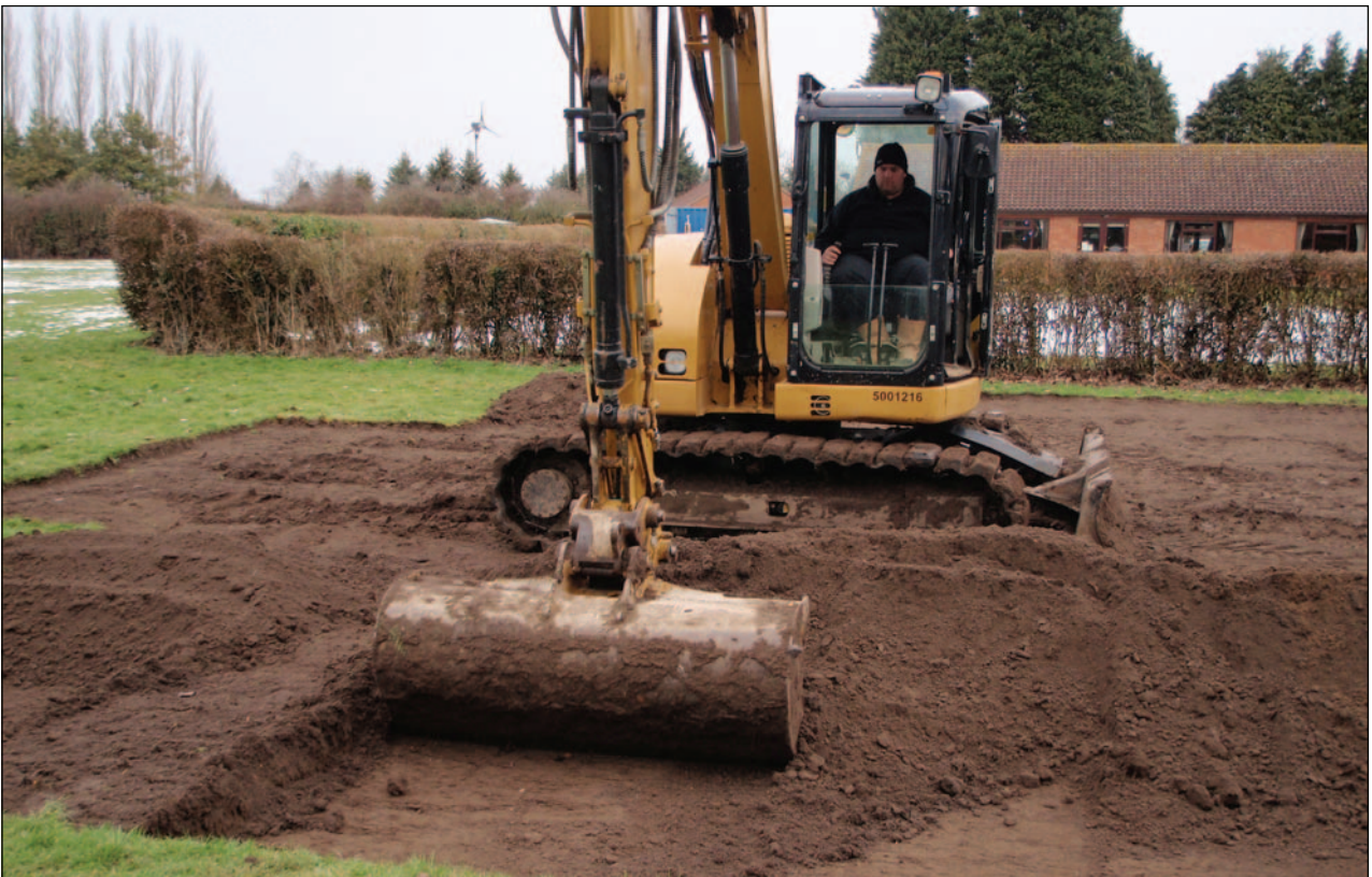
Plate 2: Removal of topsoil
