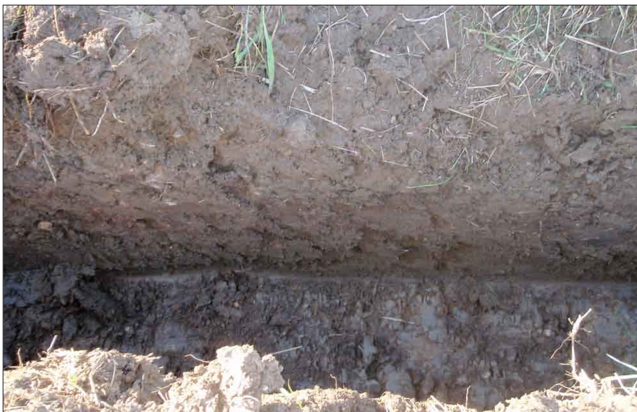
Plate 1: Section showing build up of modern material
