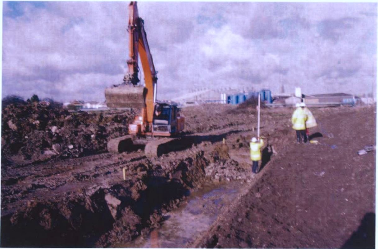
Plate 1: Drainage ditch excavations. Looking West
