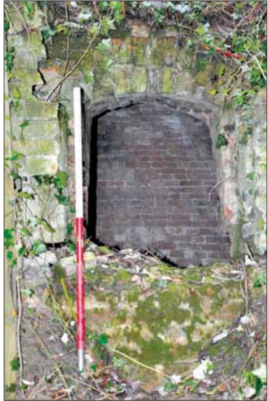
Plate 10: Inner doorway and surrounding brickwork, viewed from the east.
