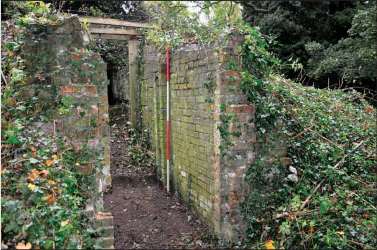
Plate 15: The northern wall and position of the new doorway, seen from the south-east.
