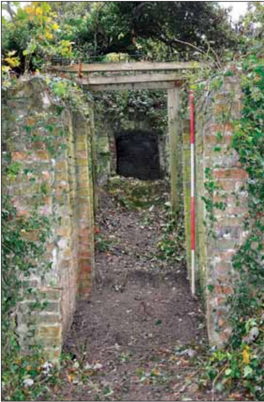
Plate 7: View of the inner ice house door, viewed from the south-east
