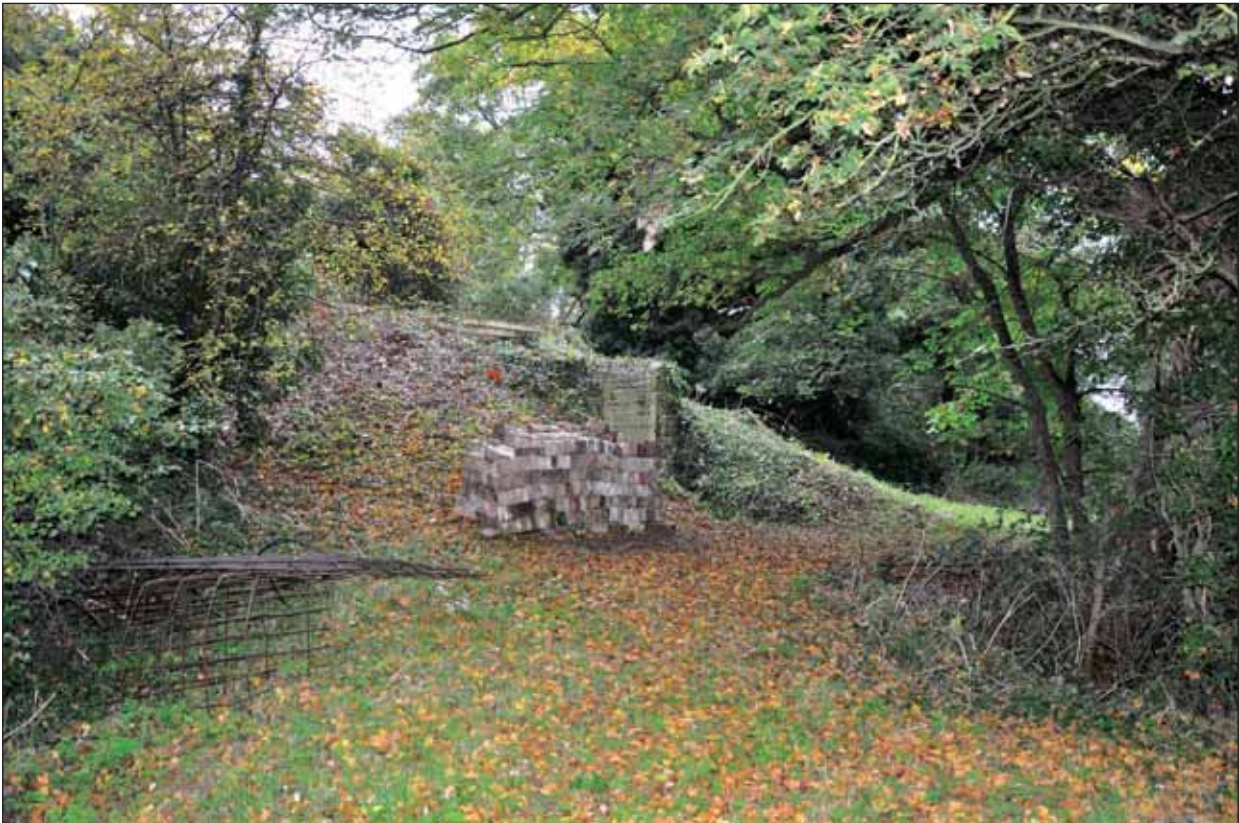
Plate 1: View of the ice house, from the south-east
