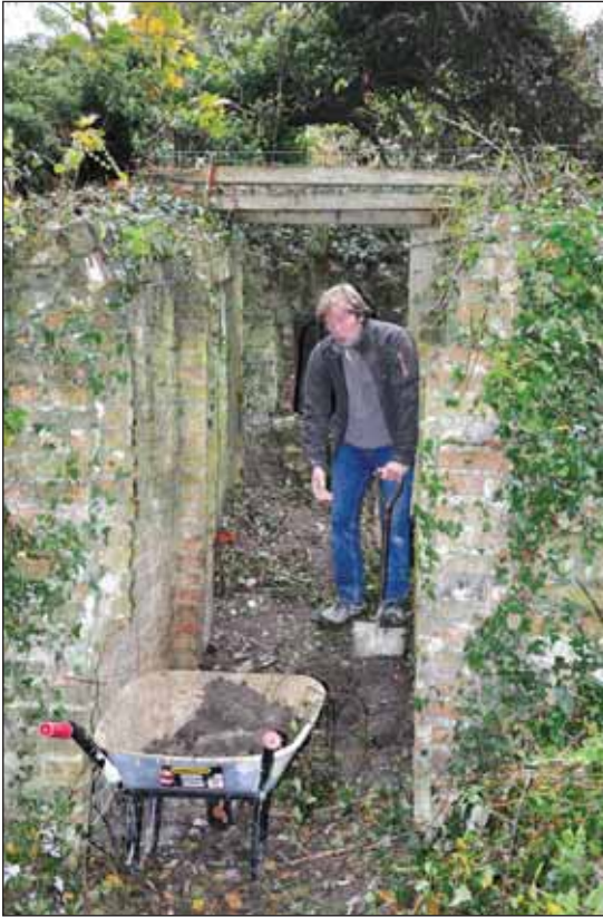
Plate 5: Removal of soil from the entrance, viewed from the east.
