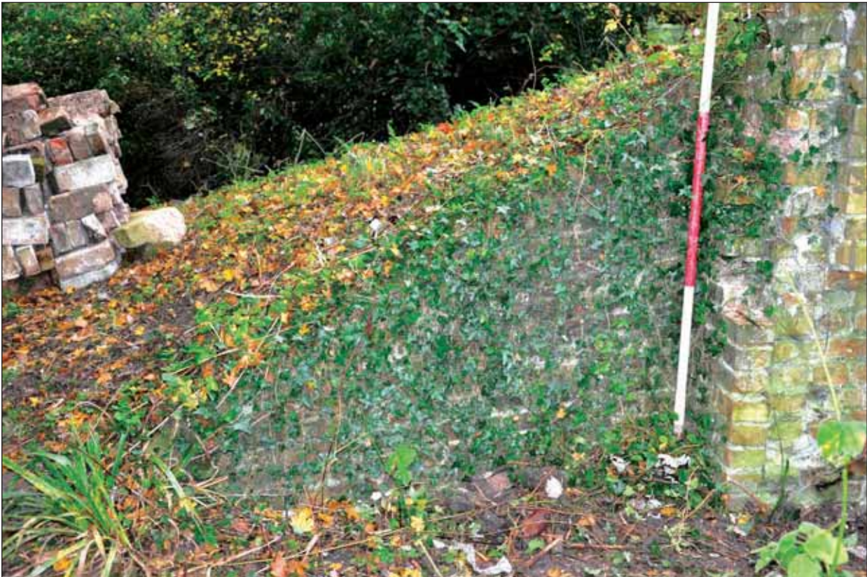
Plate 11: Detail of the retaining wall at the entrance to the Ice house, viewed from the north.
