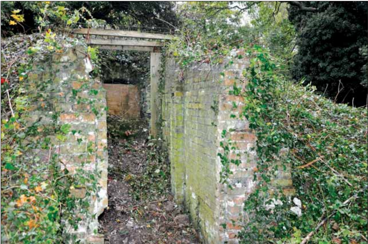
Plate 6: The northern wall prior to soil removal, viewed from the east.
