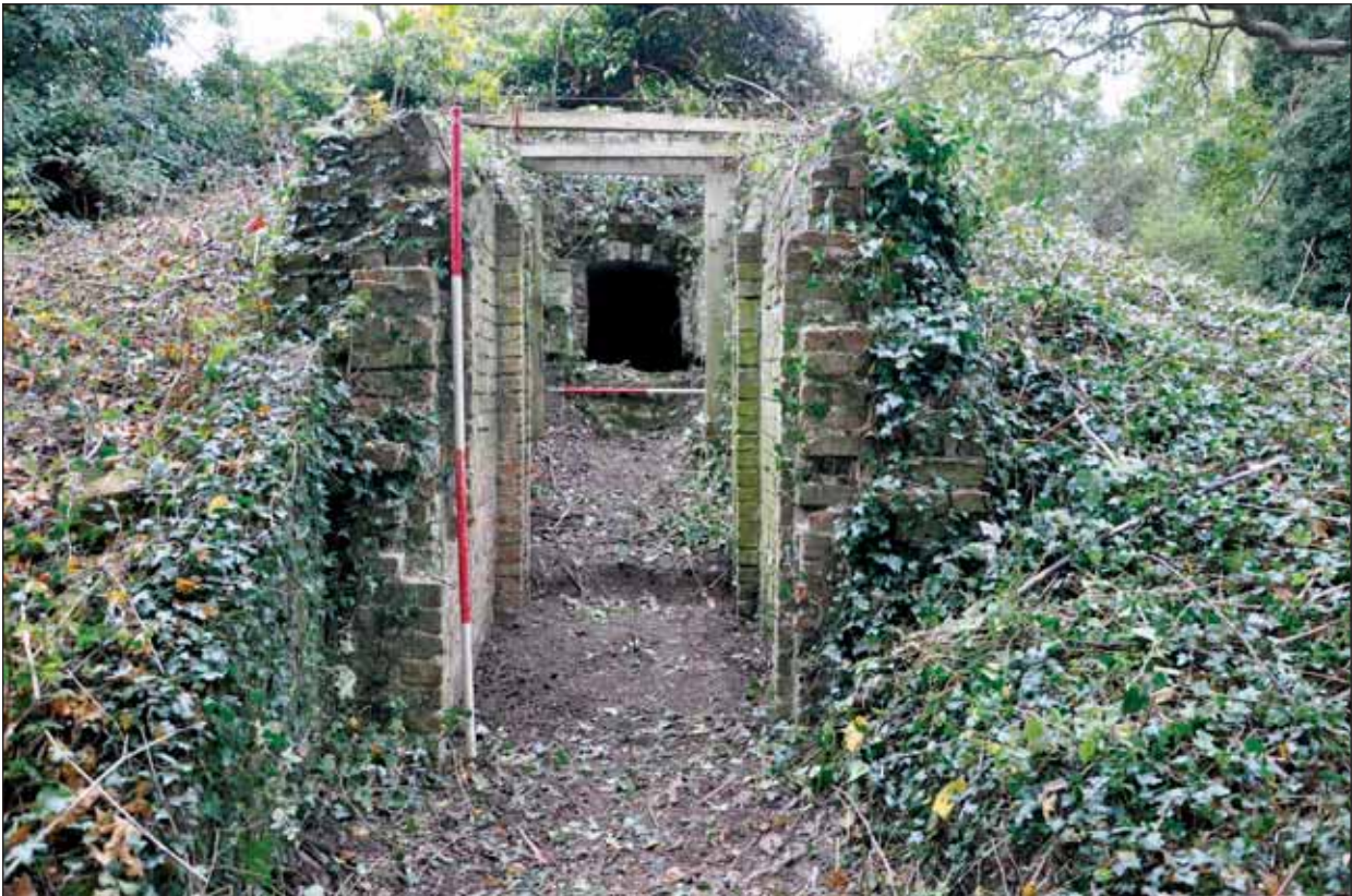
Plate 16: Pillars to outer entrance way, seen from the east.
