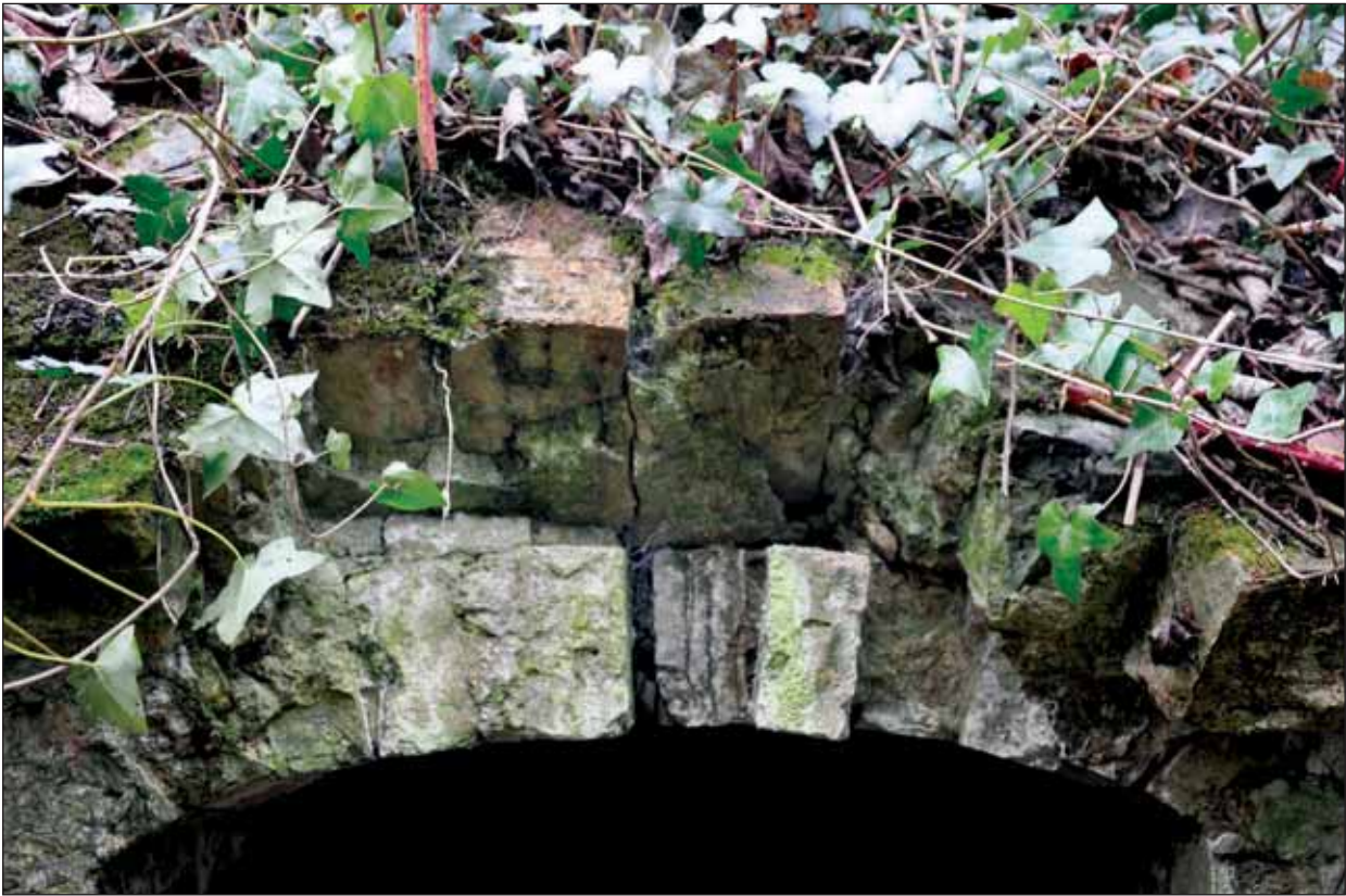
Plate 13: Detail of brick arch above the inner entrance to the ice house, seen from the east.
