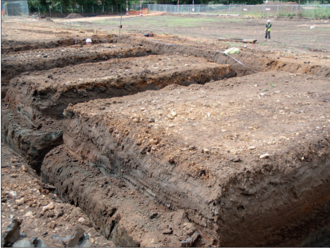
Plate 1: Overview of site with foundation trenches for plots 1-4 in foreground and plots 8-11 marked out on lower terrace in background.
