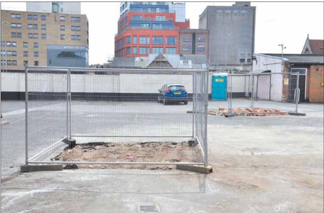
Plate 10: Location of backfilled Test Pit 1 and 2, from north-east.
