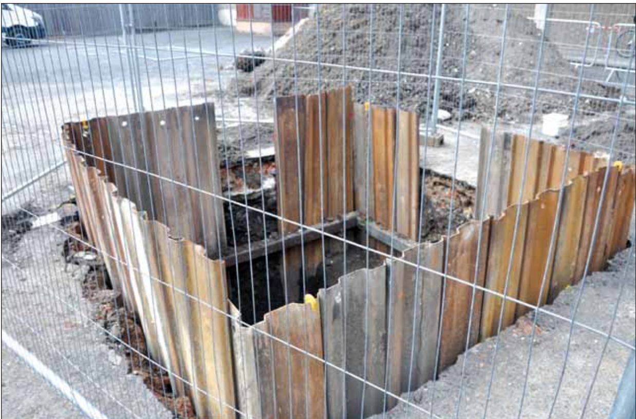
Plate 6: Shoring around Test Pit 2, from south-east.
