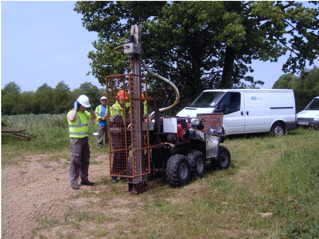
Plate 1: Auger drilling to a depth of 2m in preparation for the seismic charge at TP1
