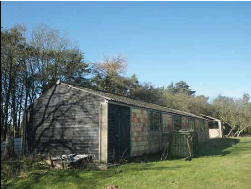
Plate 14: Standing MoWP huts to the east of the development area, view from south-east.
