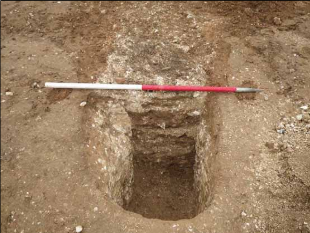
Plate 7: Service ditch terminus 131, view from the west.
