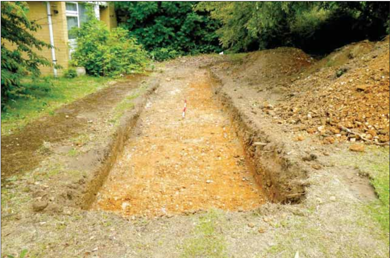
Plate 2: General shot of Trench 2 looking north-east
