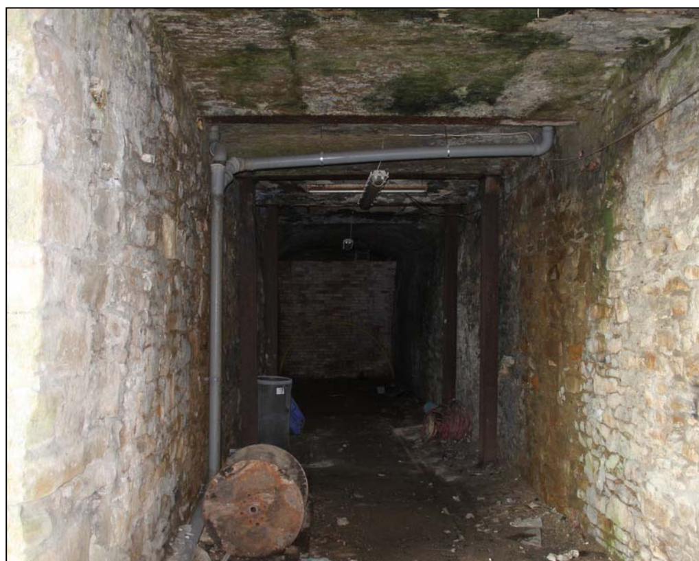
Plate 11: Access tunnel beneath Manchester Road
