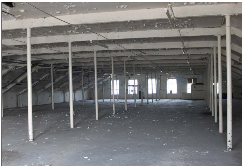
Plate 18: Wide, open attic space in Britannia Mill
