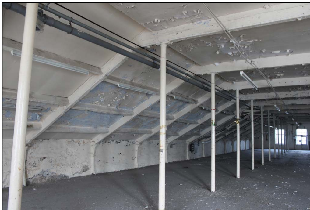
Plate 19: Column and cast-iron raised foot carrying principal rafter of roof truss
