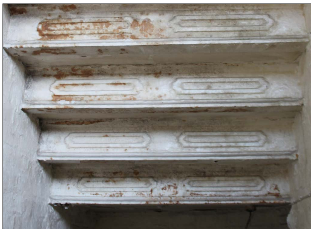
Plate 9: Decorative cast-iron risers in stair tower
