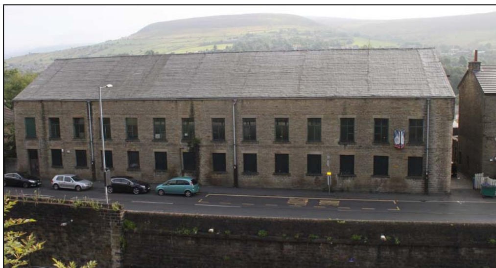
Plate 13: View of Britannia Mill from the west
