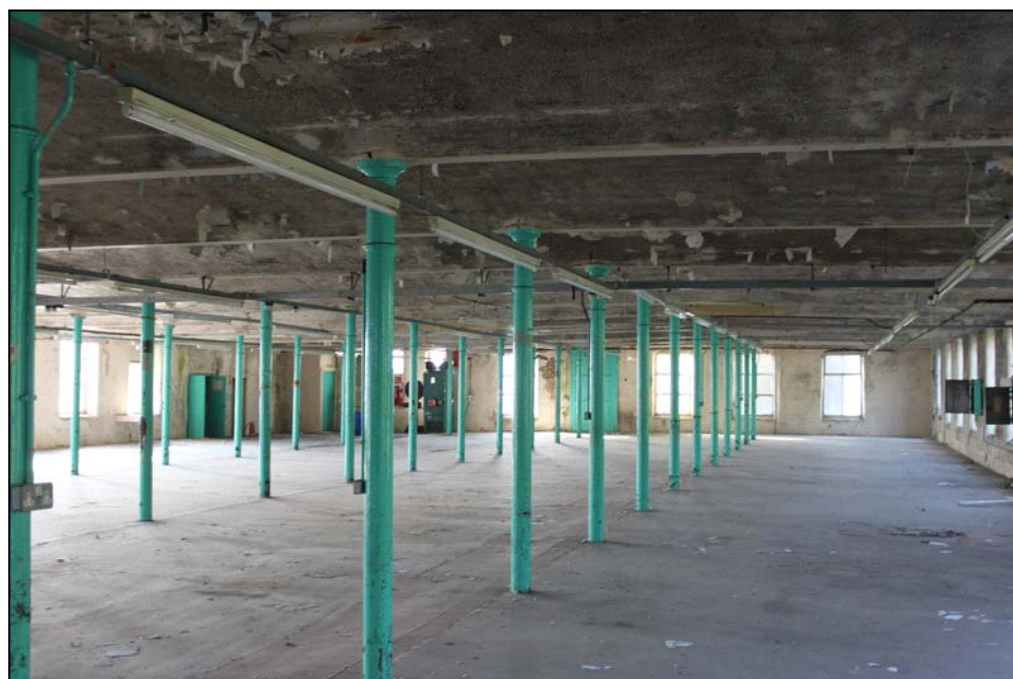
Plate 16: First floor of Britannia Mill, showing fireproof construction
