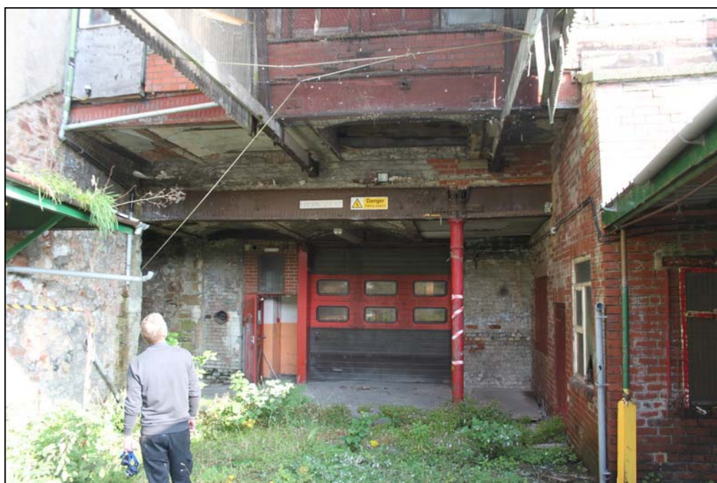
Plate 10: Loading bay added to southern elevation of Britannia Mill
