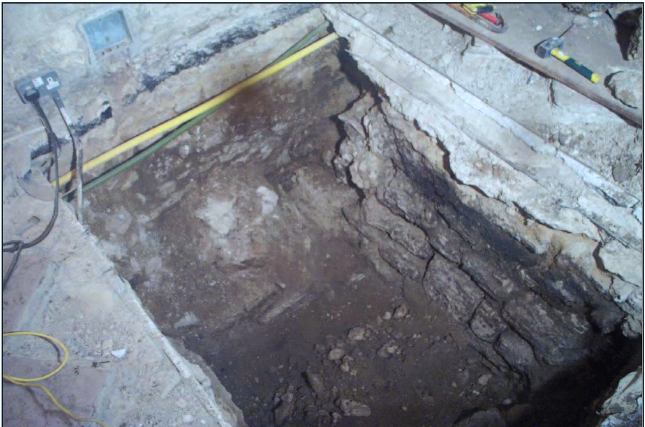
Plate 6: Trench 3 Footing 313 following partial dismantling of wall 305
