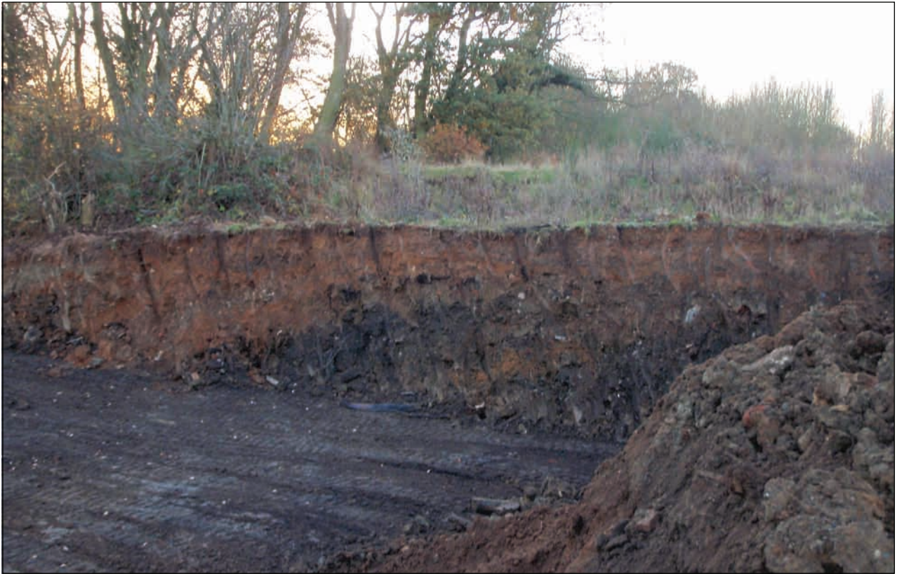
Plate 4: The eastern end of the site, showing 3m thickness of dumped material against the dam. View from the north.
