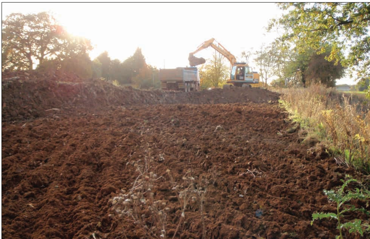
Plate 2: The site of the swimming pool at the eastern end of the site, before removal of dumped material. View from the west.
