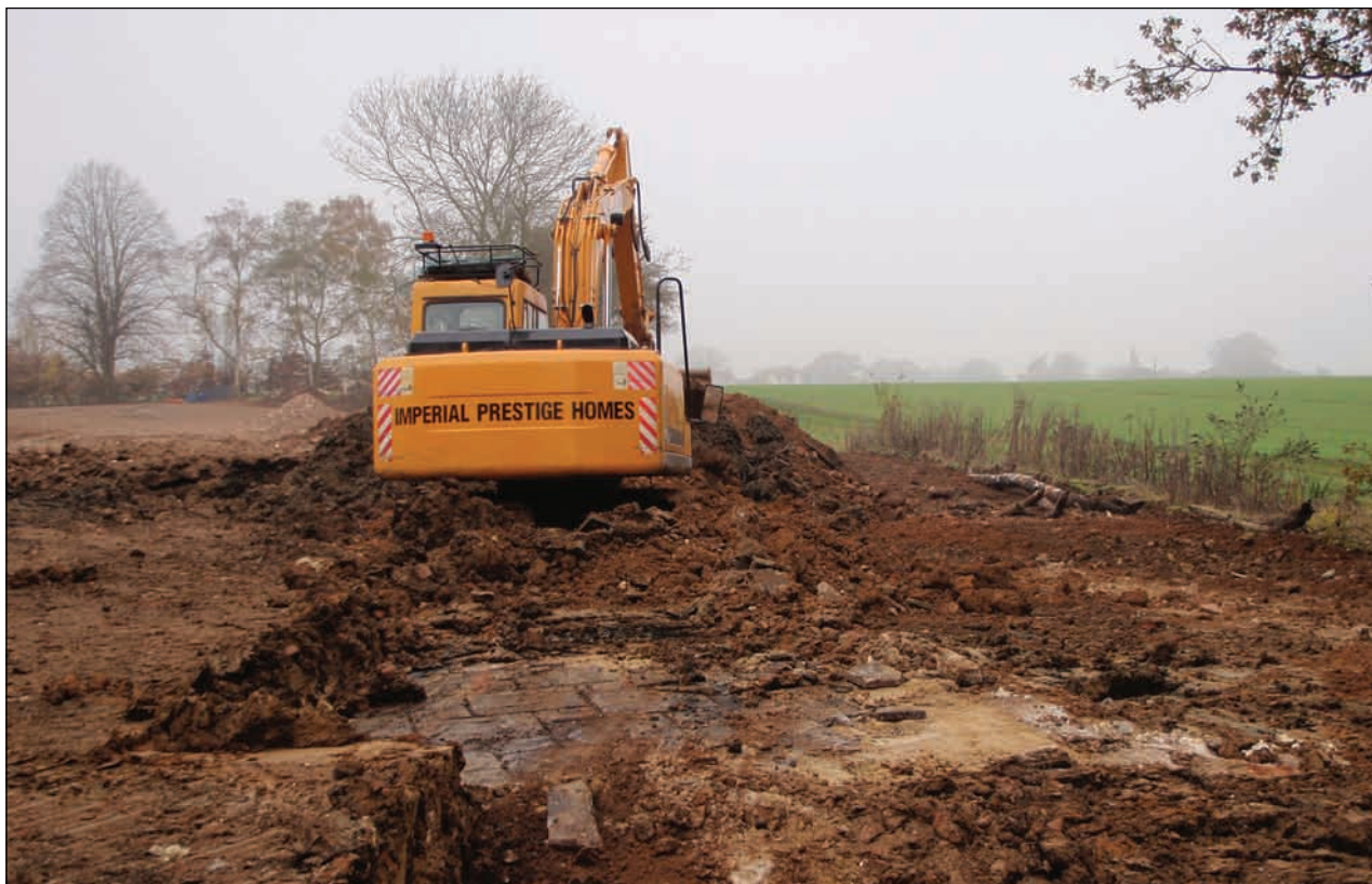
Plate 3: Removal of dumped material over the swimming pool. View from the east.
