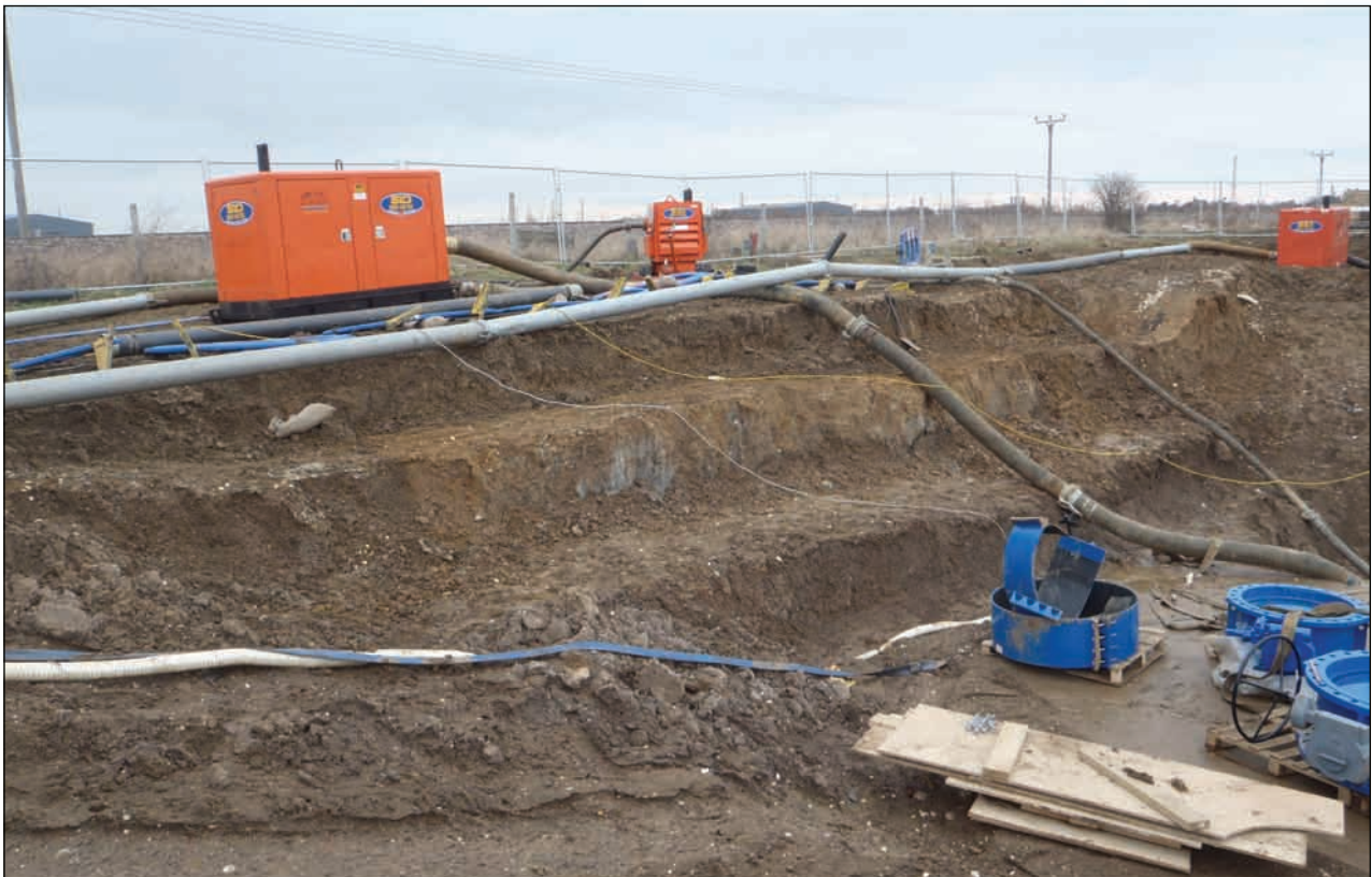
Plate 2: Large scale excavation was required to access the water main
