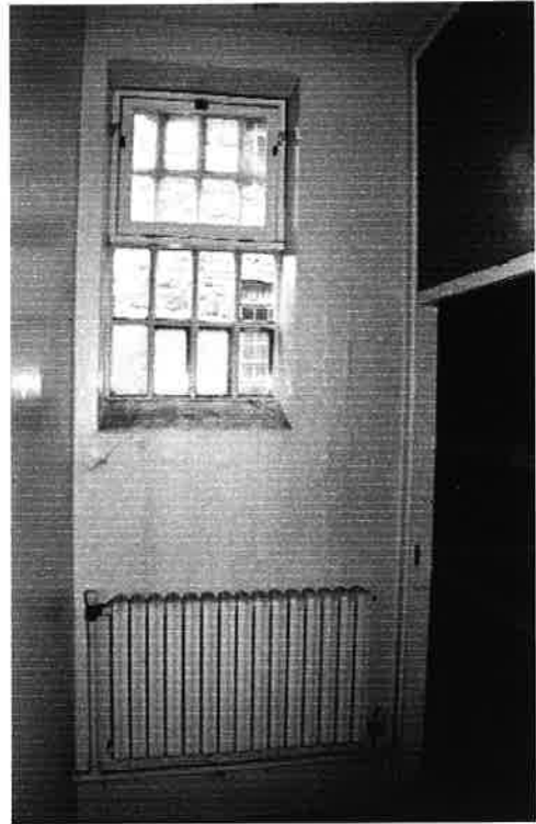
Plate 22: Window within secure unit
