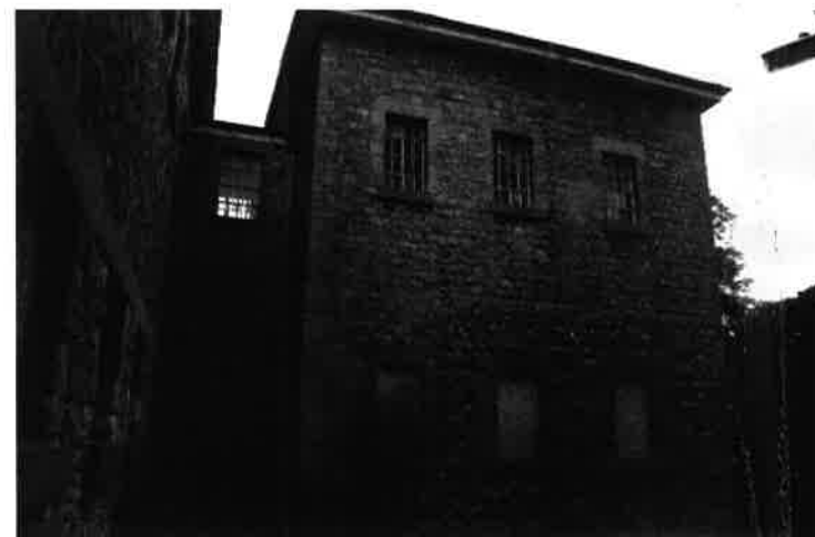
Plate 14: Extension to west of south wing
