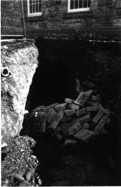
Plate 32: Cold air channel exiting south Wing during infilling
