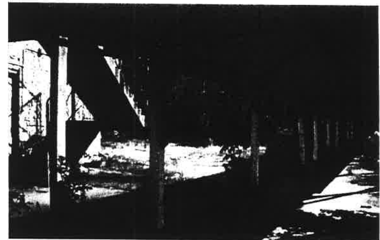
Plate 39: Walkway viewed from north
