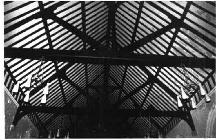
Plate 41: Church roof from west
