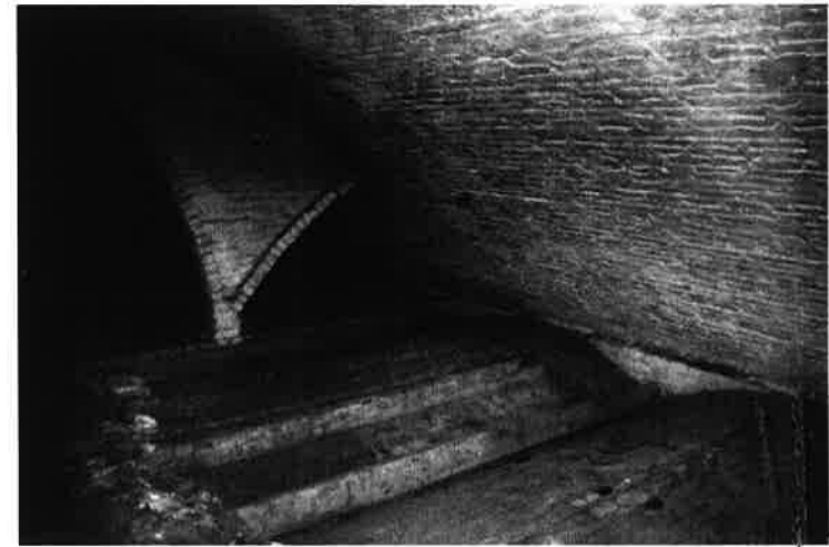
Plate 10: Brick ceiling arches from above
