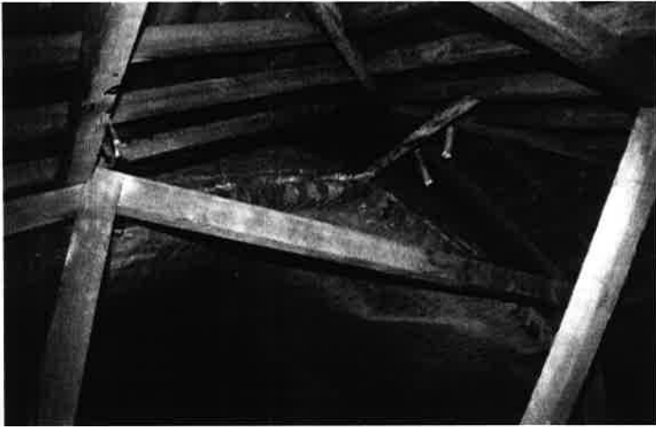
Plate 9: Junction between brick vaulted roof and central section
