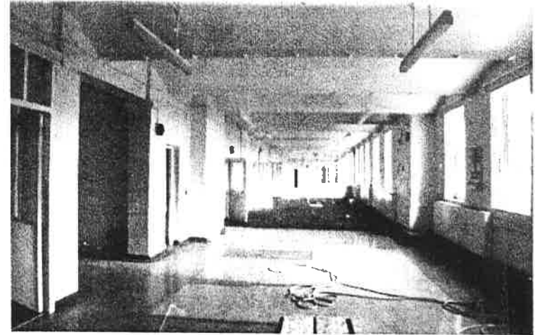
Plate 2: Gallery (F1) from south
