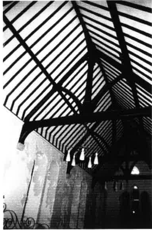
Plate 45: Roof of later aisle
