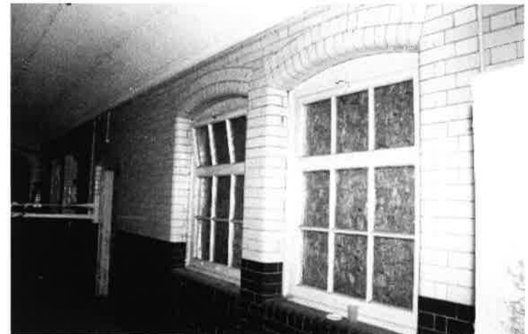
Plate 27: Corridor added to north in 1904
