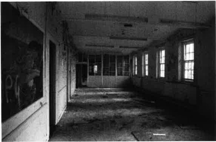
Plate 17: General view of F41 from south
