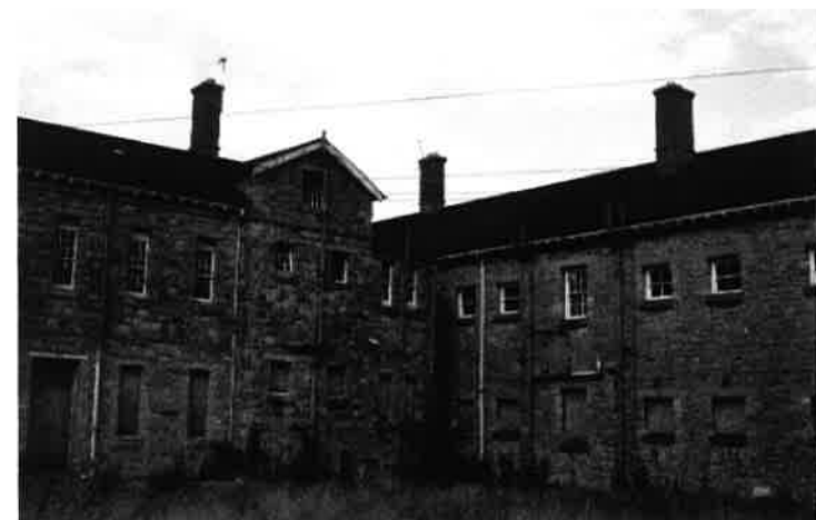
Plate 16: Junction between main north wing and central projection
