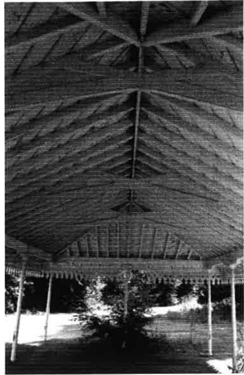
Plate 33: Inside of north pavilion
