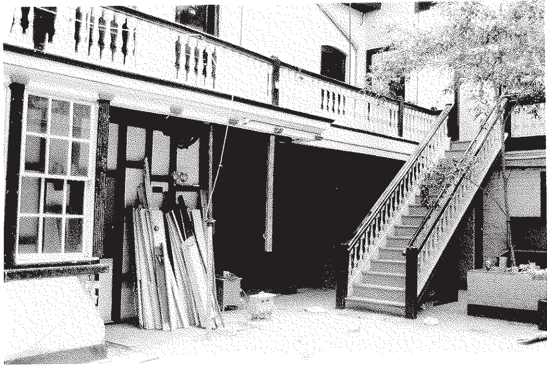
Plate 13: Stair in south-east corner of courtyard removed during refurbishment
