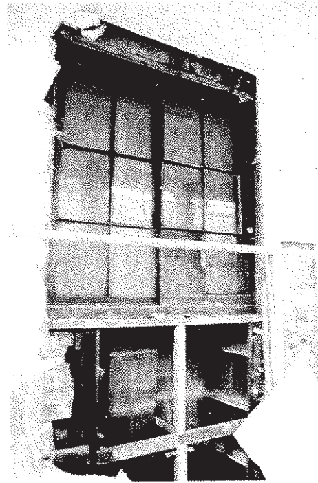
Plate 10: Horizontal sliding sash, 'Back bar'
