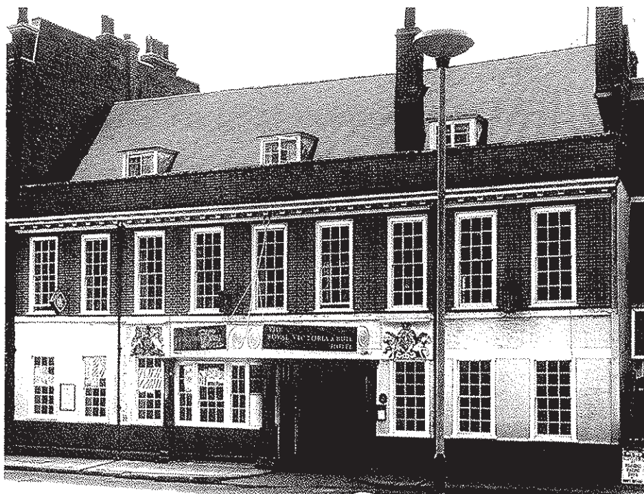
Plate 3: Front elevation, before refurbishment (RCHME, Swindon)
