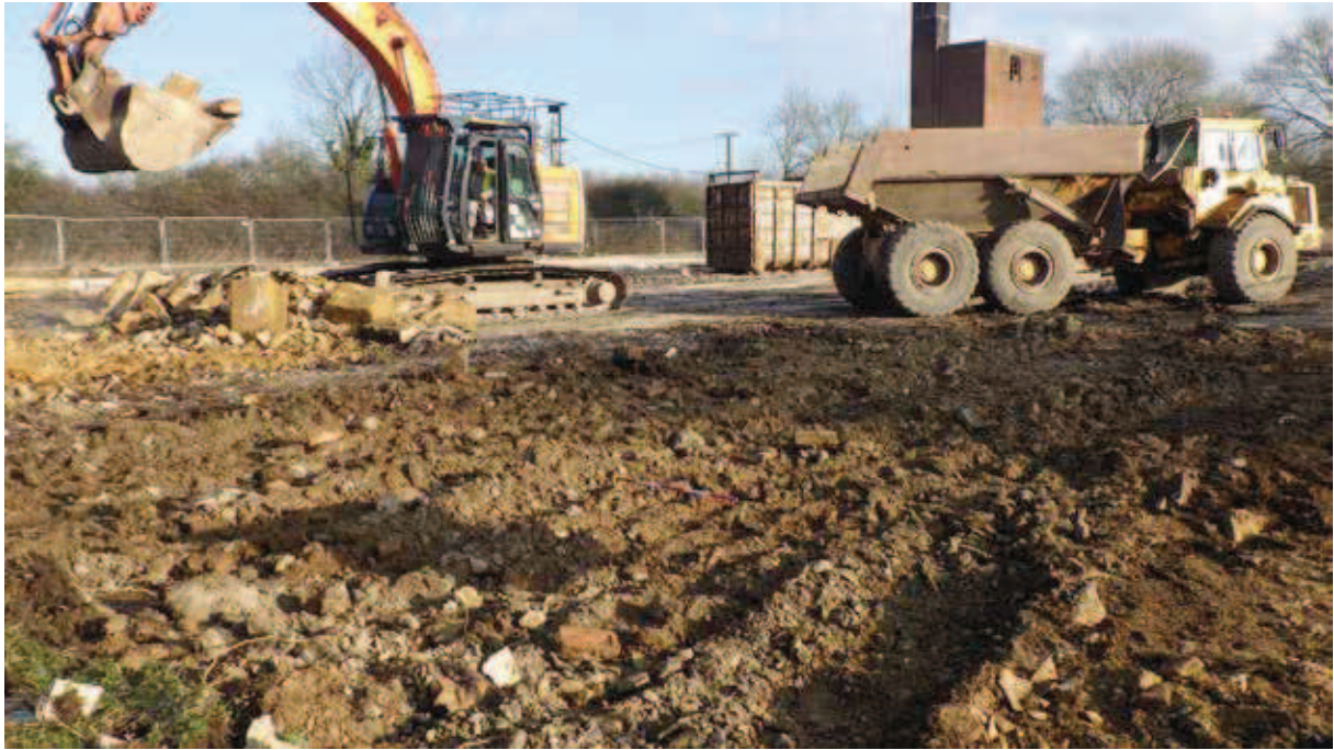
Plate 2: Rodney House concrete slab removal showing underlying hard core rubble and the limitation of plant to existing hard standing areas. View north
