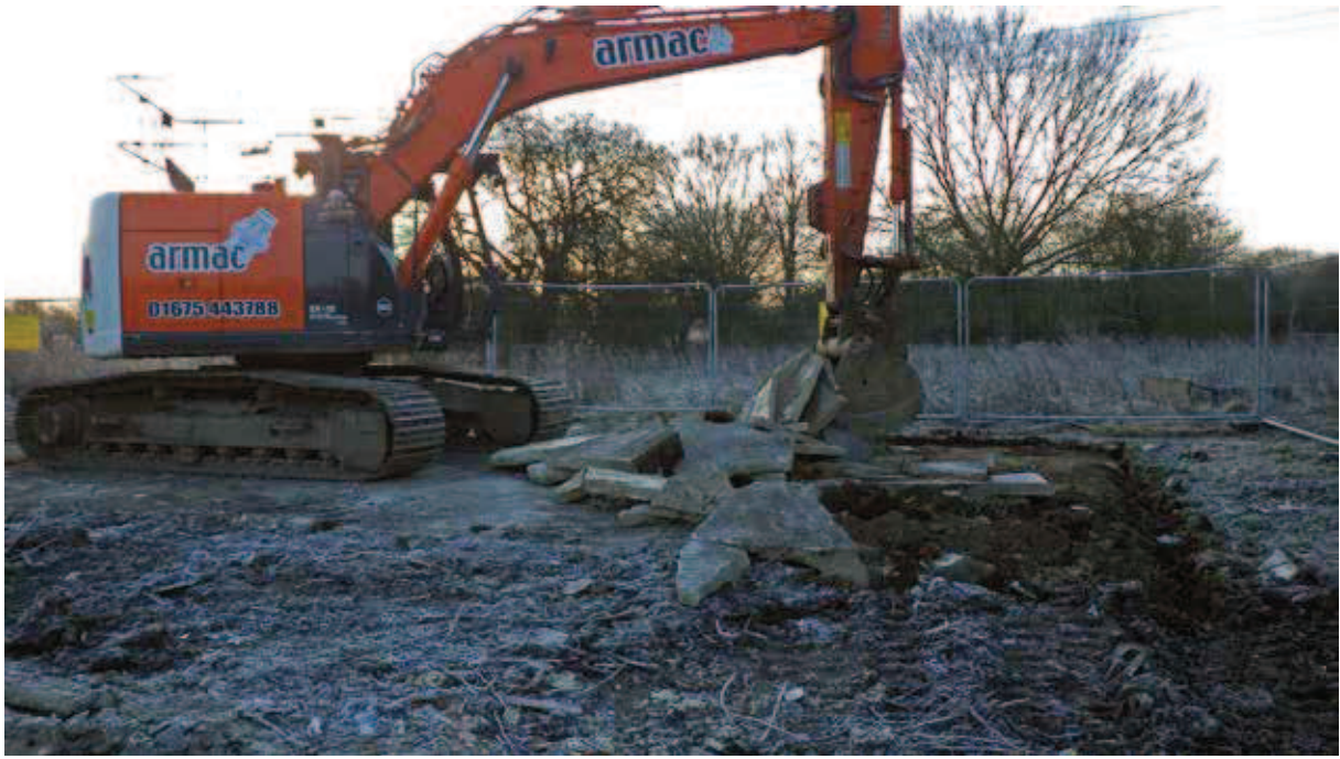
Plate 1: Rodney House concrete slab removal
