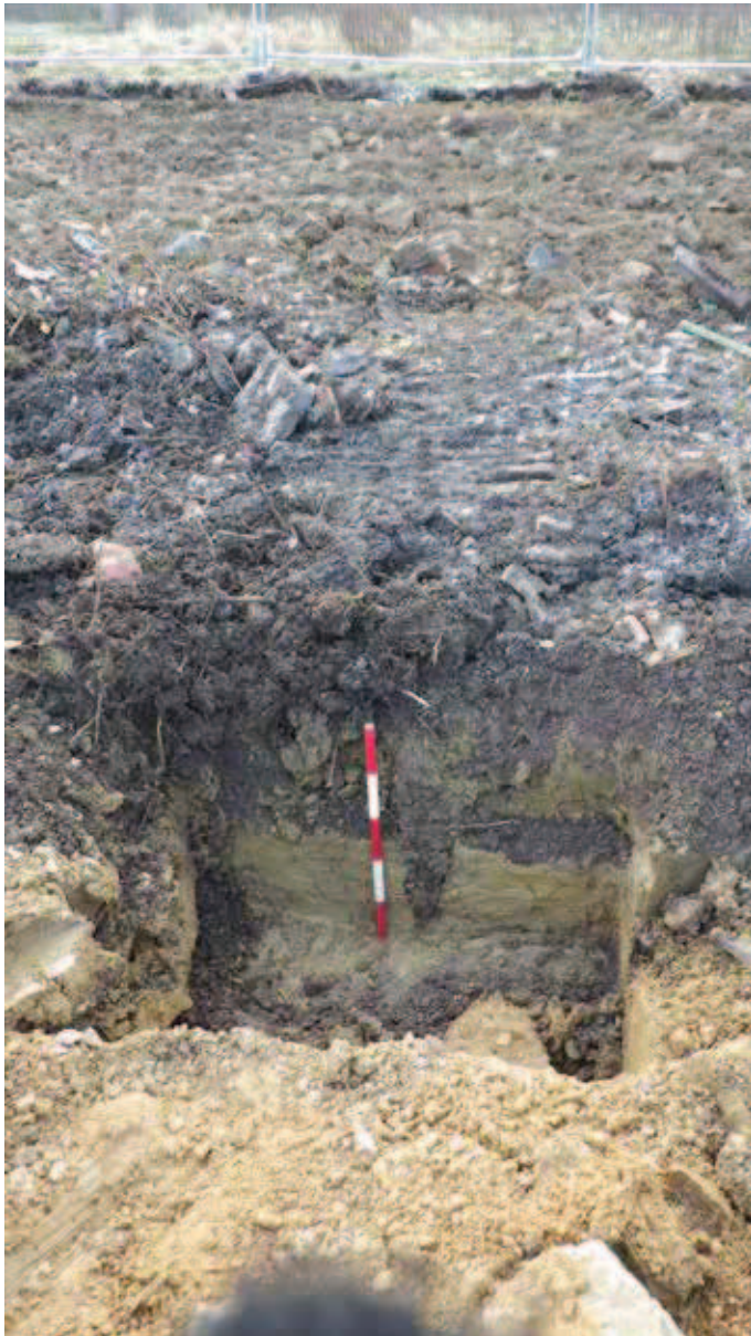
Plate 4: Foundation pad removed showing the exposed level of natural clay and the hard core rubble laid directly over this
