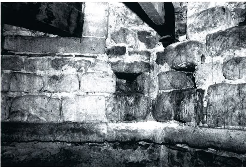
Figure 36: South-east corner turret: projecting stone string course below current roof level denotes former roof line; note ceiling joist (left) housed within splay of former loop.
