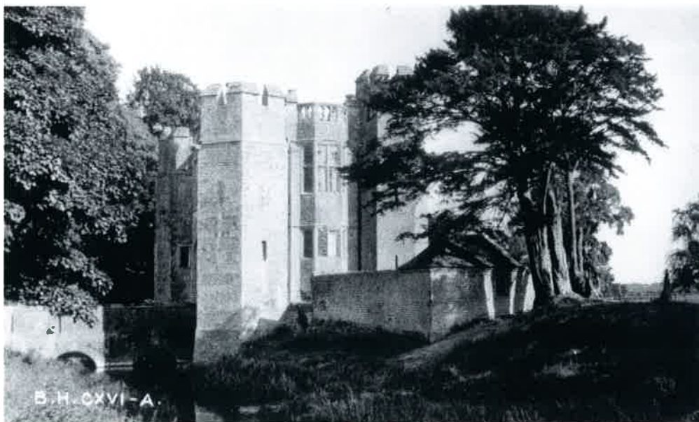
Figure 10: north-east elevation, photographed in 1911
