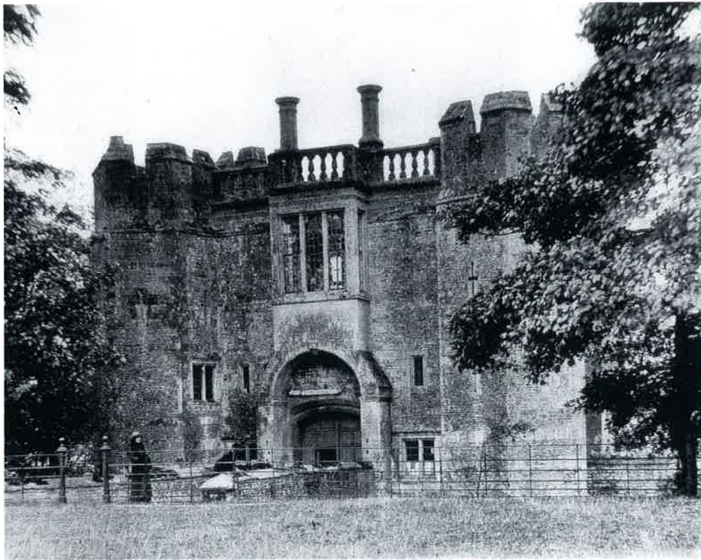
Figure 9: North-west elevation, photographed in 1911
