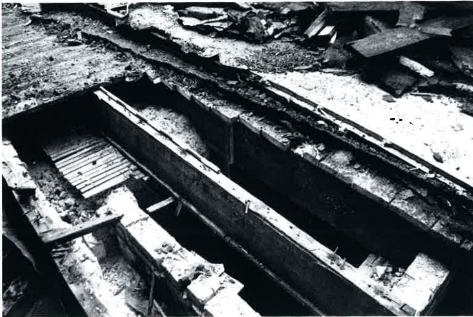
Figure 27: annexe roof during dismantling showing successive layers of boards and roofing felt
