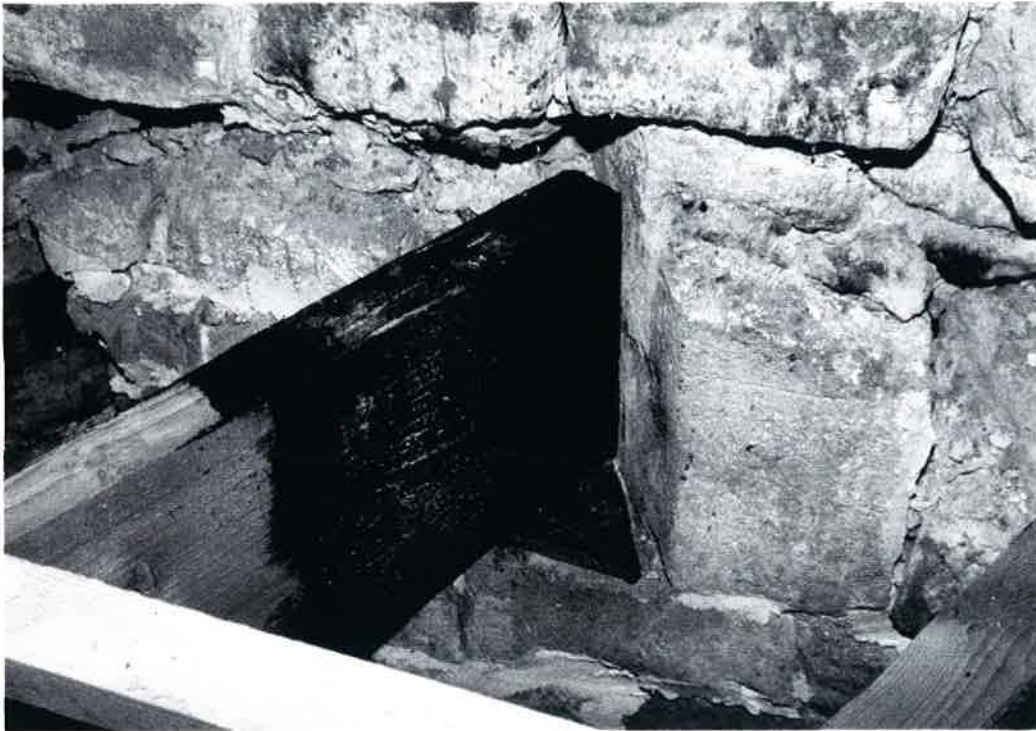
Figure 35: Ceiling joist of south-east corner turret housed within splay of former loop.
