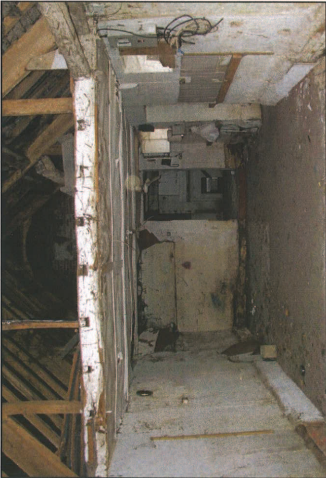
Plate 17: Interior of Block B looking south
