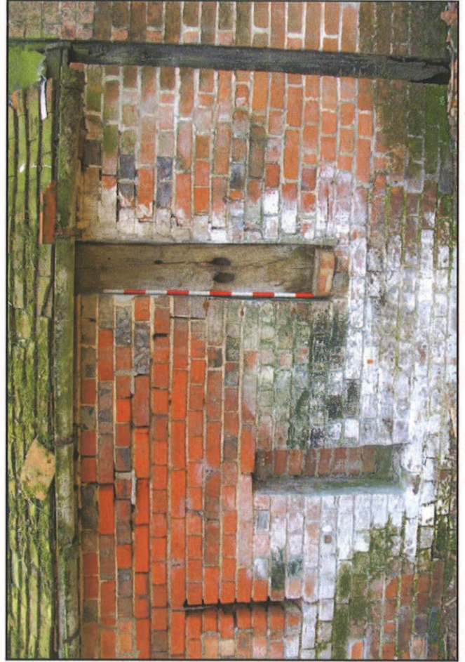
Plate 4: Former openings for machinery belt drive in north wall of barn
