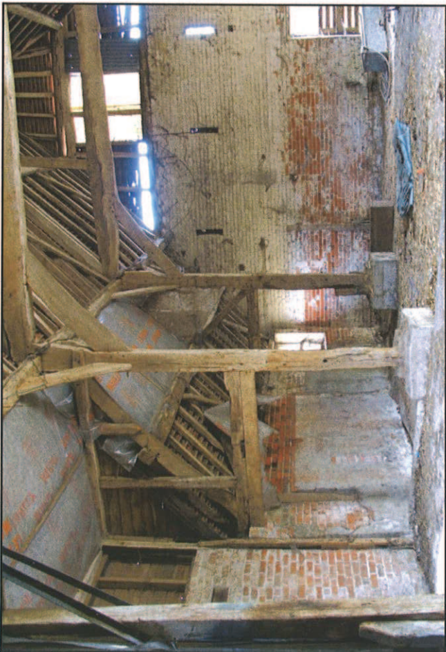
Plate 9: Part of interior of barn looking north-east
