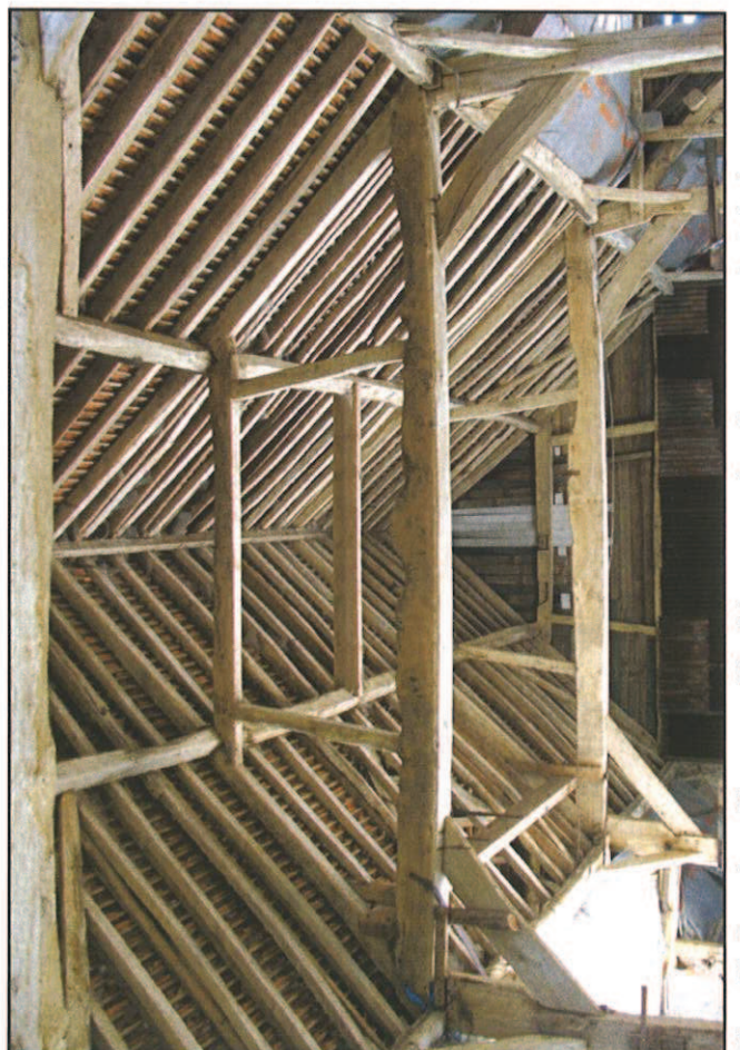
Plate 11: Interior of barn roof looking west showing trusses 2, 3 & 4
