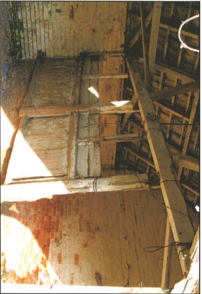
Plate 21: Timber partition within shelter shed, looking north-east
