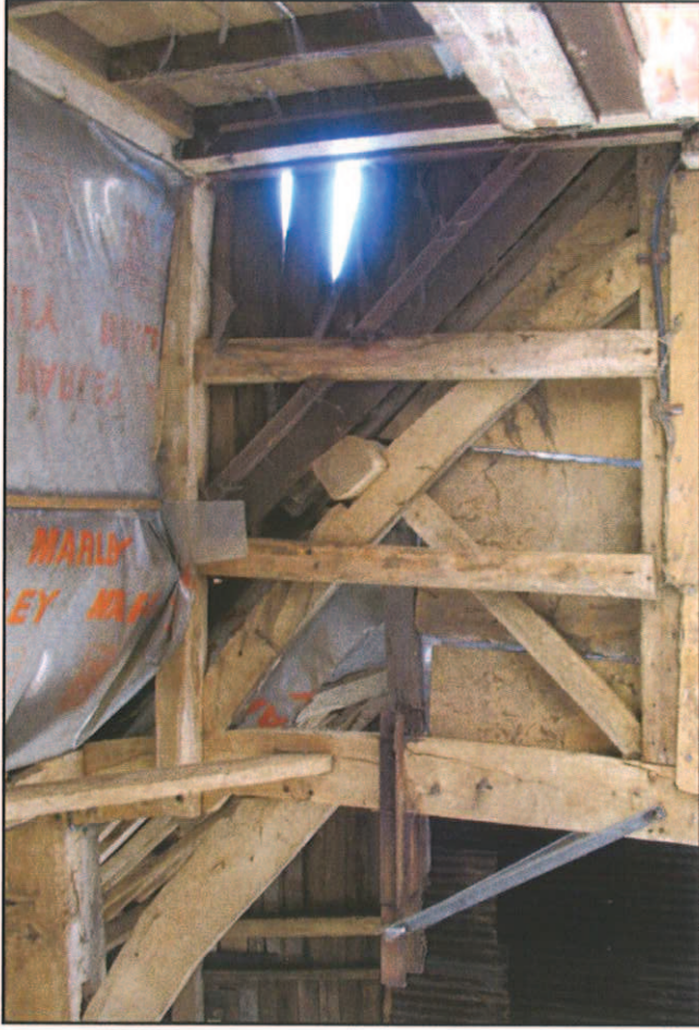
Plate 14: North side of truss 3 showing addition of later porch timbers, looking west
