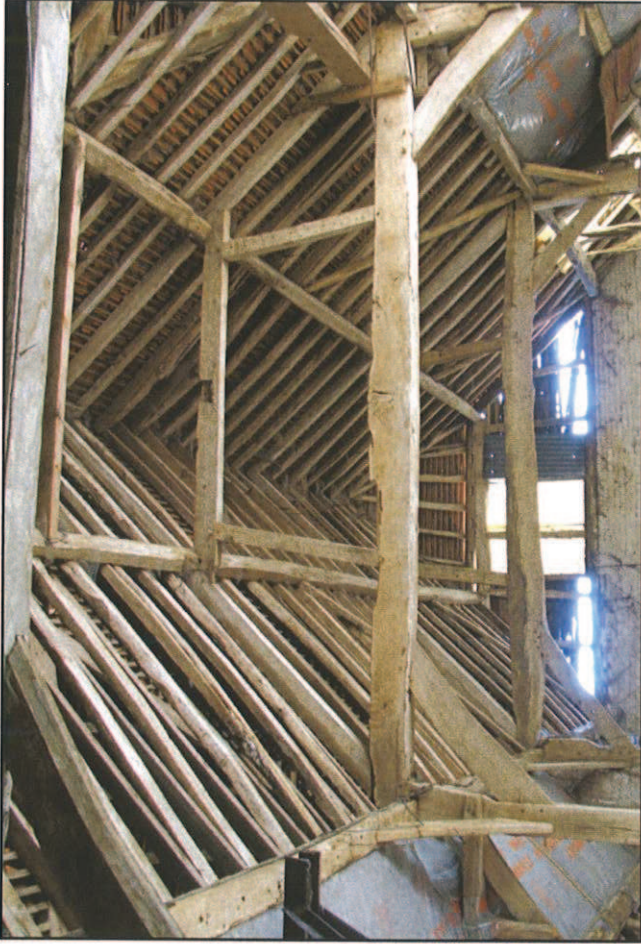
Plate 10: Interior of barn roof looking east showing trusses 1 & 2
