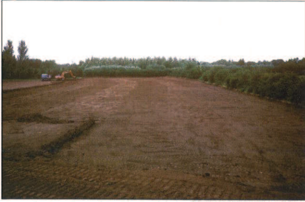
Plate 1: Stripping of site
