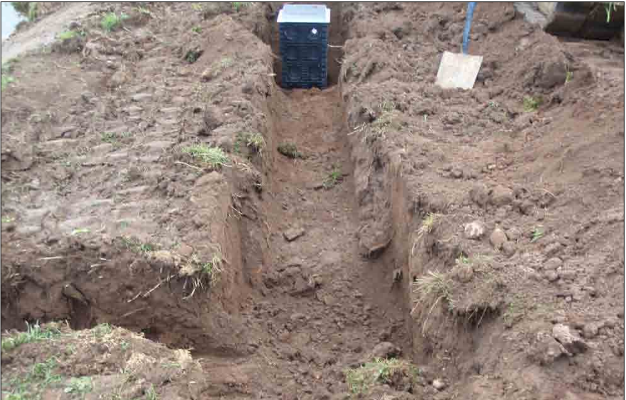
Plate 4: Embankment groundworks, taken from north-east.
