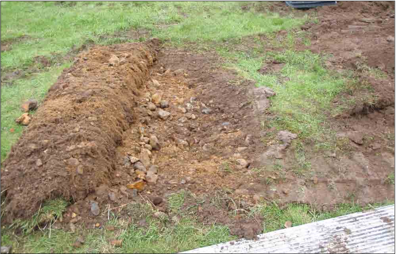
Plate 3: Turf removed by machine bulldozer blade, taken from south-west.
