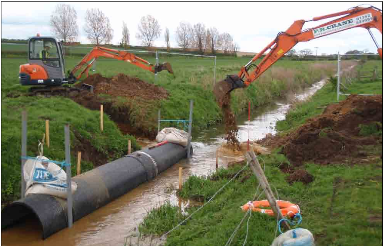
Plate 1 : Excavation of the trench through the river, taken from south-west.
