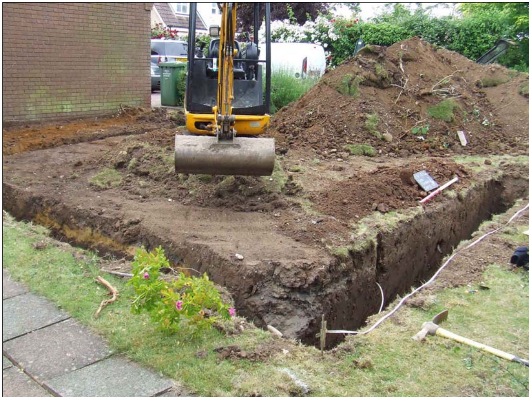
Plate 1: Site Overview from North East
