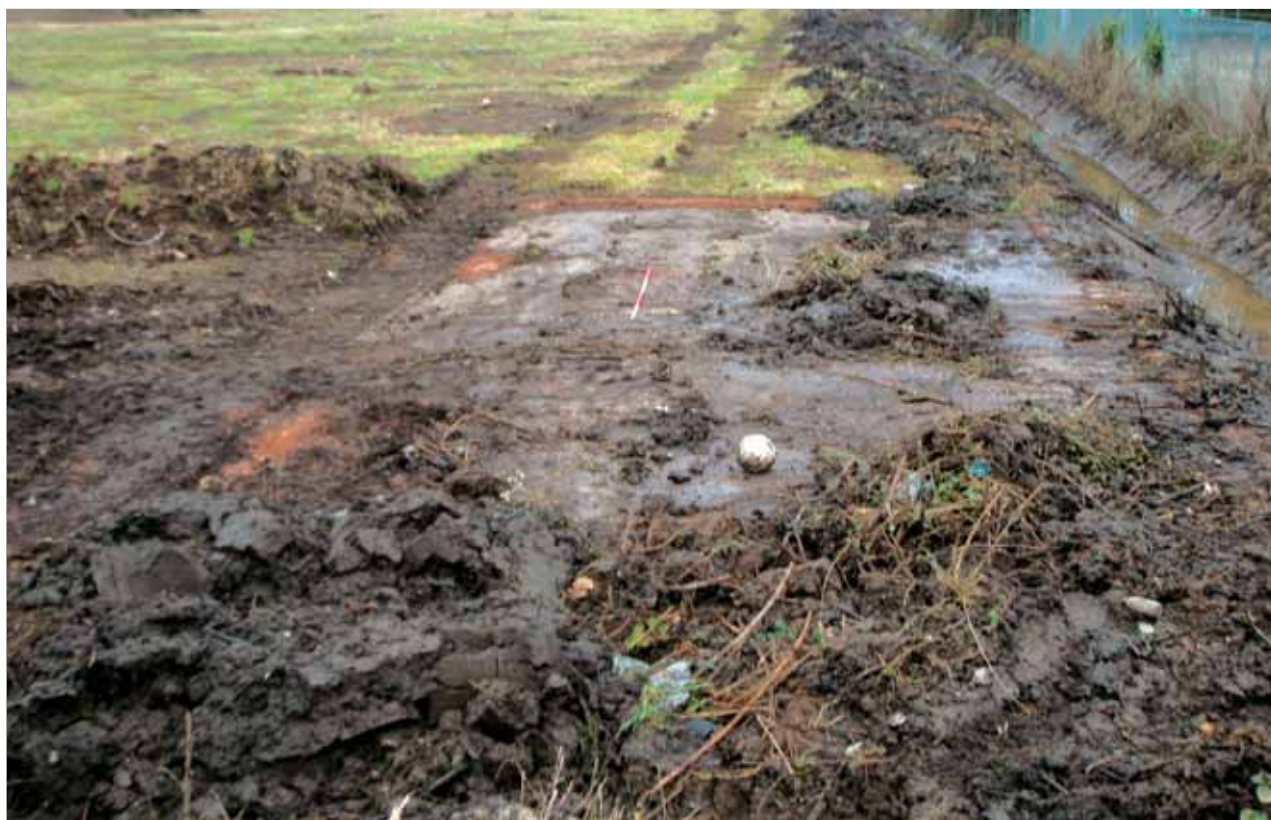
Plate 6: Exposed concrete pad in area E
