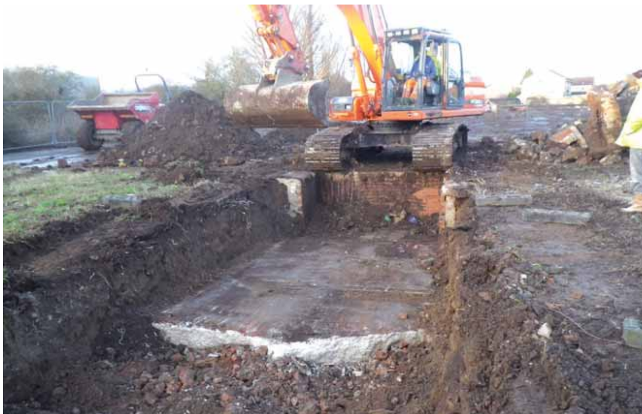
Plate 5: Possible vehicle access to south end of area D
