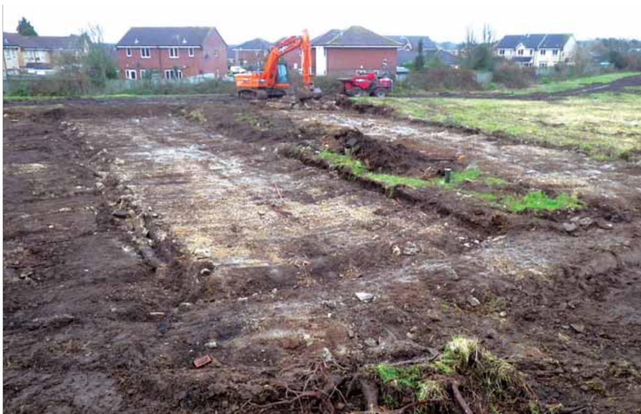
Plate 1: Concrete removed from bays 1, 2 and 4 in area C
