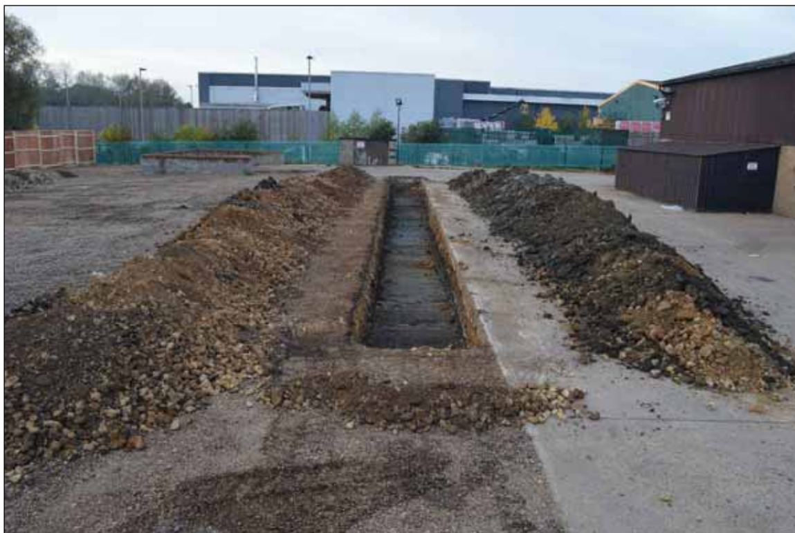
Plate 5: Trench 8, looking south-east
