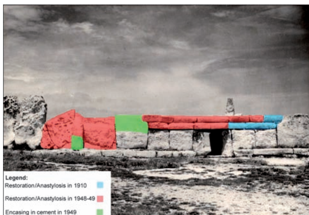
Figure 4 Ħaġar Qim: Restoration of the façade, interventions of 1910 and 1949–50.
