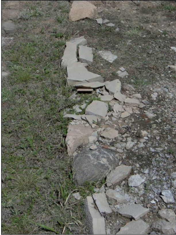
Figure 3 The outer kerb of Mound 4 at Location 2. This type of stone, perhaps micaeous, is particularly susceptible to freeze/thaw cycles, and has deteriorated very rapidly since exposure.
